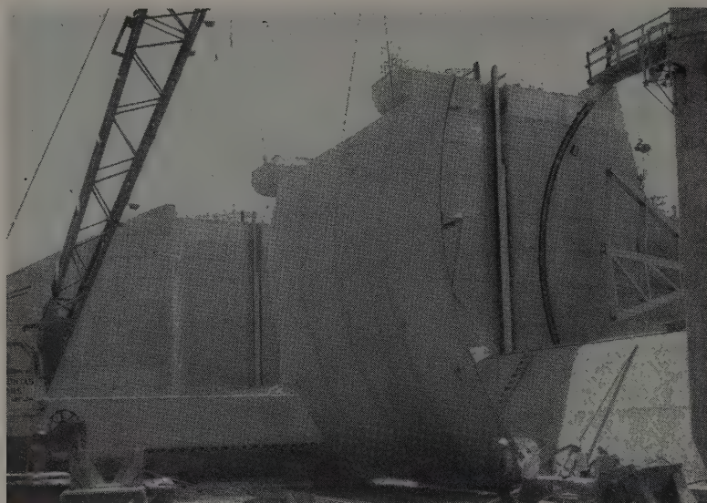
GATE LEAF at Dexter Dam is hoisted to vertical position. Arms are in place.
