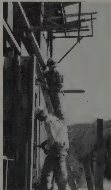
FORM TIES are being installed in concrete formwork for the exterior wall of the west side of the powerhouse. Large window openings on this side will be glass block.
