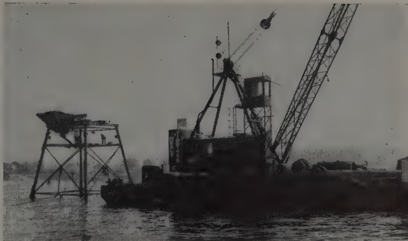
IMPORTANT FEATURE of tower is attached hopper. Gravel placed in hopper by derrick is chuted to bottom. Diver directs flow to embed the pipe. Intrusion Prepackt method will be used.
