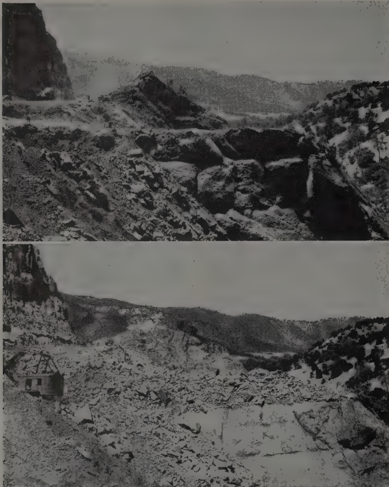
PHOTO PROFILES of rock knob above spillway site on right abutment show results obtained with a computed powder factor of 2/3 lb. per cu. yd. Breakage was good and the Northwest moved right in to clean things up for a final trimming shot.
