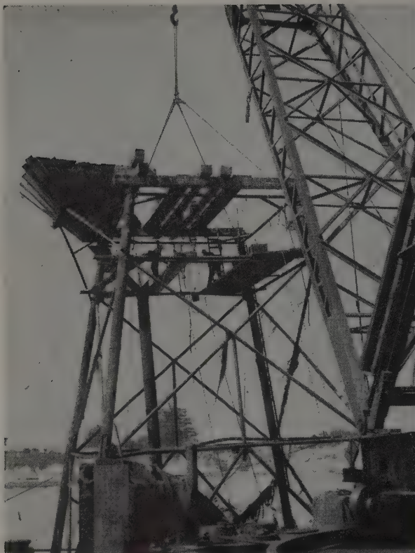
LIFTING the 22-ton tower to position over a newly laid section of pipe requires but a few minutes for the derrick. Tower is 60 ft. tall and will handle laying problems out to 40-ft. depth.
