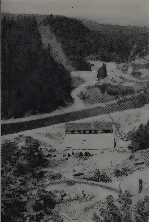
LOOKING FROM surge chamber location shows stockpile of timbers for tunnel support and tracks of mine cars (lower). Northwest crane to right of powerhouse is placing concrete in west wall. Natural river bend to the right of the picture will be lowered and straightened by tailrace channel excavation.
