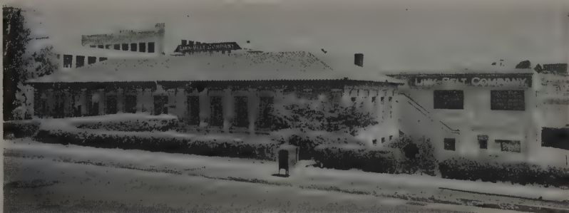
LINK-BELT CO. has completed a 3-story addition (above) to its San Francisco plant to allow for increased manufacturing, engineering, and warehousing facilities and a factory branch store. The company has also started work on a new district sales office and warehouse building in Portland.
