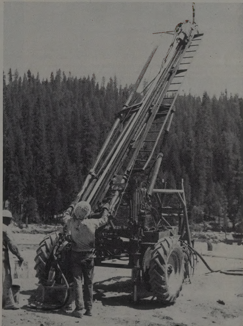
SETTING UP the Joy Challenger drill takes but a few seconds. The 30-ft. long mast is shown here in the process of being raised to a vertical drilling position. Leveling the 9,000-lb. weight of the frame is handled by three hydraulic jacks—located near each wheel.
