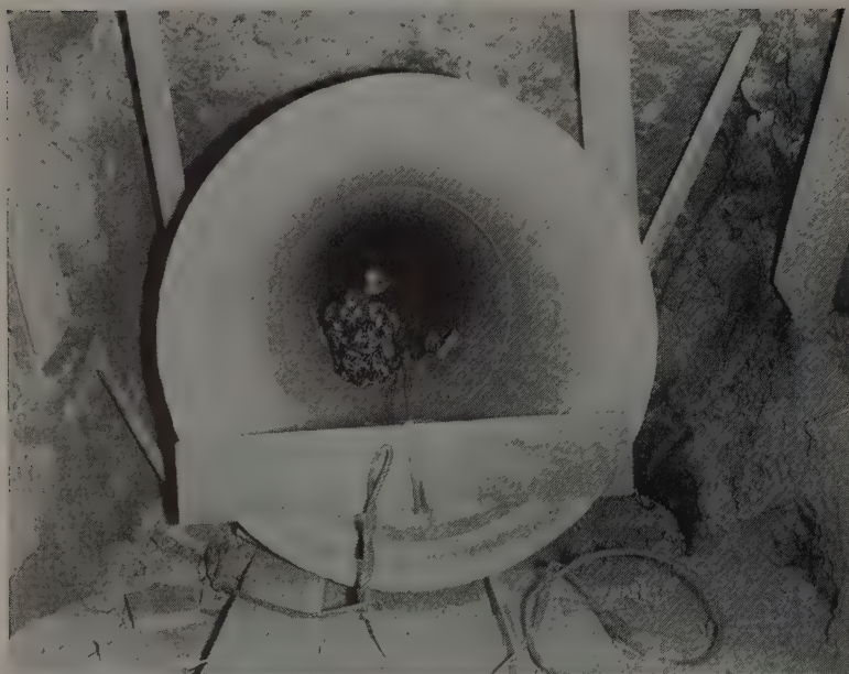
VERY LITTLE ASSISTANCE was required from a come-along to move five sections of pipe down the 30-deg. slope. The pipe rested on a concrete cradle in the pilot tunnel. Excess dirt is cleared away in front. (Photo courtesy of United Concrete Pipe Corp.)
