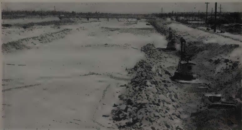
Looking upstream along the Lower Los Angeles River. Channel and levee improvement operations on left bank. Toe trench is being excavated to receive toe rock, shown stockpiled in foreground of picture.
