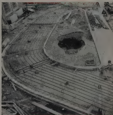
SNOW MELTING, RADIANT HEATING
