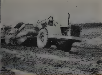
QUICKSAND! D8 push-loads DW21 and No. 21 Scraper in quicksand over blue shale for Ralph Myers Contracting Corp. (Salem, Ind.).
