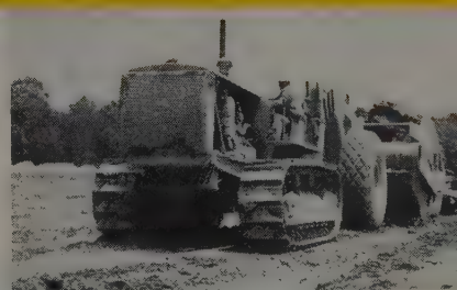
GUMBO! No. 90 Scraper, pulled and push-loaded by D8s, works in gumbo for Harrison Construction Co. (Pittsburgh).
