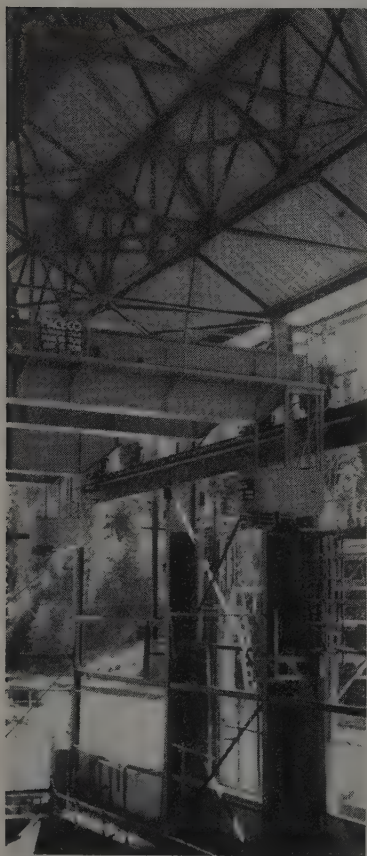
ABOVE THE PIT, two 115-ton capacity cranes are in use for setting heavy parts. Walls to the right are being formed around glass block window openings. Roof is composed of laminated 2x4's on edge.
