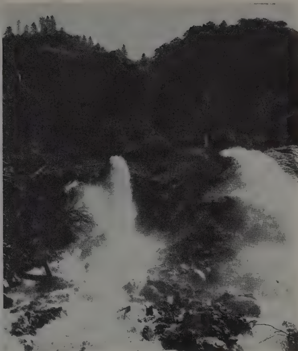
TUNNELING CONDITIONS can best be described by looking at this 16,000-gpm. discharge coming from the outlet portal. An additional 4,200 gpm. is being pumped from the upstream adit. To concrete line the tunnel, "panning" will be necessary first, this to be followed by grouting behind the walls.
