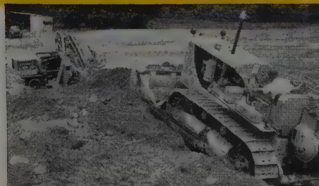
CRUSHING! D8 loads portable gravel plant powered by D337 for W. J. Menefee Construction Co. (Sedalia, Mo.).
