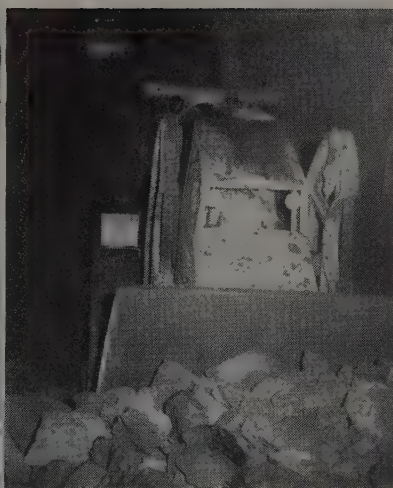
NEW EIMCO makes quick work of muck, but small body size of Dumptor requires mucking in low gear. Otherwise, Eimco could nearly throw muck clear to the portal!
