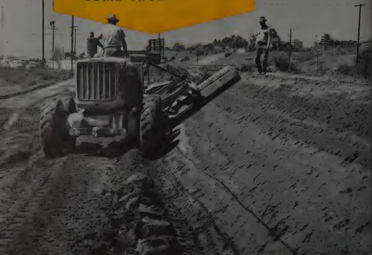
This No. 12 Motor Grader, owned by Daley Corp., is bank-sloping for a canal along the new Wabash Freeway, San Diego, Cal.
