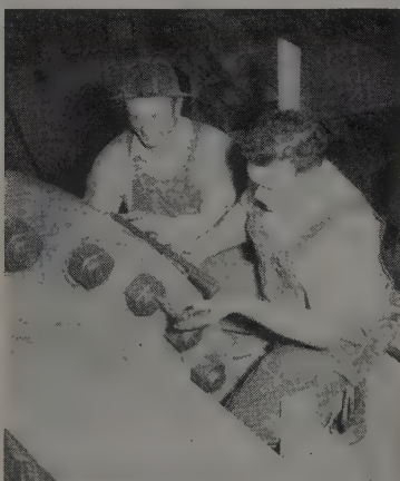
BOLTS CONNECTING flanges of the spiral case and the relief valve are tensioned to 23,000 lb. Tension is determined by micrometer measurement of bolt elongation, which is only 0.009 in. in this case for full stress.
