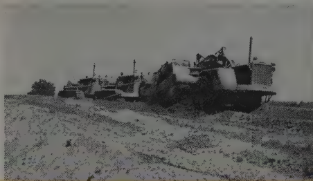
ROCK! D8s in tandem push-load DW21 and No. 21 Scraper in rocky soil for R. B. Potashnick (Cape Girardeau, Mo.).
