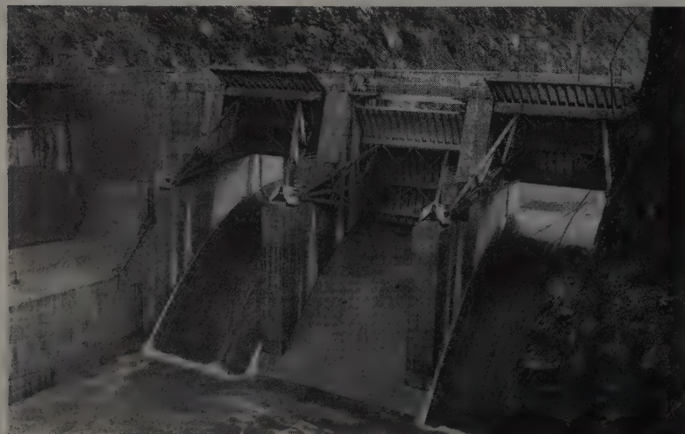
... HERE they are open, with water pouring over spillway in a test operation.
