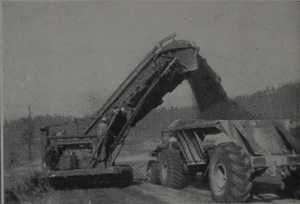
DAYTIME OPERATIONS utilize this Euclid elevating loader to load bottom dump wagons. One pass of the loader takes an 18-in. lift. Also being used are Cat DW20's with D8 pushers.
