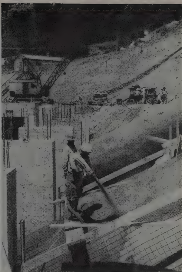
GUNITE COVER of 1-in. thickness over the two 12-ft. diameter penstocks is required where they pass under the future transformer area. Penstock is first treated with hot coal tar and then covered with 4x4-in. wire mesh reinforcement for the gunite. Penstocks are 830 ft. long for 382-ft. fall.
