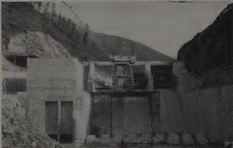
WHIRLEY CRANE on a steel trestle erects gate parts at Big Cliff Dam . . .
