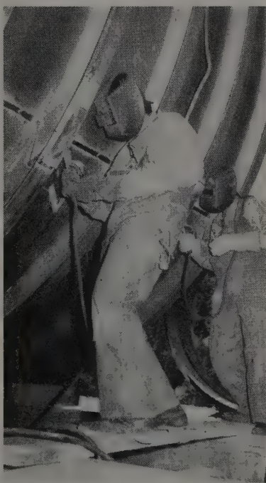
BETWEEN the surge chamber and the outlet portal, 300 ft. of steel liner will be installed. The liner arrives in quarter-circle segments shown here being welded together.
