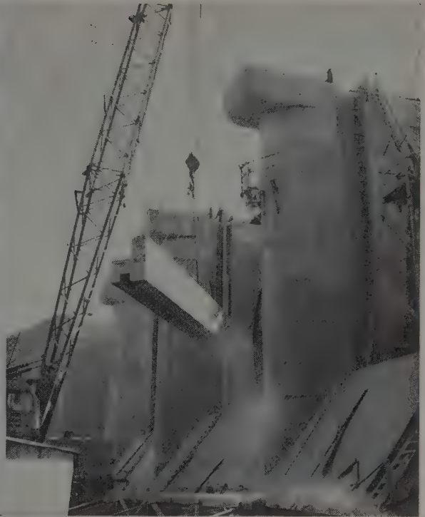
MANITOWOC CRANE with 120-ft. boom has good control (above and below) in two steps of handling a 60-ton bridge girder.
