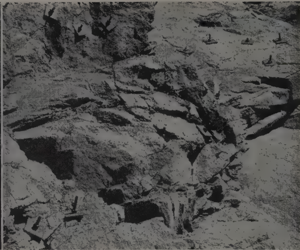
RAILROAD CUT in Montana uses bolts to stabilize massive, non-stratified rock which breaks into big, irregular slabs. Bolts stabilize toe, which in turn supports rest of cut bank.
