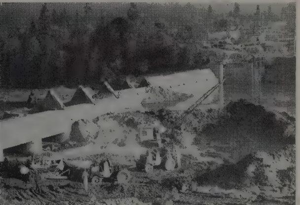
OCTOBER 15, 1953 —Cofferdam No. 3 removal with completion of work on south half of dam. River flow is through sluiceways under pumphouse at right center. Note new river outlets under dam at left.
