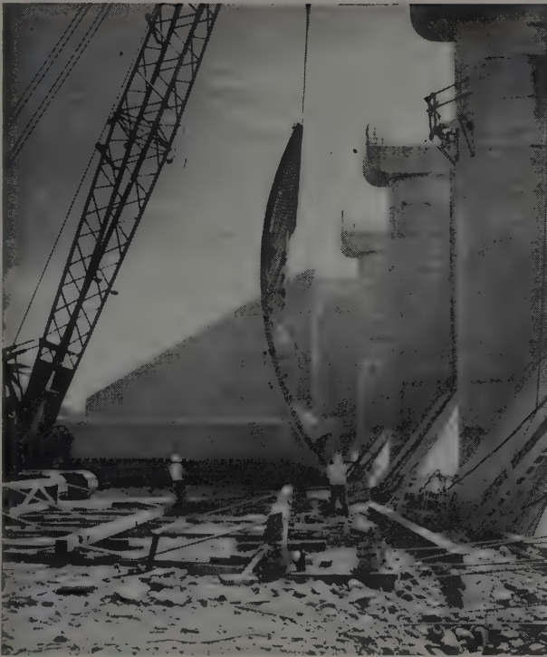
TAINTER GATE , all 44-tons of it, is shown being lifted shortly after taking it from the assembly cradle in the foreground.
