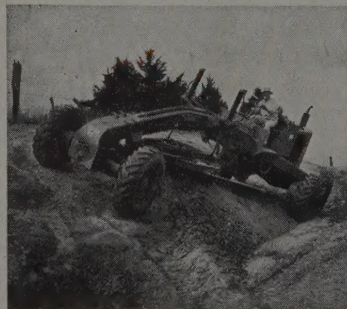
8 Live power in front drivers makes it easy to ride steep banks, when finishing.
