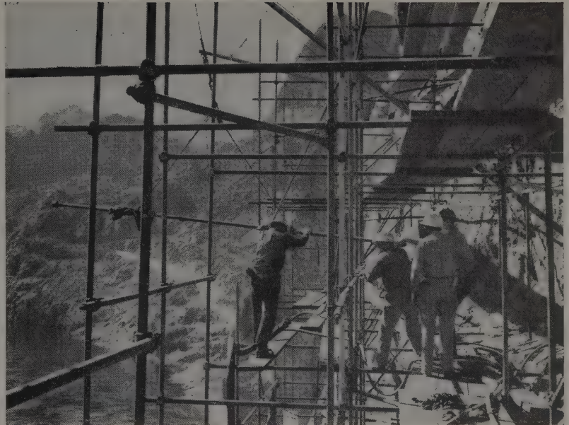
ANCHOR BARS at Hoover Dam are king-size—2 in. in diameter and up to 30 ft. long. Driven on 7½-ft. centers and tensioned to 63,000 lb., they anchor a rock slab on the canyon wall above Nevada valve house. Slab is about 120 ft. high, 180 ft. long, and up to 19 ft. thick. After pinning, rock was pressure grouted as an added safety measure.
