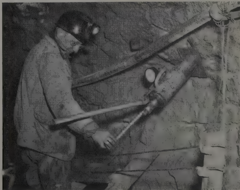
PULL-OUT TEST in Duchesne Tunnel uses 50-ton jack. Pulls up to 10 tons were applied with no slippage. Bureau of Mines furnishes men and equipment for tests on request.
