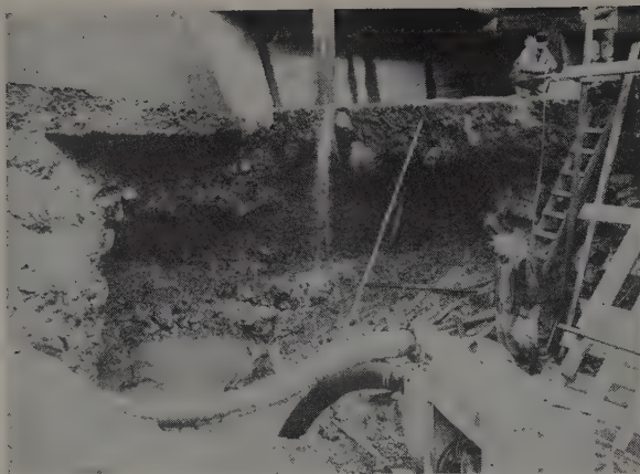
NOVEMBER 15, 1953 —Downstream cofferdam for the north half of the dam has been completed to allow repair work on the badly eroded sluiceway and tailrace wing wall. Hole is 20 ft. deep.
