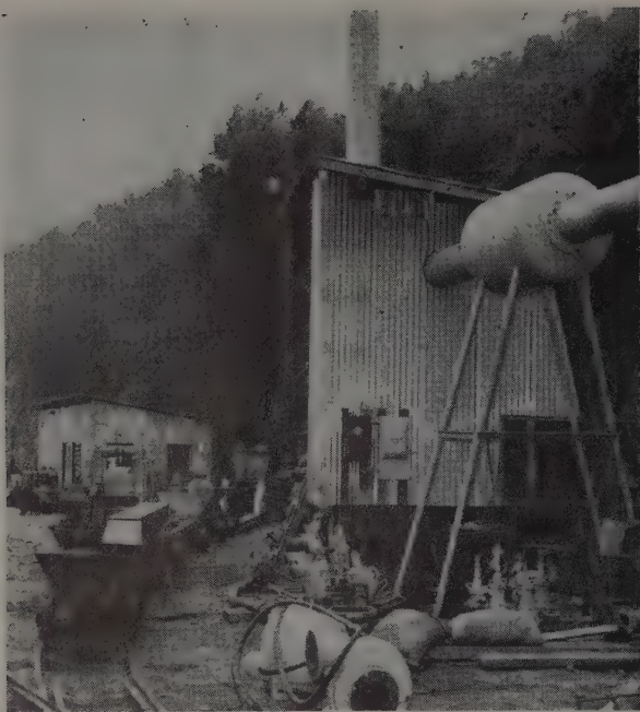
AIR is vital, especially on this job, where 5,000-cfm. Sutorbilt blower figuratively (and in this picture) overshadows other machinery, including train of mucking equipment.
