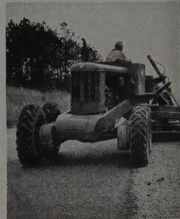
6 No tire marks on this shoulder, thanks to rear steer.
