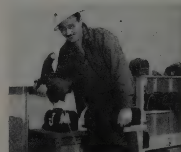
BILL ROBERTS , shift walker and another of the Eklutna gang, shows how easy it is to pour water from a boot! Like the others, he hopes it won't be necessary to do much more grouting. It takes time, and "it seems like you're just pushing the water ahead of you instead of getting rid of it."
