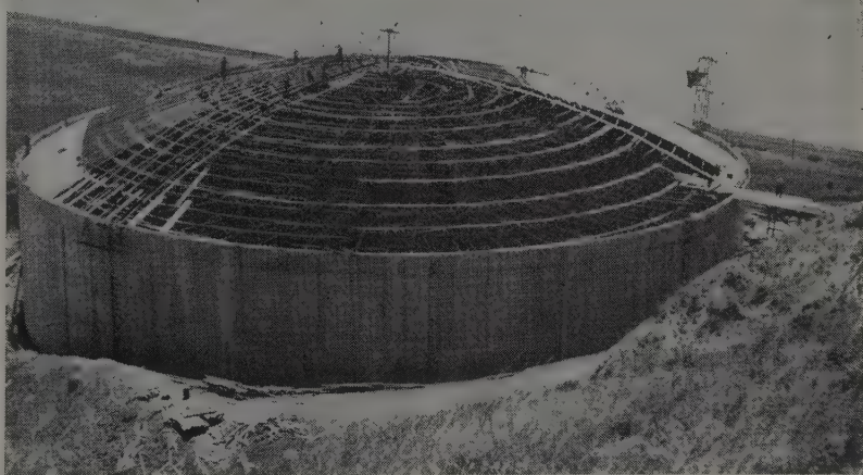
WALLS have been poured with embedded horizontal and vertical cables but not yet stressed. Dome framing is placed at proper elevation by measuring down from pipe frame template.
