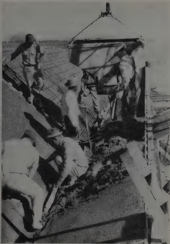
VIBRATING 2-in. slump concrete out of the bucket was required. This enabled concrete to remain on steep slopes.
