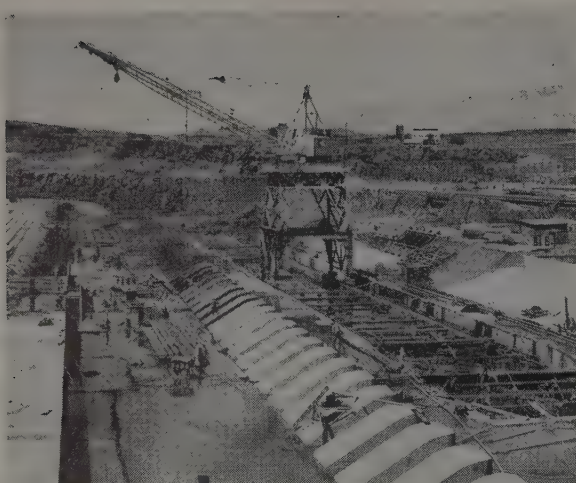
ABOVE—Concreting operations are well under way on the stilling basin of the spillway. Two Clyde whirleys handle all materials.
