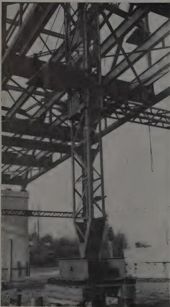
BELOW —Falsework tower rests on four capped piling. Double pin connection at bottom allows complete freedom for alignment.
