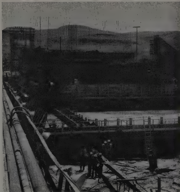
ABOVE—Concreting operations are well under way on the stilling basin of the spillway. Two Clyde whirleys handle all materials.
