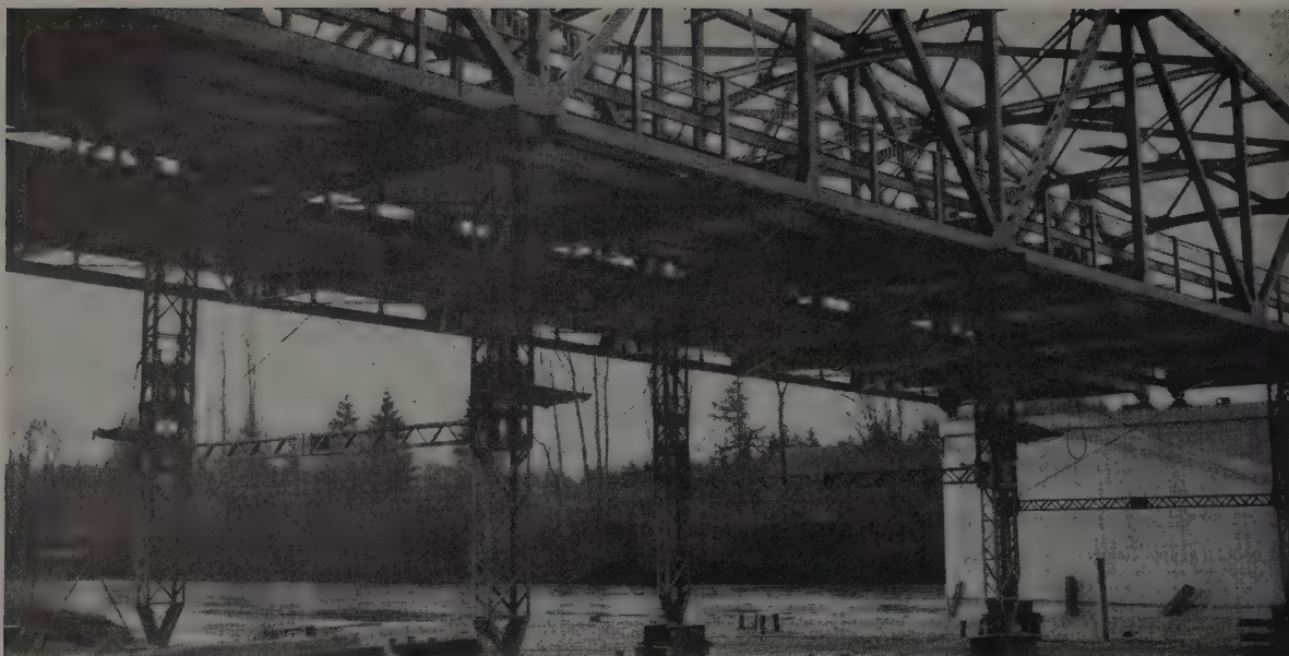
BELOW —Falsework tower rests on four capped piling. Double pin connection at bottom allows complete freedom for alignment.
