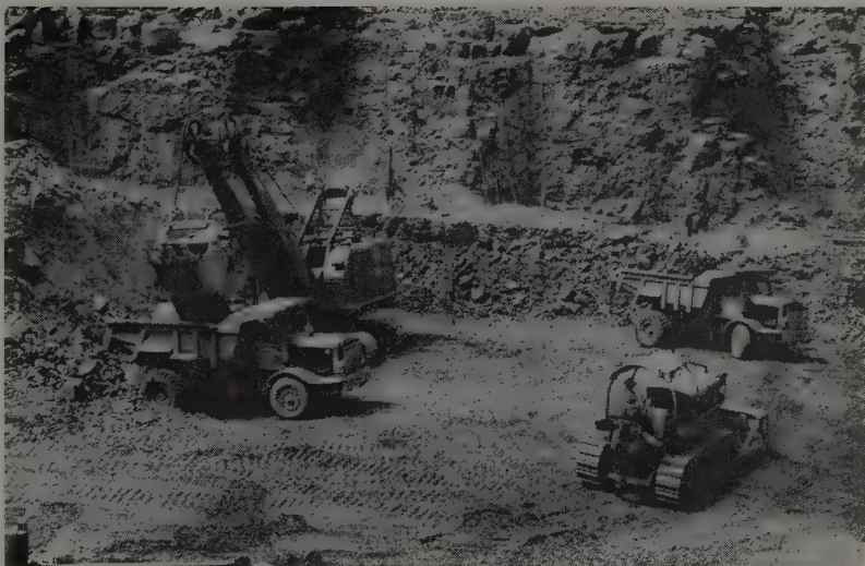
ABOVE—A Bucyrus Erie shovel, with 4-yd. dipper, has loaded up to 250 Euclid 16-cu. yd. truck-loads in one 8-hr. shift, while Cat D8 bulldozer keeps working area level. BELOW—Same area, drilling and shooting to 18-ft. depth is well ahead of excavation.
