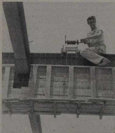
BELOW LEFT —Rod clincher clamps rods to steel beam.
