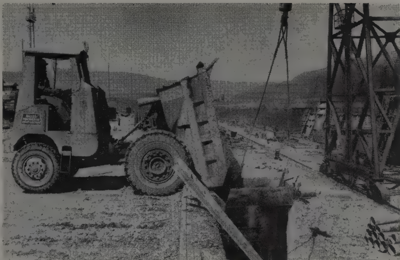
JOB-MODIFIED Koehring Dumptors, 4-cu. yd.-capacity, have quick dumping action. This method of transporting concrete is a first for any Corps of Engineers project. Dumptors normally haul rock, but eight of them are used to deliver 240 cu. yd. of concrete per hour.
