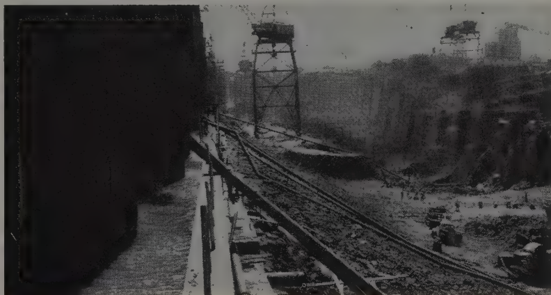
CONCRETE water collection flume catches infiltration through cofferdam and is a place to pump water from excavation area. Nine Johnson 5,000-gpm. pumps lift it back to river.
