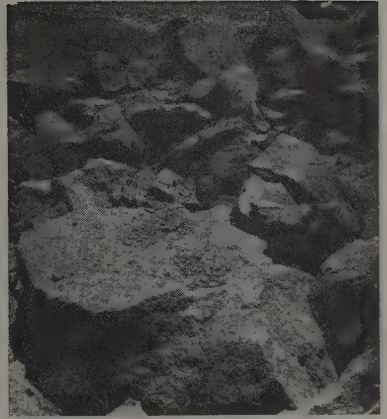
AFTER blasting, similar pieces were produced in the same location to hold a new 4-in. gravel blanket in place.
