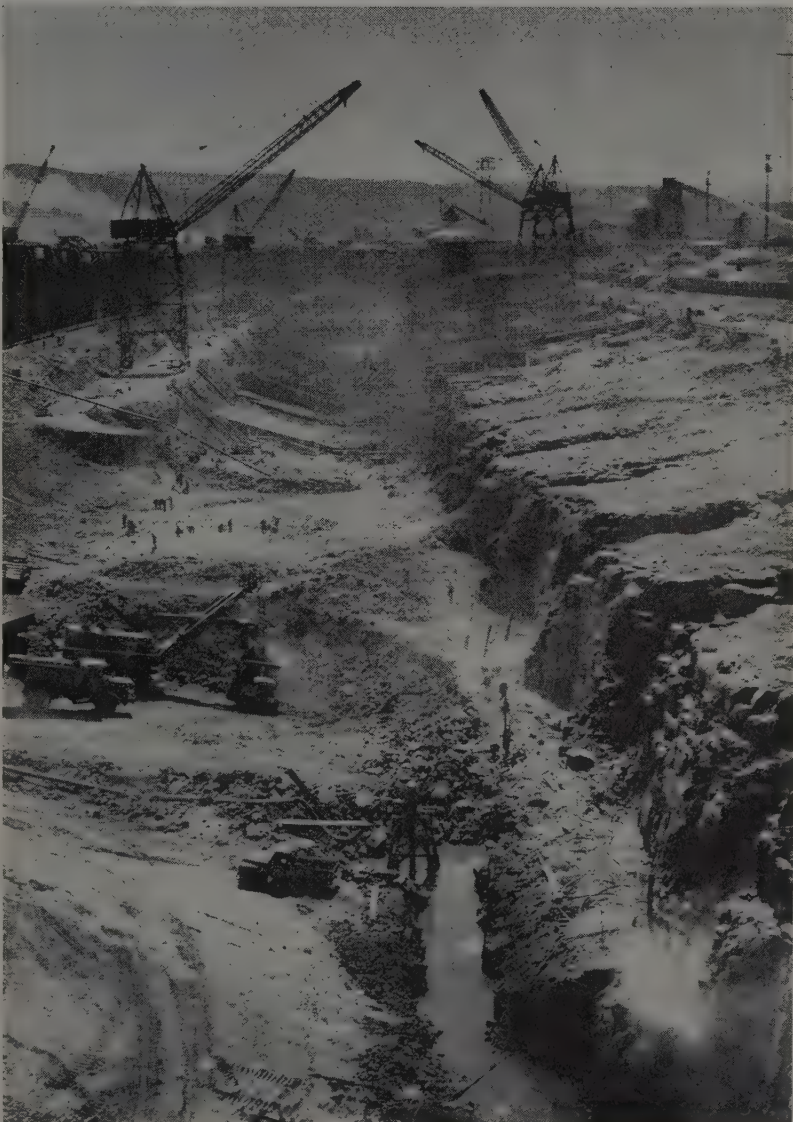
ABOVE—A Bucyrus Erie shovel, with 4-yd. dipper, has loaded up to 250 Euclid 16-cu. yd. truck-loads in one 8-hr. shift, while Cat D8 bulldozer keeps working area level. BELOW—Same area, drilling and shooting to 18-ft. depth is well ahead of excavation.
