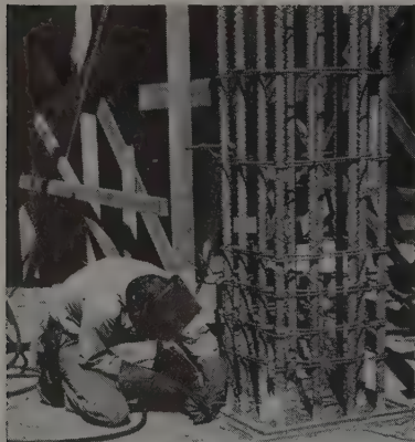
Welding Column Bars Saves $18,000 in Hospital Construction at Burlingame, California.
