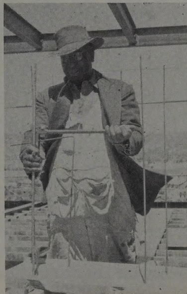
TOP RIGHT —Bender puts 90-degree kink in pencil rods.
