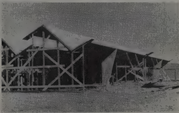
COMPLETED Z slab with forms removed except for supports at center and ends of cantilevered section.
