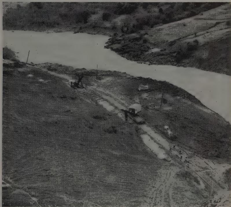
MATERIAL WAS BULLDOZED down face of slide at left, lifted over the tracks by shovels, and further bulldozed to river's edge.
