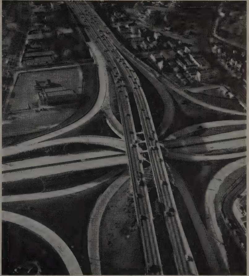
NEW FOUR-LEVEL traffic interchange structure provides maximum efficiency in less land area than conventional four-leaf clover traffic interchange.
