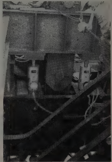
JACKS ARE SEATED (above) on bearing girder of the bridge tower and lifting the special girder that supports the plate links and concrete counterweight. Below, counterweight has imbedded steel anchorage to which cables are attached at left and lifting links at right.
