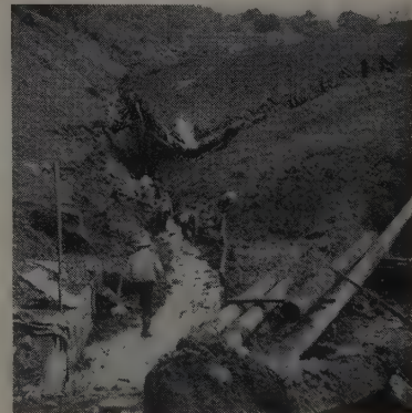
ABOVE , drainage water cascades from tunnel in Abbott Rock, part of work done in 1938. BELOW , up on the face of 1954 slide, men work to repair the broken drainage system and install new pipes in an effort to stop the earth movement.
