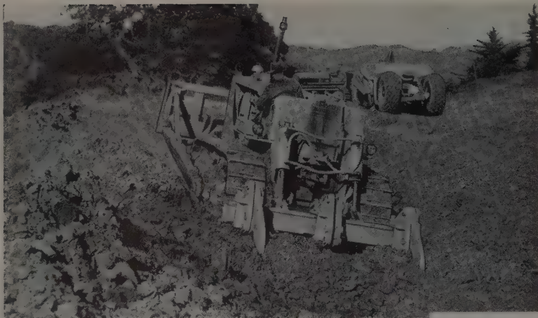
ATECO HRD8 rippers on Guy F. Atkinson Co.'s Waldo approach job, Marin County, Calif.
