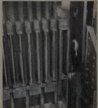
JACKS ARE SEATED (above) on bearing girder of the bridge tower and lifting the special girder that supports the plate links and concrete counterweight. Below, counterweight has imbedded steel anchorage to which cables are attached at left and lifting links at right.
