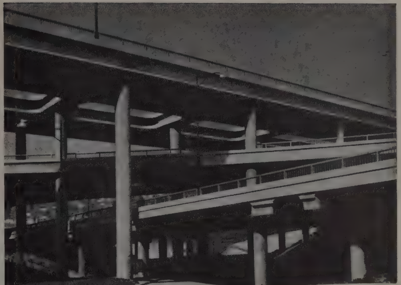
PHOTO COURTESY OF CALIFORNIA STATE DIVISION OF HIGHWAYS
