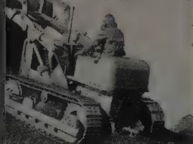
Backhoes sand, aggregate. Has action and flotation to work tight up on the pile.
