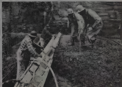
▲ These electric, two-man CP-5190's are ideally suited for knocking down and compacting harsh, mass concretes in open forms.
