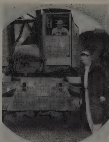
EASY DOES IT for Darrell Yearly (left), crane operator for Madonna Construction Co. as he jockeys a pipe section into place under the watchful eye of Leonard Hawkins, state inspector. A twist on the usual method of culvert installation is shown right. Contractor has permission to set pipe sections with inside tongue upstream. When joints are mortared and backfill is compacted, culvert will be tight.
