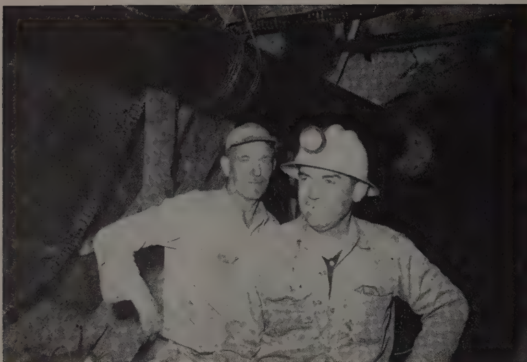
HEADING UP the work for Kiewit and Coker at Tecolote Tunnel ( Western Construction —April 1954, pp. 49-51) is Ray Blasongame (right) superintendent. Blasongame, who holed through Alaska's Eklutna Tunnel last fall, has brought key men to the new job, among them being Frank Weibel (left) master mechanic. Others on the job are A. M. Coker , project manager; Charles (Greaseball) Conrad , assistant superintendent; Don MacGregor , project engineer; Henry Franey , safety engineer; Ole Kusch , chief electrician; and Jake Omann , office manager.
