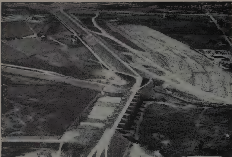
AERIAL PHOTO looking westerly across the spillway section of Whittier Narrows Dam shows work in progress on central embankment and floodway channel.
