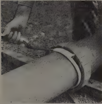
YARN SERVES as a sling (top) for pipe and helps centering by being in bell when stabbing spigot end. Caulking (bottom) is as easy as when older methods are used.
