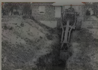
Trench hoe digs flat bottom ditch 27 in. wide to 8 ft. depth, 1/2-yd. bucket.
