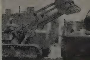
Cleans up rubble with one-cu. yd. tractor-width bucket.
