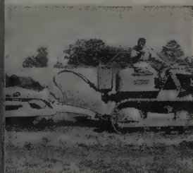
Does drawbar work scraping . . . grading.
