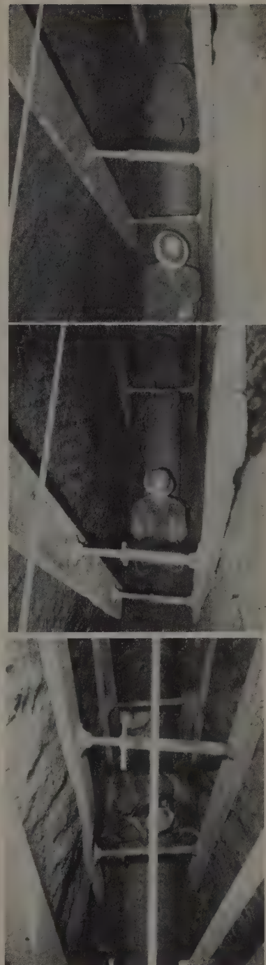
RESTRICTED AREA of 14-ft.-deep trench makes sling aspect handy (top); centering pipe and cutting yarn to exact length follows (center). Caulking is no problem in 17-ft.-deep wet trench (bottom).
