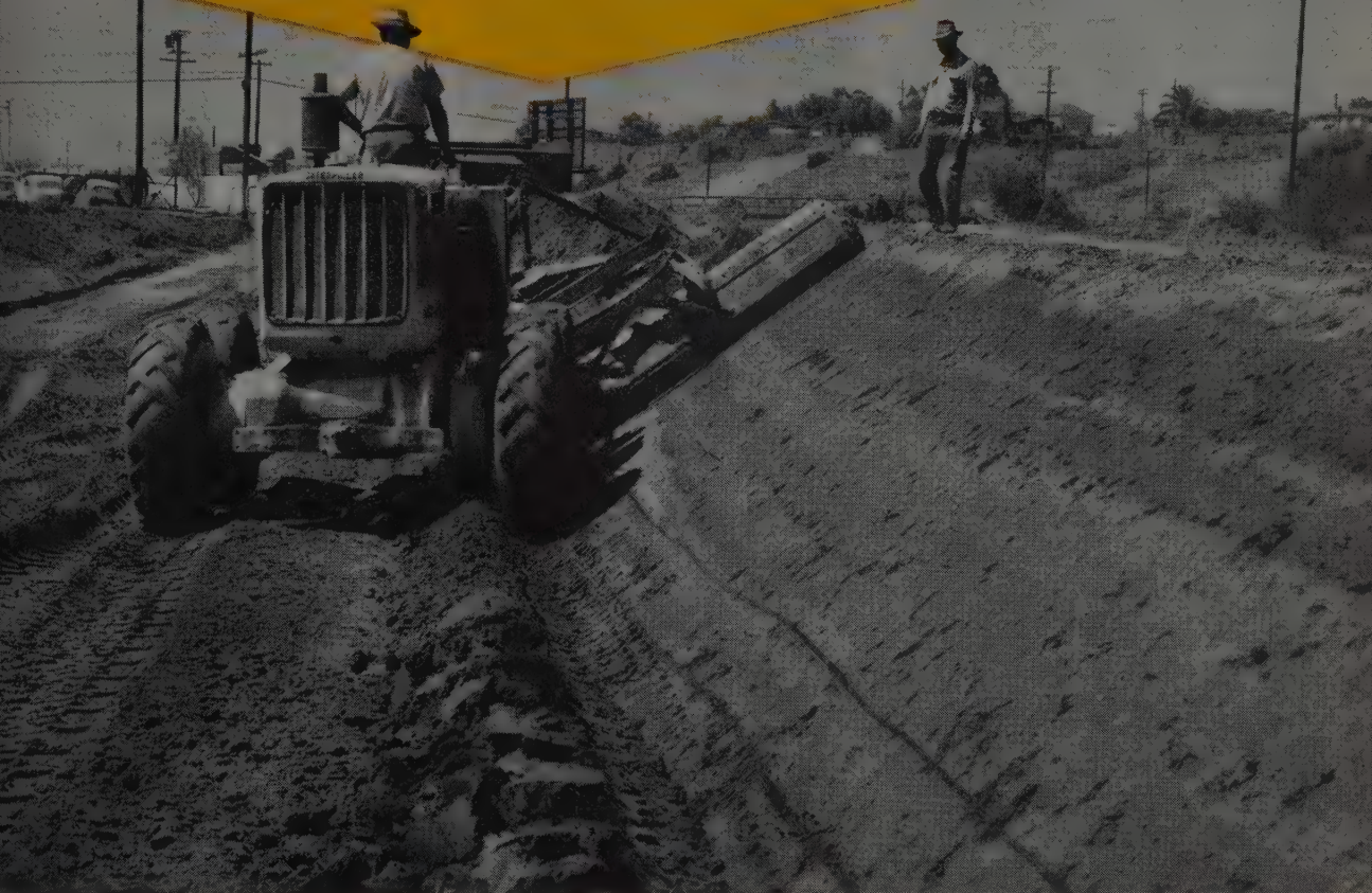
This No. 12 Motor Grader, owned by Daley Corp., is bank-sloping for a canal along the new Wabash Freeway, San Diego, Cal.
