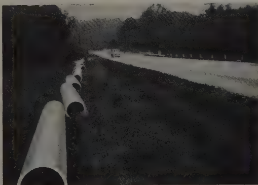
"Century" pipe awaiting installation along U.S. Route 1 — part of an 8000 ft. water supply line, 12" Class 150 pipe, from the Borough of Media Water Works to Middletown Township, Pa.
