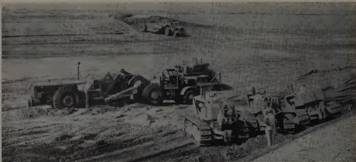
EARTHMOVING RIGS IN ACTION ON THE SAN GABRIEL RIVER
