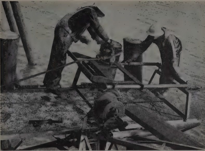
KEY FEATURE of the "gizmo" (above) is an air-operated chain saw mounted on a sliding frame. The frame rests on guide rails which run full length of the platform. This arrangement cuts piles to within 1/16 in. of grade. Piling (top right) are snubbed securely into position against platform by rope. Dogged drum is being tightened. Angle iron projections provide slot giving accurate center-to-center spacing of piling. Hand-turned screw jack (center right) raises or lowers this end of one of the two bent booms. Platform at far end of boom goes up or down in opposite direction. Boom rests beneath cap in lower foreground, then passes over cap of next bent. Cantilevered platform (below) is shown shortly after "gizmo" had moved to new location. Vertical piling has been snubbed into place. Note cable holding batter pile in position until preliminary cut-off has been made. Cable is from winch at other end of platform, similar to one shown here.
