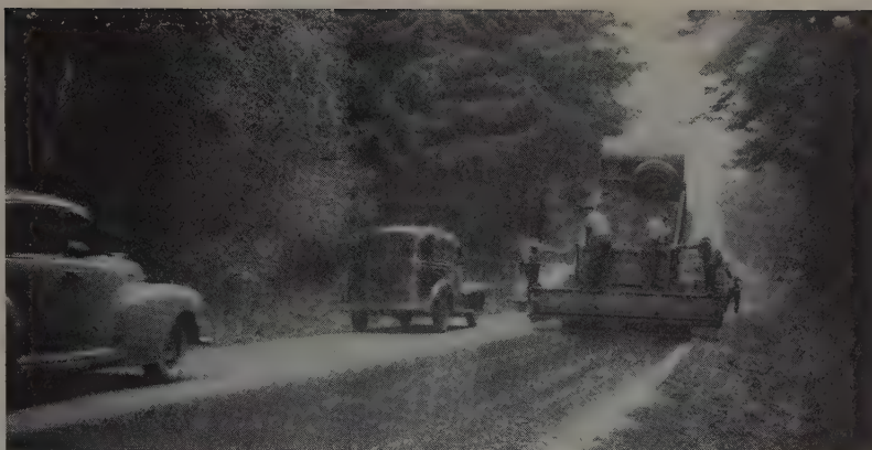
SPREADING screenings presents problems in obtaining a uniform spread quickly without spillage. Note spreading crew riding the spreader box.
