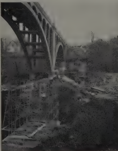
PIER 3 of the new bridge is in the foreground (left) looking toward the south abutment. Right is a closeup of Pier 2. Note steel I-beams through the pier which will support the bowstring trusses as falsework.
