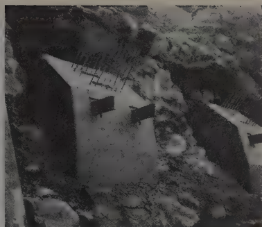
SKEWBACK rock excavations at the site of the Dunsmuir Bridge as shown by Martin Cornelius (left) and Reuben Sells, assistant superintendents. Right is the skewback after concrete was placed. Note steel I-beams for falsework trusses.
