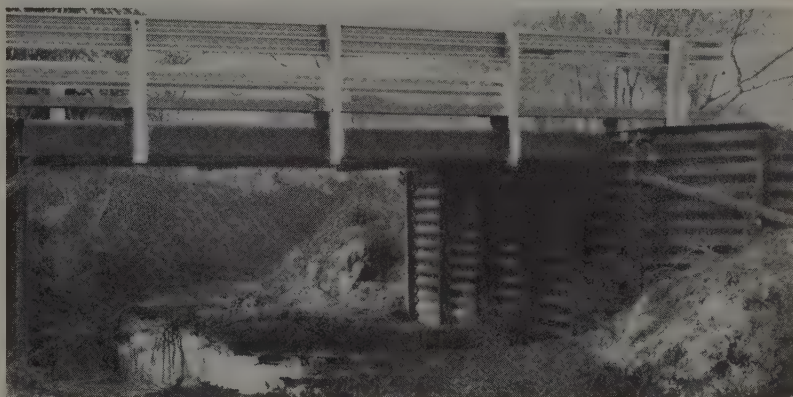
COREY BRIDGE —This is a hatch-cover span of 20 ft. These piles are made of 60-lb. rail, backed with Army surplus corrugated sheeting for abutments.
