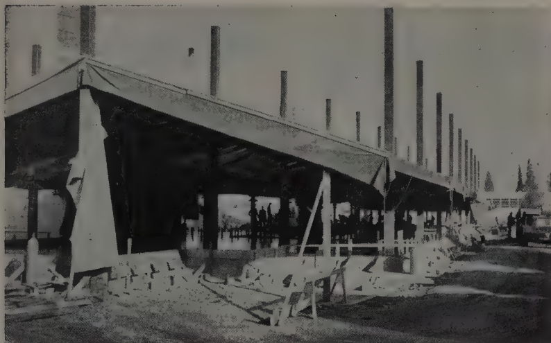
THIS TEMPORARY tent-type enclosure protected pouring of lift-slabs from the weather. After the pour was completed, the tent was removed.
