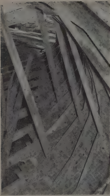
DRAFT TUBE THROAT FORM (left) is built in one piece, but designed for cutting into 7 pieces. One cut can be seen in this interior view, beginning at lower right and curving into the background at top center. Bolted timber members bridge cuts so that form can be handled intact for initial placement.
