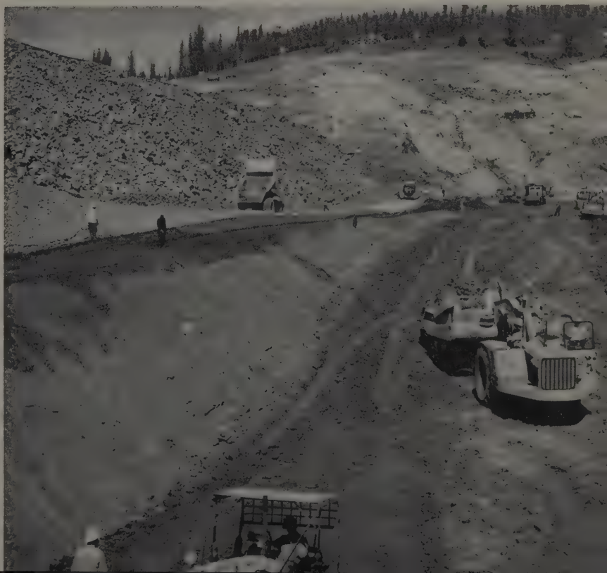
AERIAL VIEW above shows the dam area. Clay core for dam is completed, and last of main rockfill is scheduled to be finished within 20 days. The 234-ft.-high dam was built within two working seasons. Work on clay and sand filter zones is shown below three months before completion of dam.
