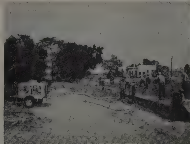
5. 105-c. f. m. Pneumapower providing air for backfill tampers.
