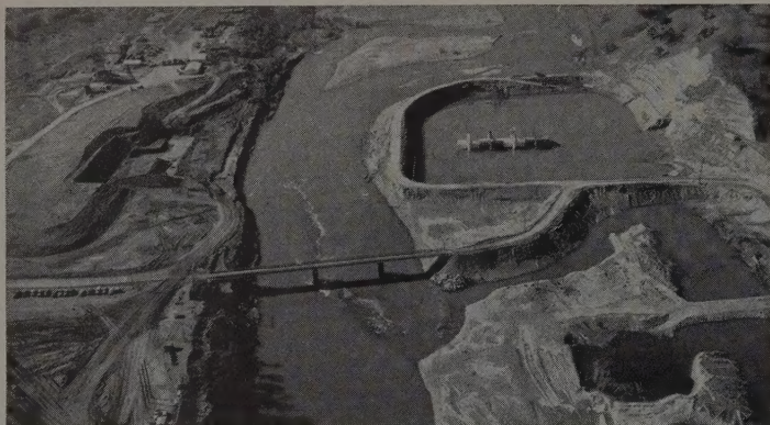
FIRST OF THREE floods came in January 1953. Work concentrated on left abutment during following winter months, using natural left bank for cofferdam, as shown here.
