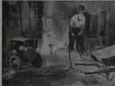
2. Model 35-c. f. m. operating demolition tool for removing concrete base.
