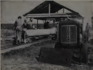
4. Model 60-c. f. m. furnishing air for paint sprays coating 65 mile of 20" pipe.
