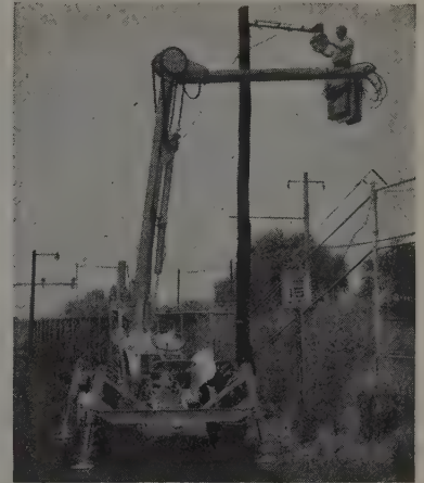
3. Schramm Pneumatractor with Sky- Worker solves overhead problems.
