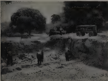
7. 315-c. f. m. operating three heavy duty rock excavating tools preparing new foundation.
