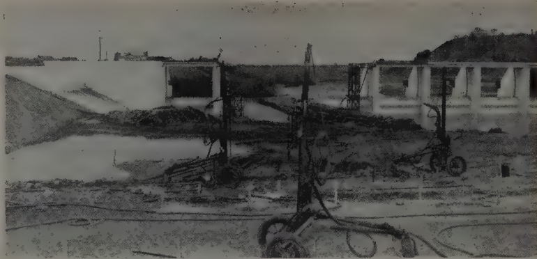
DRAFT TUBE THROAT FORM (left) is built in one piece, but designed for cutting into 7 pieces. One cut can be seen in this interior view, beginning at lower right and curving into the background at top center. Bolted timber members bridge cuts so that form can be handled intact for initial placement.
