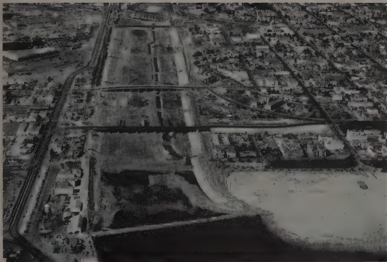
Aerial view shows cofferdam (foreground) and levees up to grade as—
