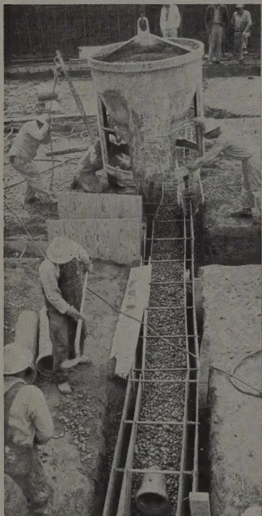
FILTER TRENCHES underlie downstream concrete apron. General view shows pattern, also method of handling graded filter material. Closeup of trench illustrates use of templates to place three grades of material in "circles" around perforated sewer pipe. The problem itself appears in the detail.
