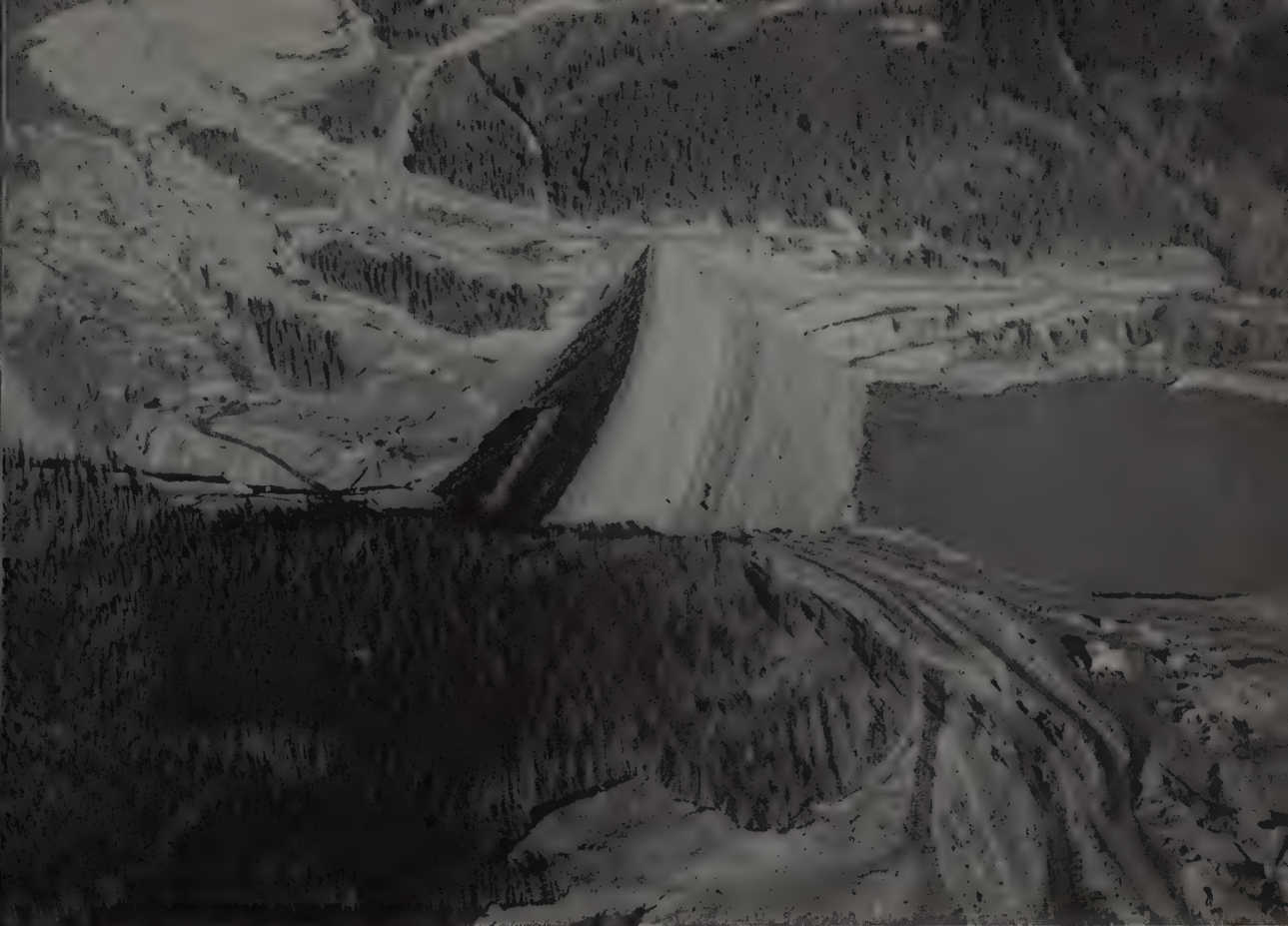
AERIAL VIEW above shows the dam area. Clay core for dam is completed, and last of main rockfill is scheduled to be finished within 20 days. The 234-ft.-high dam was built within two working seasons. Work on clay and sand filter zones is shown below three months before completion of dam.
