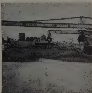
On this job, on which no spreader was used, the Paving Tube materially reduced the cost of spreading concrete.
