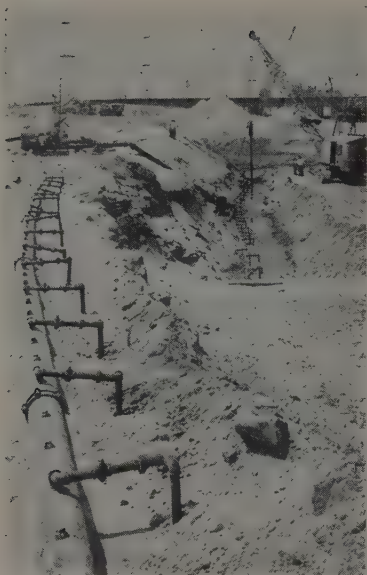
FIRST STAGE wellpoints (left) in submerged sill area. Second stage points (center) are to lower level of water table.
