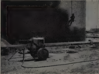
1. Model 20-c. f. m. operating paint spray for painting steel tank.
