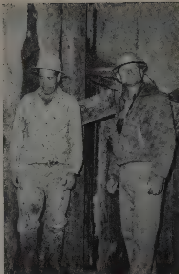
MINING FOREMAN Leo Durocher (left) and Superintendent George Trivitt check the shoring in the jacking pit. Steel sheet piling 30 ft. long was driven around the perimeter of the pit to keep the dirt walls from caving in.
