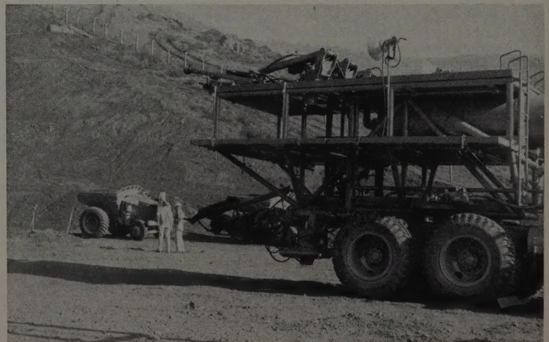
FIRST TIMBER (left) at the portal of a side drift is checked by Mike Roych (with folding rule) as tunneling gets under way. Atkinson's jumbo (right) was built to measure for this job, mounts 5 hydraulic jibs.
