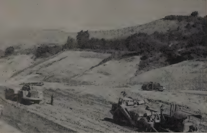
HEAVY GRADING on the four-lane highway between Monitor and Miller Street in Wenatchee, Wash., preparatory to applying the ballast and surface courses. This section of the road, when finished, will connect with the Wenatchee River bridge.
