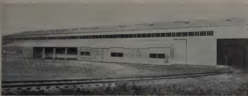
SOULE' STEEL CO.'s new plant and warehouse at Seattle, Wash., is built of steel frame with corrugated aluminum roof and siding. A 5-ton traveling crane serves the entire 355-ft. length of the building.
