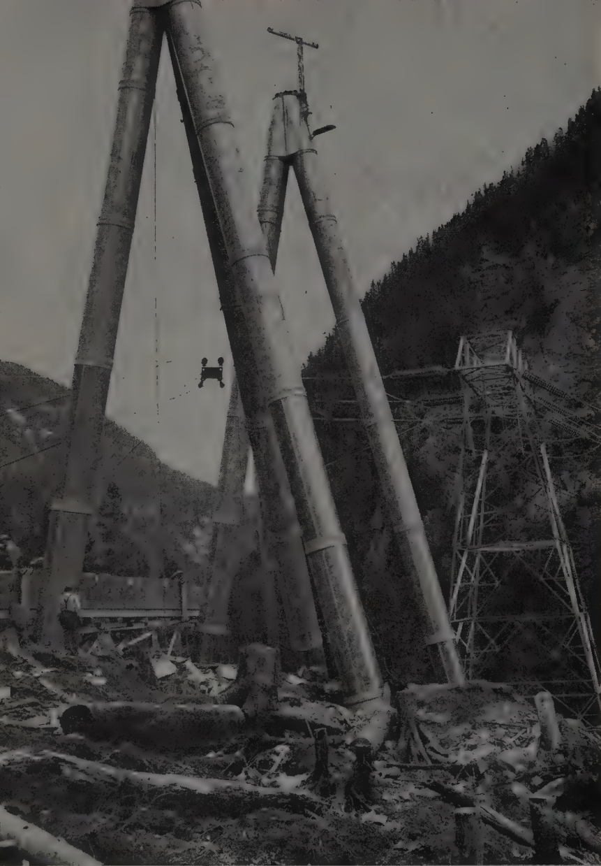
TUBULAR ALUMINUM towers weighing 22 tons each were introduced on the Alcan Project to carry one of two single-circuit lines over pass; steel towers, 42 tons each, carry the other. Both types are shown in this view. Note highline required to reach this site.
