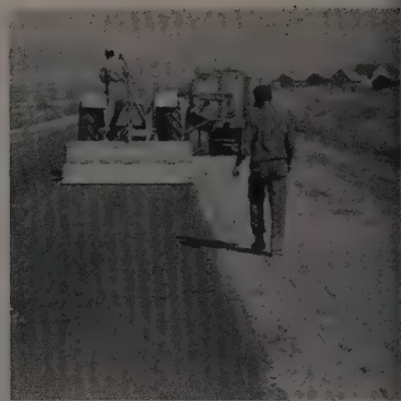
FIRST JOB of its type in Idaho was this Carl E. Nelson Co. contract to build 10 mi. of cement-stabilized base and plant-mix surface roadway in Bannock County. A Pulvi-Mixer and tank truck apply the plant-mix surface.
