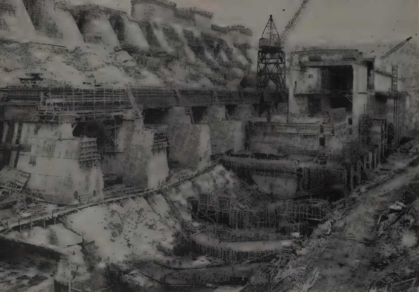
INTAKE AND POWERHOUSE construction at Chief Joseph Dam looked like this in November. This $40,000,000 job of Columbia River Constructors is the biggest of three contracts now in force totaling over $73,000,000.
