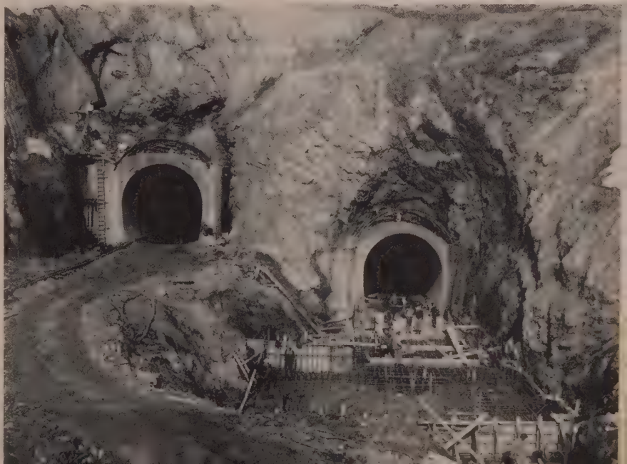
FULL-FACE DRIVING is proceeding with similar procedures and equipment at all four main tunnel headings. Job-built steel jumbos travel on gantry rails on 14-ft. centers, with 15 to 21 drills mounted on three decks of front section. Intake area is shown below with slab partially completed for transition. Tunnel No. 1 is at right, Tunnel No. 2 at left.
