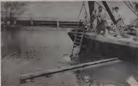
GETTING A RIDE on a barge (above), pipe is hauled out to site, then dumped into water for installation by diver (below).
