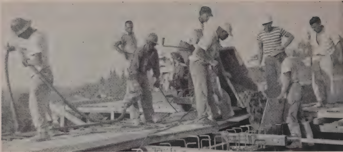
FAST WORK by powered concrete carts is reflected in a better pace for the whole placing operation, more efficient use of vibrators, form men and finishers.
