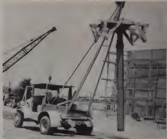
EASILY MOVED from caisson to caisson, tremie is lifted clear by cables from truck's winch.
