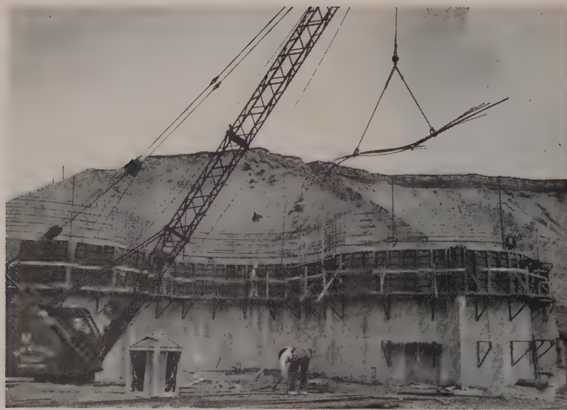
THIS CURVED wall will hold various sizes of sand and gravel in the bunkers formed by its 15½-ft. radius curves. The wall is 40 ft. high.
