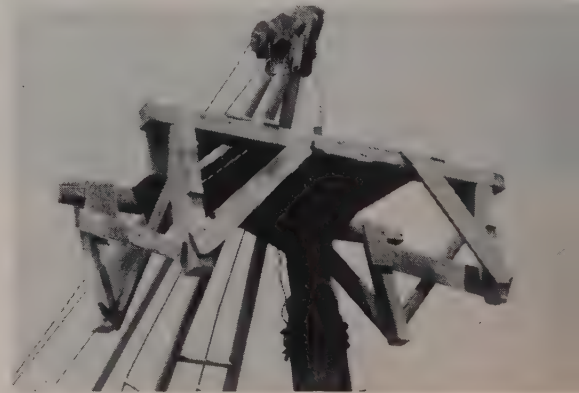
CLOSE-UP of the tremie's four 11-ft. sections telescoped, hopper and tremie head.
