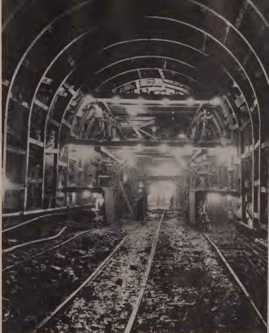
FULL-FACE DRIVING is proceeding with similar procedures and equipment at all four main tunnel headings. Job-built steel jumbos travel on gantry rails on 14-ft. centers, with 15 to 21 drills mounted on three decks of front section. Intake area is shown below with slab partially completed for transition. Tunnel No. 1 is at right, Tunnel No. 2 at left.
