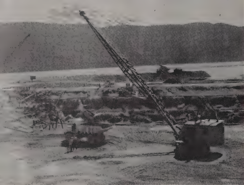
INTAKE INVERT 60 ft. below natural level of Tahtsa Lake required dewatering of work area within cofferdam. Wellpoints and pumps remove up to 11,000 gpm. of water infiltrating from the lake. Included in facilities for intake are six sets of trash racks and trash rakes and a 15-ton traveling crane.
