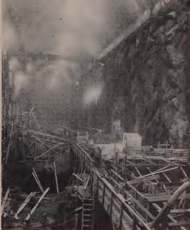
POWERHOUSE with arch concreting completed and turbine pits being excavated. Looking south, penstocks enter from left and tailraces go out at right. Initially, powerhouse is 700 ft. long, 140 ft. high (from bottom of pit liner pads to top of arch), and 83 ft. wide, and will house eight turbines. Ultimate length of the powerhouse is 1,100 ft. to accommodate 16 units.
