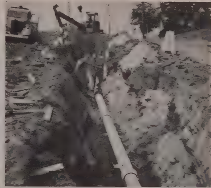
Because "Century" pipe is so easy to handle and assemble, the laying crew works right on the heels of the "digger".
