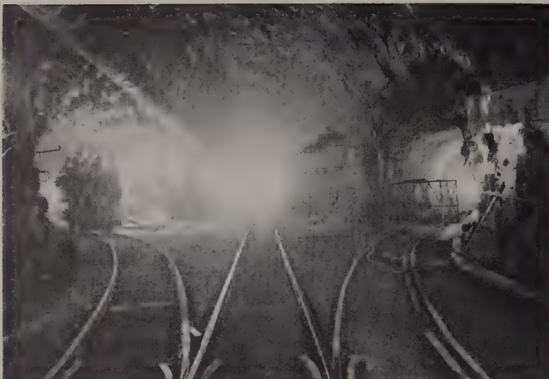
AT THE 2,600-FT. "Y", looking toward portal of power tunnel adit, with the two penstock branches veering to left and right. Butterfly valves will be installed in chambers at this level.
