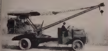
The first truck crane — 1918 model
