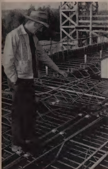
A.K. EMBREE, superintendent for Brezina Construction Co., indicates 4-in. fibre ducts installed on their job to house electrical services. The ducts are a fine idea, but must be secured so as not to float out on a slab pour. Contract is a $758,350 administration building at Fort Rich. Progress is past 40%, with about 40 men on the job. Chris Lee is project manager. For the Army, O. W. Urbom is project engineer and John Holland is inspector.
