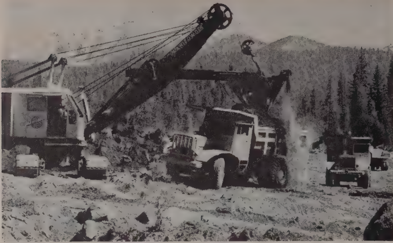
AT THE SITE of Vermillion Dam and reservoir construction in central California, one of the fleet of Kenworth 801 earthmovers takes on a load of excavation from a Manitowoc shovel for the 477,000 cu. yd. to be removed from the damsite. This large earthfill dam, being built for Southern California Edison Co., will require 5,135,000 cu. yd. of material, and the reservoir will have a capacity of 125,000 ac. ft. Bechtel Corp. holds the prime contract for the $8,500,000 project.
