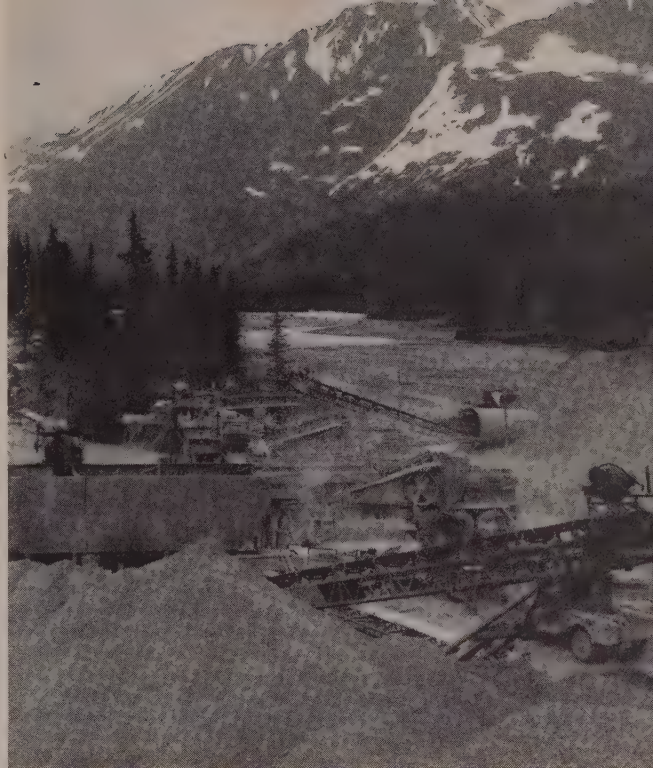
THE DUST of construction activity can never top the mountains of the Kenai Peninsula, where Rogers Construction Co. and Babler Bros. are completing surfacing of the new Anchorage-Seward highway for the Bureau of Public Roads.
