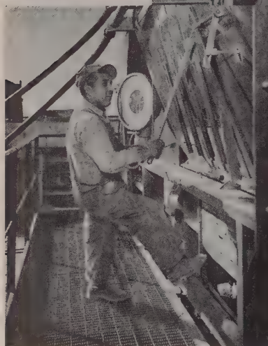
Easy motion type controls and scales are located so as to provide a minimum of movement and effort by the operator.
