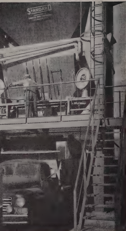
4000 lb. capacity plant at Industrial Asphalt, Los Angeles, California
