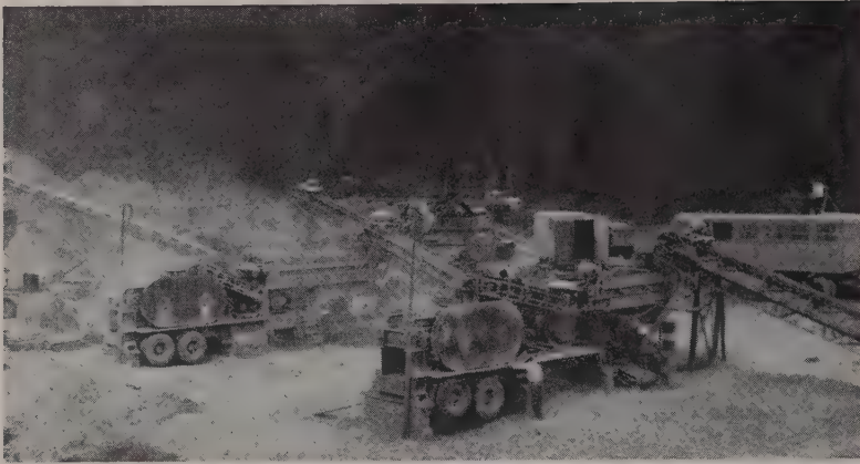
PANORAMA shows contractor's crushing and screening set-up, except for jaw crusher. General features of portable design are evident here, as DW10 and W10 wagon load out of bins in left background.
