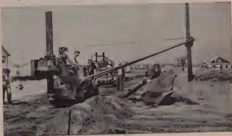
Here, a Cleveland Model 80 is speedily and cleanly backfilling the trench shown in the top picture. The 80 is also an excellent pipe layer. When job conditions require backfill compaction, the 80 does an outstanding job with no additional men or equipment necessary.
