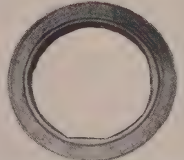
Old line after reconditioning by Pipe Linings, Inc.
