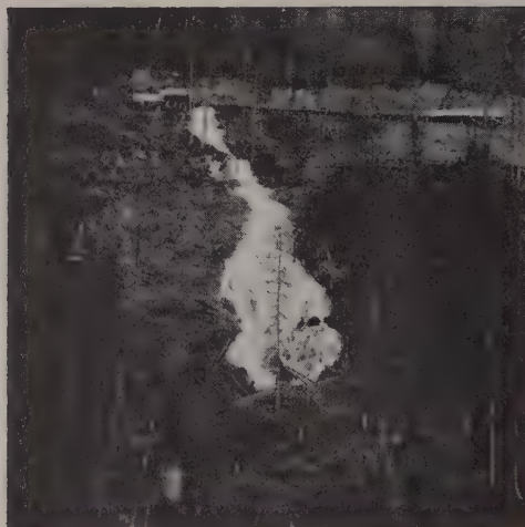
PRETTY FAIR flow for a tunnel that isn't even holed through! Wasting down the hillside from the adit of Eklutna tunnel last November was 7,800 gpm. Maximum flow from bad spot at Sta. 208 + 75 was 16,000 gpm. Uncontrolled, the water ponded behind a highway embankment below, threatening that structure until the contractor breached it and installed a culvert. Even at Sta. 213 + 82 there was a lot of water, as shown by this view (right) at the contractor's weir. Before extra fan lines were installed to carry the water it spread across the full tunnel width in a knee-deep stream.
