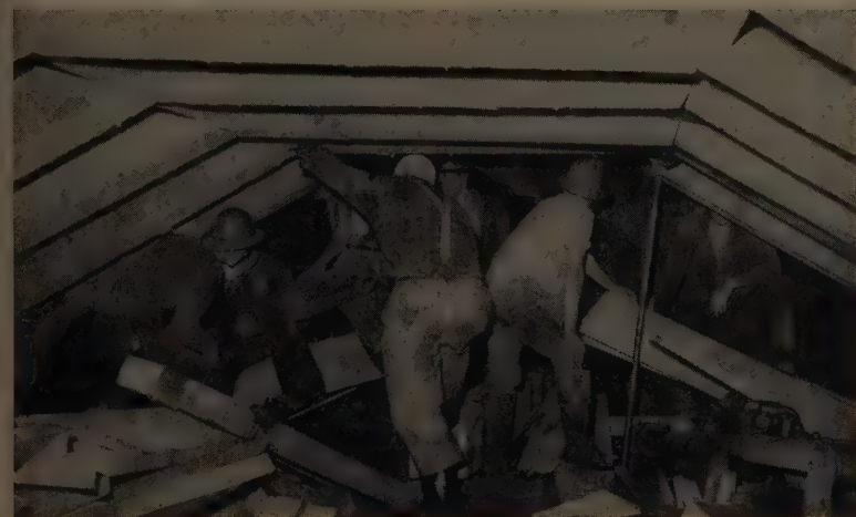
SUPPORT WORK after each round goes fast. The jumbo is held back while plumb posts are set, then moves in against the face so that miners setting arch support can work from the top deck. Timber segments, crown bars, bracing and blocking are all hoisted topside by the cherry picker, a whole carload at a time.
