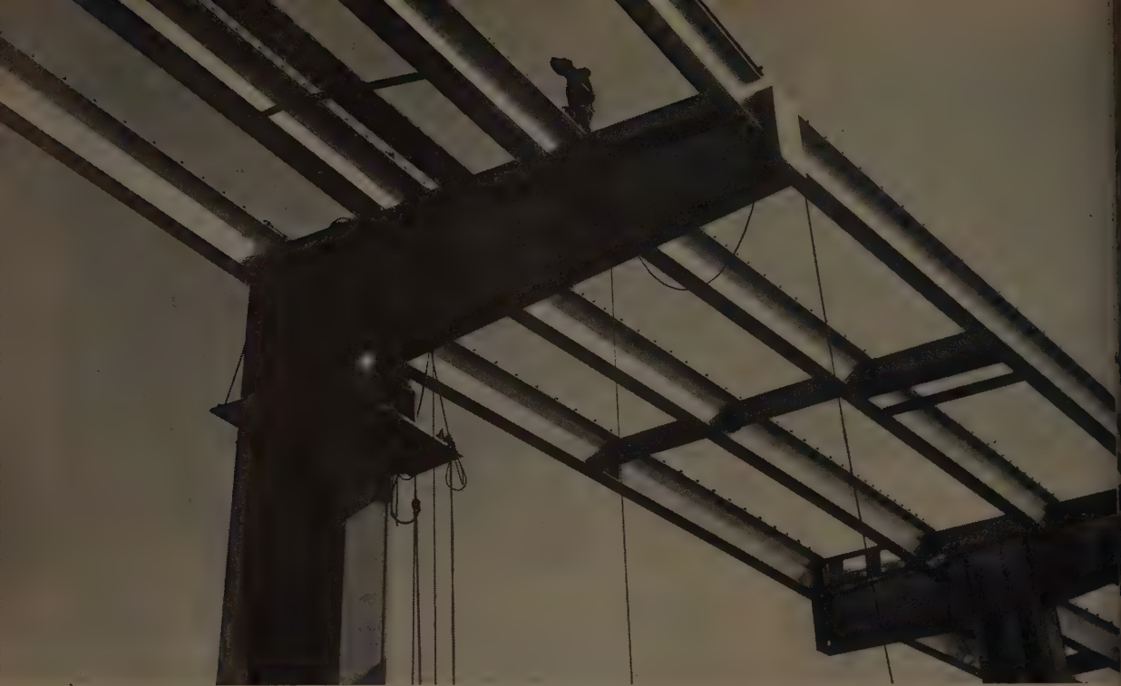
30,500 TONS of all-welded steel, with plate thicknesses to 2\frac{1}{2} in., required techniques that push forward the frontiers of welding science.
