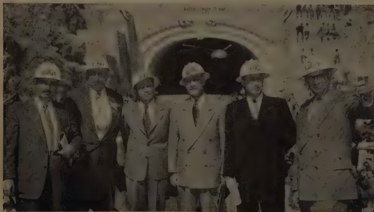
PRESIDENT Del Fisher of Fisher Contracting Co. is pictured at right pointing out roadway connecting Queen Creek bridge and tunnel at the ceremonies dedicating these major engineering improvements in the State of Arizona. Participating officials (all decked out in Fisher "hard boiled" hats) are shown from right: Louis Escalada , former chairman of the State Highway Commission; Fred D. Schemmer , Highway Commission member; John Scott , vice chairman of the State Highway Commission; Arizona's Governor Howard Pyle ; Reverend Larsen , who gave the ceremonial invocation, and Fisher. Entrance to the tunnel is in background.
