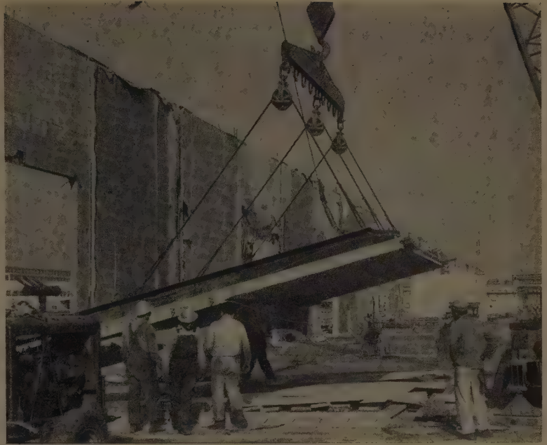
PRECAST WALL PANELS, 23 ft. 2 in. wide and 30 ft. high, were cast inside building area on top of first course of asphaltic concrete floor. For placing, crane picked up 27-ton panels by means of heavy steel H-frame bolted to panel.
