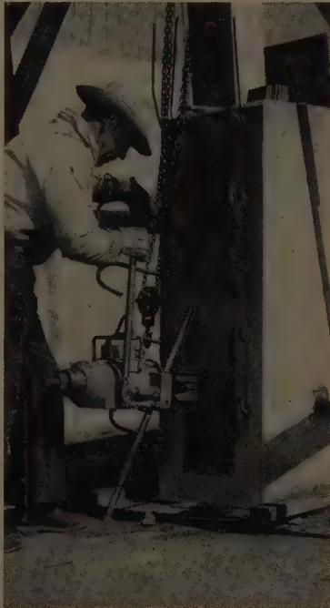
CABLES were tensioned from both ends of girders by hydraulic jacks fitted over end anchors. It was found that two men could stress the twelve cables in one girder in about four hours.
