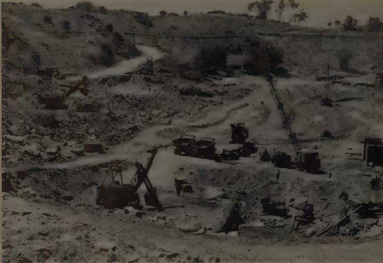
TAKEN from the upstream cofferdam at mid-channel, this view of Folsom Dam site shows the situation in the latter part of July. The truck crane is resting on gravel which buries Block 14 to a depth of 30 ft. Two Northwest shovels are in evidence, one of them above Block 15, and the other about at the toe of Block 15. The Marion shovel at the left is doing rock excavation for the left training wall downstream from Block 17. Just below it are concrete footings from which the January flood swept a trestle bent.
