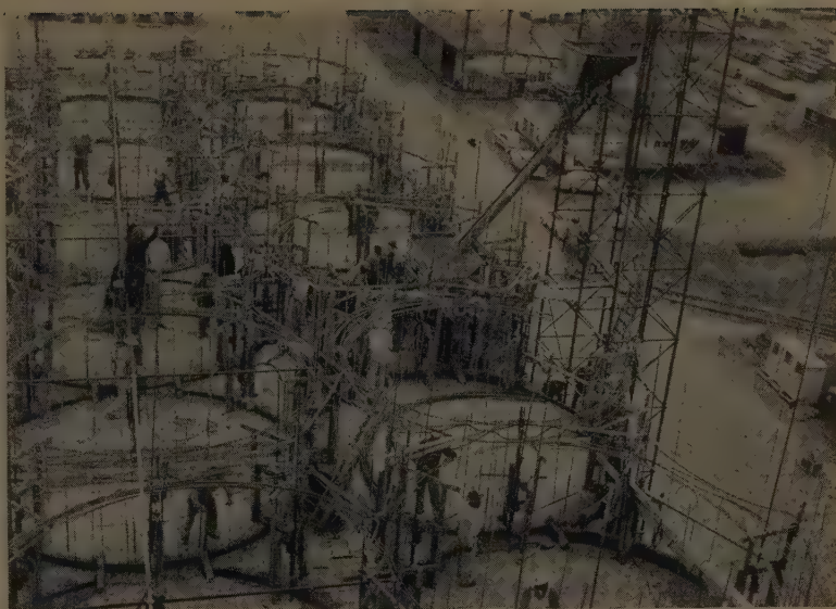
THERE'S NO time for dawdling when a slip-form pour is on a 24-hr. schedule. Concrete buggies are concentrated at the twin hopper (center right) at the same time more reinforcing steel is being placed (center left) and members of the jacking crew lift the form the requisite number of notches.
