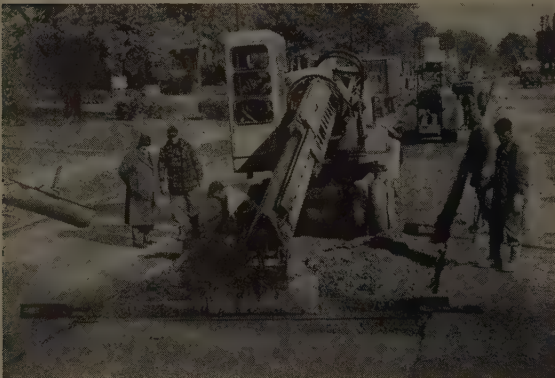
DRIVING test piling for a proposed new bridge to replace the longest wooden bridge in the United States is a 20-ton Lorain Moto-Crane, Model MC-414, operated by a Hansen & Parr Co. crew (above). The barge, appropriately enough labeled "The Thing," is in Lake Pend Oreille, Idaho. The present bridge extends across the end of the lake near Sandpoint.
