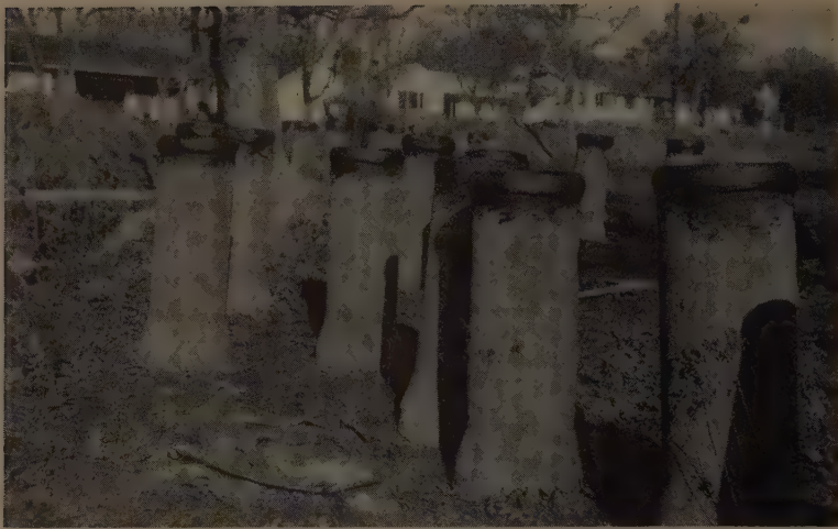
LENGTHS of 8-in. pipe have been coated with sealing mastic and stand ready to be placed in the trench as part of the "Country Club Park Addition" to the Medford sanitary sewer system.
