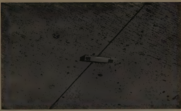
PROPERLY TIMED sawn joint is neat and straight, with a minimum of raveling at the edges. An absolutely clean joint indicated that the pavement had set first, and random cracking may therefore have already taken place.
