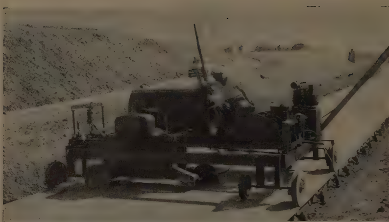
DEVELOPED especially for pavement joint work, the multiple-bladed saw is self powered along the pavement headers, has independent power for the transverse carriage mounting the blades.
