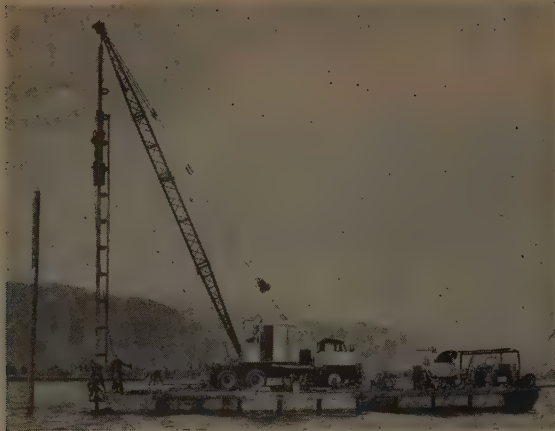
DRIVING test piling for a proposed new bridge to replace the longest wooden bridge in the United States is a 20-ton Lorain Moto-Crane, Model MC-414, operated by a Hansen & Parr Co. crew (above). The barge, appropriately enough labeled "The Thing," is in Lake Pend Oreille, Idaho. The present bridge extends across the end of the lake near Sandpoint.
