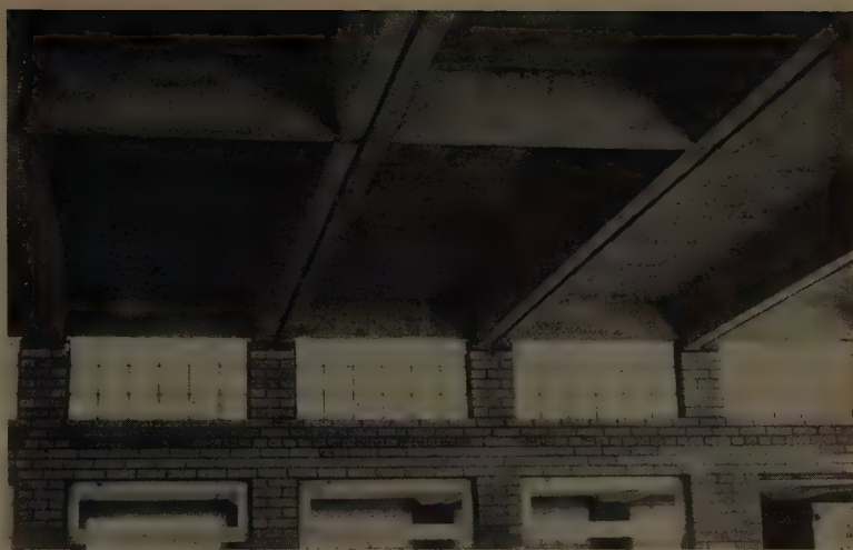
THIS IS HOW the roof looks directly following erection and before the final grouting. The flanges will remain exposed, but they will be painted and acoustical tile will be cemented directly to the bottom surface of the web.
