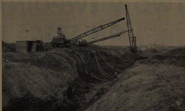
SLOUGHING BANKS and water problems characterized work under normal scheme of open-cut excavation. Using bentonite slurry, trench width was barely more than that of dragline bucket.
