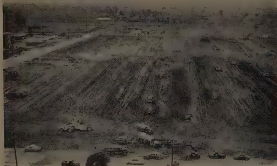
LOOKING DOWN from a hovering helicopter on the 16-acre cut and fill job, accomplished in less than 20 working hr. by the Los Angeles Excavating and Grading Contractors' Association.
