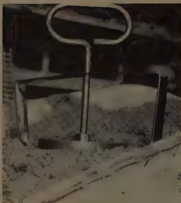
CLOSE-UP of the Kelly Ball in action. If it sinks too deep, back goes the batch to the mixer for more material.
