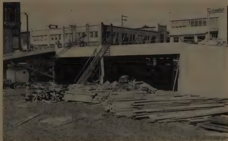
SOUTH PORTAL is a skewed structure, its alignment showing how subway cuts under corner of Film Exchange Building (right). Approaches to subway are part of the contract, and total 2,000 ft. in addition to the 2,134-ft. subway.
