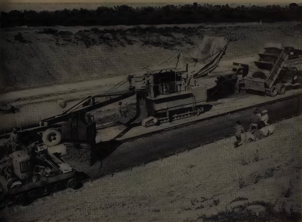
Paving the new Santa Ana Freeway
