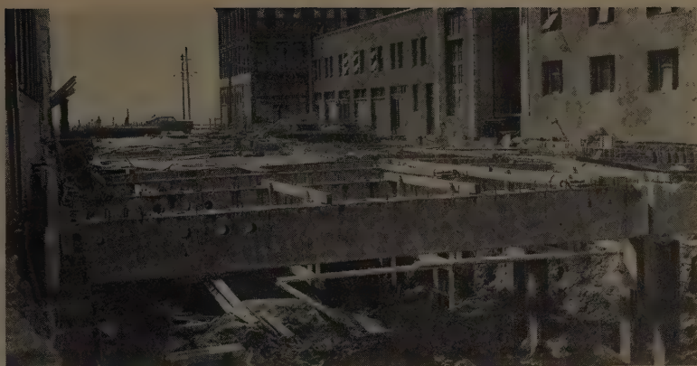
TOPSIDE of work shows shallow cut made initially to receive concrete beams, which are seated on H-piles at centerline of divided structure and on concrete poured at 15-ft. intervals between H-piles underpinning abutting property. Temporary timber roadway over these beams gives access for equipment on later pouring operations along center wall.
