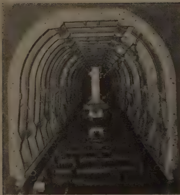
SPECIFICATION AND RESULTS are shown here. Drawing indicates lining for two types of tunnel. Reinforcing steel is placed only as directed—little has been used. Collapsible steel forms establish flat crown, leaving room above for slickline as concrete is placed.
