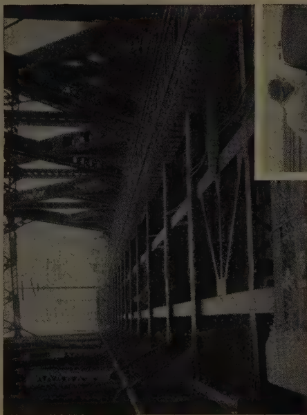
▲ Fig. 3. Double track right-of-way on Shaker Heights Rapid Transit System. Weakened cross braces were replaced in minimum time with arc welding.
