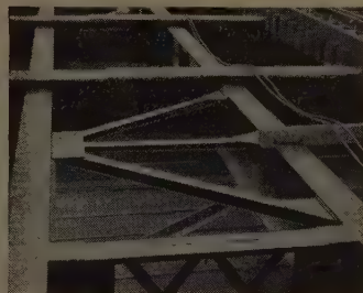
Fig. 1. Rusted-out Braces originally riveted to flanges of bridge girders are cut out quickly with torch.
