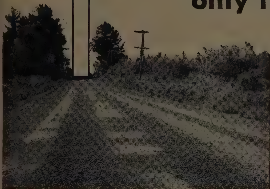
A gravel road in which bumps, undulations and rippling are developing because of gravel segregation. The loose gravel between wheel paths is dangerous and wasteful.
