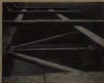
Fig. 2. Faster Construction. Angles sawed to length are fillet welded to web of girder with Lincoln "Fleetweld 5" type electrode.
