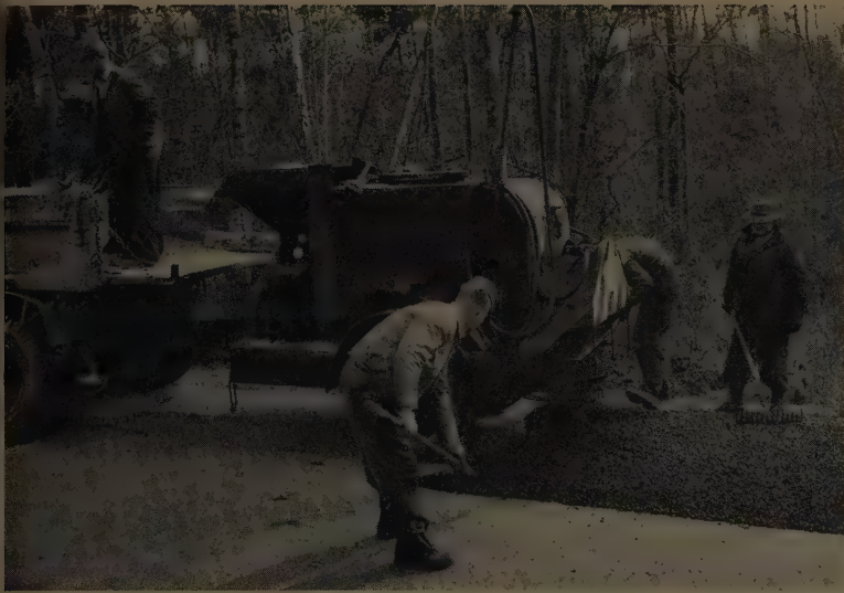
FEATURE of the Hetherington and Berner Moto-Patcher is a 400-gal. storage tank which keeps the asphalt hot at all times.
