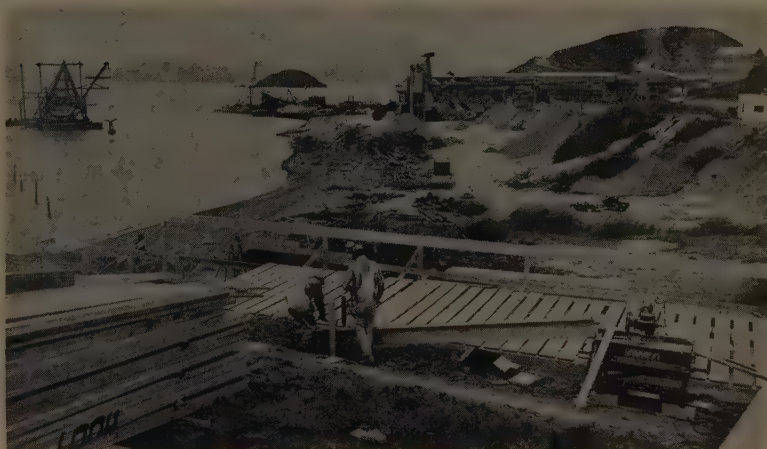
FIRST CONSTRUCTION on the San Rafael-Richmond (California) bridge across the northern part of San Francisco Bay is a $16,000 office building for engineers, shown going up here on the Richmond side of the Bay. The dredge (left) is clearing the way for four 12 x 36-ft. piers. The first steel pilings were driven early in April to prepare for the permanent structure. The $14,234,550 contract for the substructure went to Ben C. Gerwick, Inc., and Peter Kiewit Sons' Co. ( Western Construction —February 1953, p. 119). The job is expected to take 3½ yr. and employ a crew of 2,000 men at the peak of operations.
