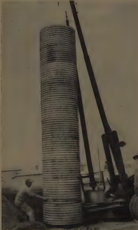
LOWERING a 35-ft. section of corrugated metal pipe, workmen complete installation of an improvised storm drainage system at an El Segundo, Calif., street intersection.
