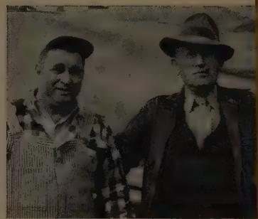
PRELIMINARY WORK for a proposed dam and powerhouse near Bliss , Idaho is carried on by John A. Wardle (left) a catskinner, and D. C. Thomas , job superintendent.
