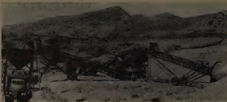
STIFF BASE COURSE specifications on the new 55-ft. expressway between Salt Lake City and Parley's Canyon were met by this portable 46VE plant. It turned out an average of 750 tons of material per 8-hr. shift for Parsons & Fife, contractor.
