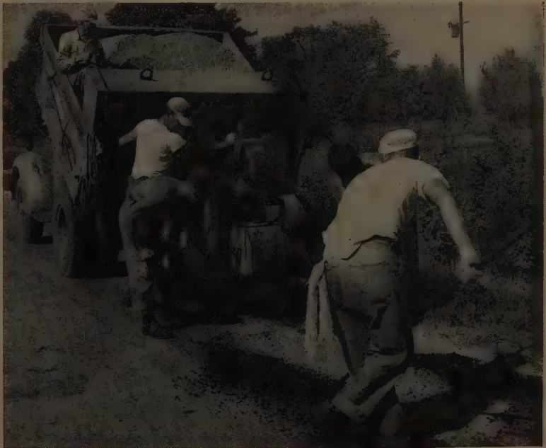
THE McCONAUGHAY Multi-Pug Mixer tosses the material back and forth through four series of blades, providing a thorough mix.
