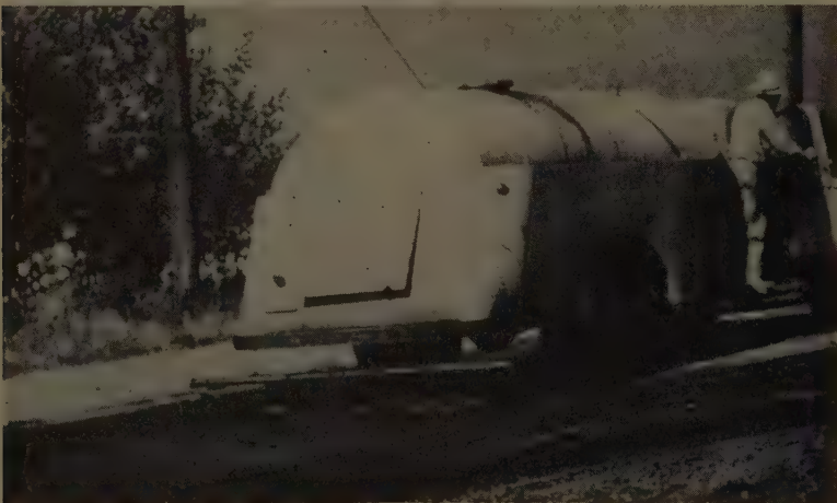
THIS STREET FLUSHER has been converted to a sprinkler for the purpose of applying emulsion mixture. Equipment belongs to the city of Renton, Wash.
