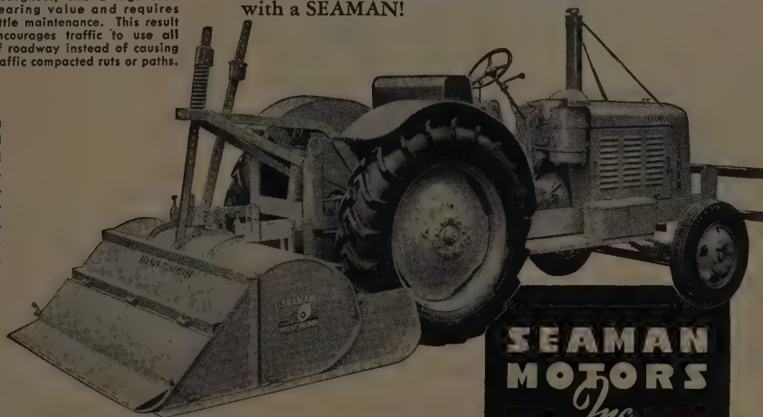
The Seaman Self-Propelled Pulvi-Mixer, 7 foot mixing width. Gasoline or diesel powered. This unit will mix and finish one mile of 3 inch oil mix at a cost of less than approximately $50.00.
