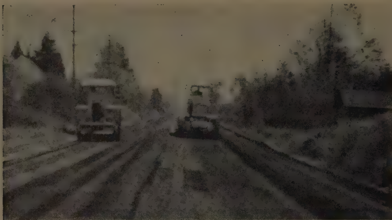
ROLLER starts compaction on section of highway in Multnomah County, Ore., while motor grader lays out processed surfacing.
