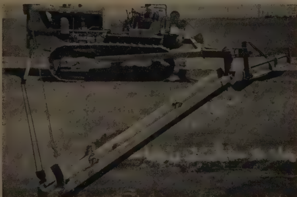
SLOPING NEW CANAL BANKS— California Central Valleys Project
