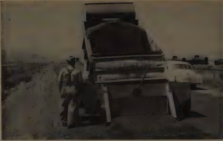
THIS ADJUSTABLE spreader box was used by Hector to measure the amount of cinders added to his road mix in Klamath County, Ore., where he worked before he went to Douglas County.
