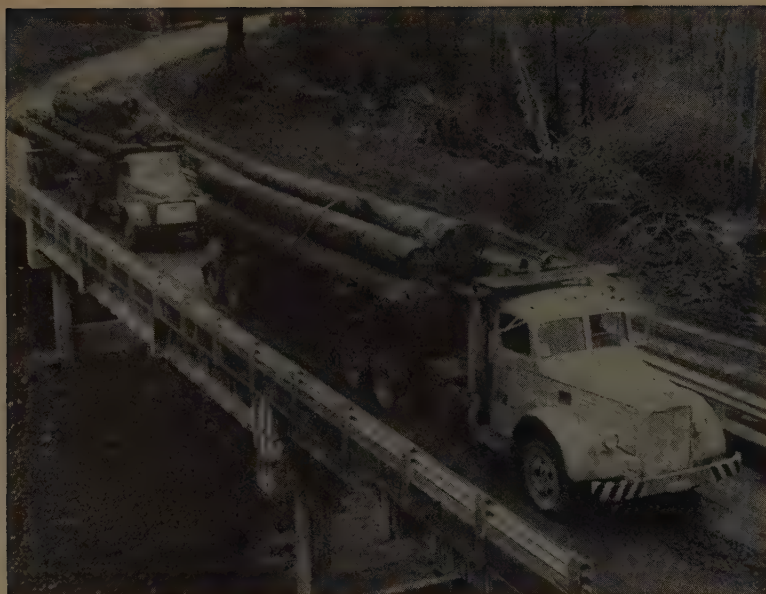
TRAFFIC LIKE THIS required permanent bridge construction on backwoods haul roads. Burma Bridge over Calawha River west of Port Angeles is one of the new prestressed structures.
