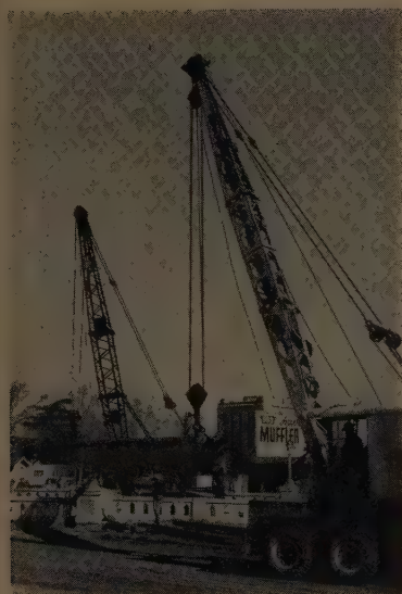
SQUARED AWAY (left) with an 18-ton beam after picking it up from casting area behind crane at right, the two cranes move out together under directions from boss rigger.
