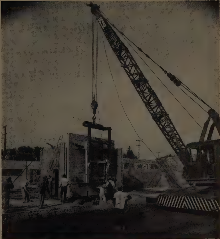
VACUUM LIFTING of interior wall slab with truck crane from casting bed. Walls were erected at the rate of 16 sections per day.
