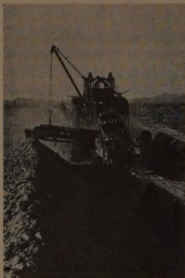
THIS DIGGING looks easy, but sandstone wore out bucket teeth in one shift. About two-thirds of the job was like this, and ditching progressed at better than 1 mi. per day.
