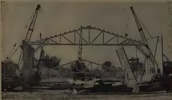
THREE CRANES cooperate to raise a prefabricated building in one working day. A crane on each side lifts a wall section into place while the third stands by with a roof truss to be welded to the walls by steel connecting plates.
