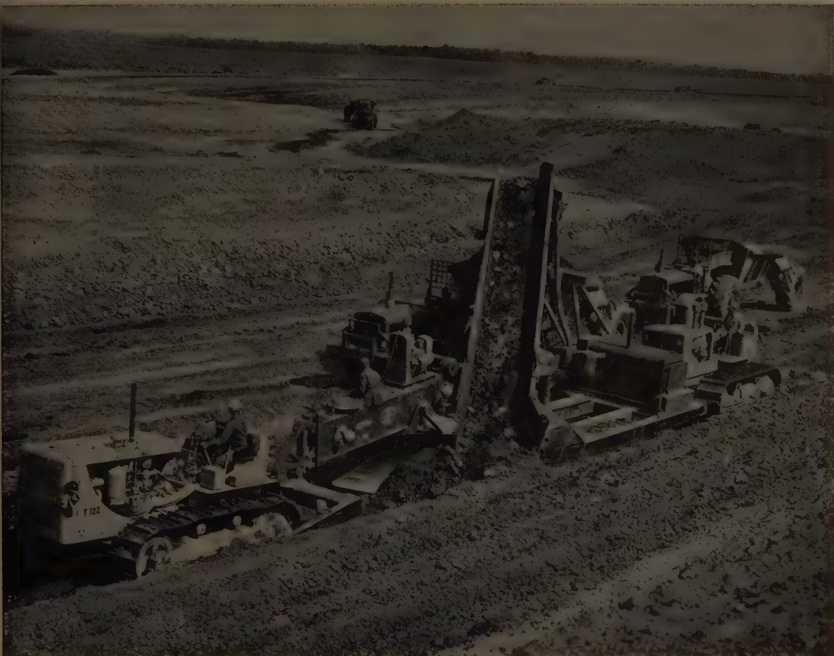
Excavating for the new Alcoa Plant in Borger, Texas
