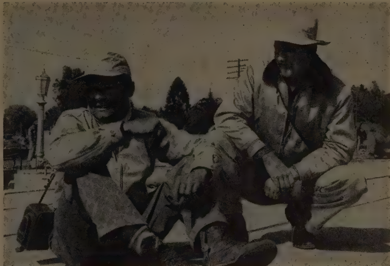
ANSWERING QUESTIONS , Tom Bezouska (left) and Walter Joens of the Division of Highways perch on one end of the bridge and face the "gallery." Joens is resident engineer on the job; Bezouska is assistant resident and designer.
