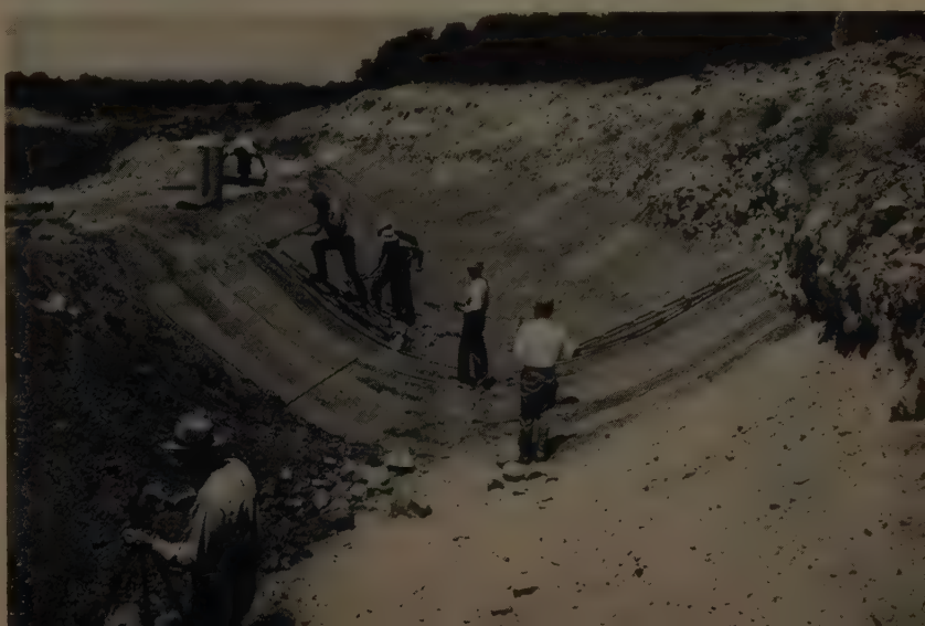
PREFABRICATED membrane required most fine grading ahead of time, gave better service than sprayed-on counterpart. Sprayed asphalt went on unrolled subgrade having such rough areas that distributor-mounted spray bar had to be replaced by hand-operated rig.
