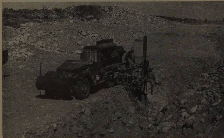
HERE'S THE THING for this country: A drill set-up on a half-track. Eight of these drilled the pipe alignment preparatory to blasting a 5-ft. trench.
