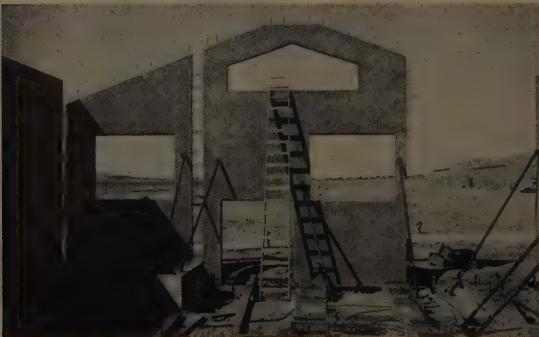
PANELS (above) come before frames on this barracks. Note adjustment on braces used to plumb the wall during erection. Wall panels (below) come in all shapes and sizes, with unsymmetrical openings as shown here.
