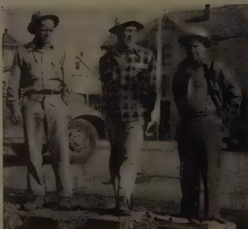
LOOKING OVER the Stolte, Inc., job to replace an outmoded storm drain with reinforced concrete pipe (see page 70) are (from left) Robert Bowen, pile-driving foreman, Bill Cole, superintendent, and Ed Strangard, Oakland construction inspector.
