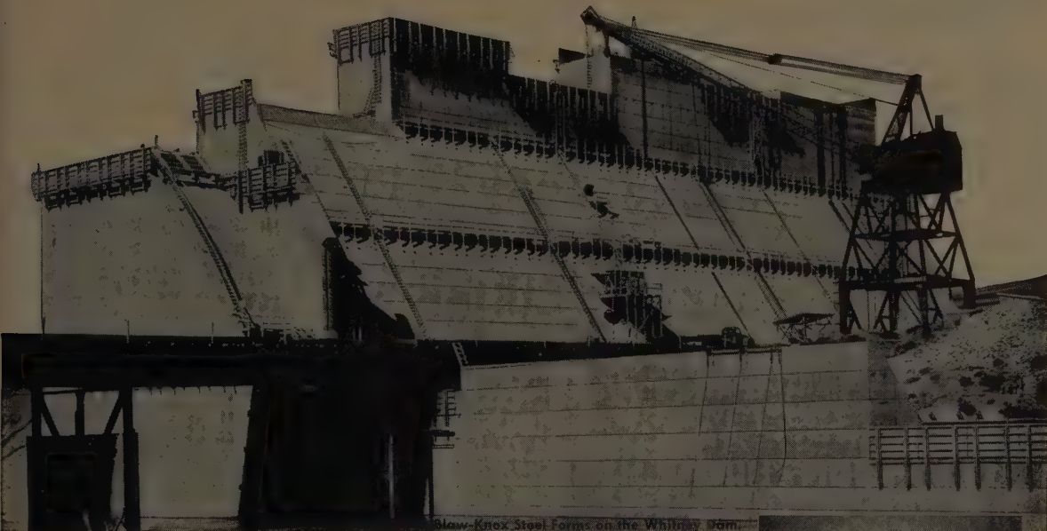
Blaw-Knox Steel Forms on the Whitney Dam.
