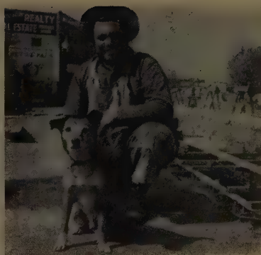
AN UNUSUAL sort of sidewalk superintendent is "Boots," who stops to chat with Louis Loper, general foreman of the box culvert section. The sign saying "Pets & Pals" in the background is strictly a coincidence.
