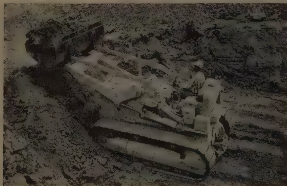
SCOOPING UP a load of dirt right next to the bank, the new Caterpillar No. 6 shovel demonstrates its ease of mobility.
