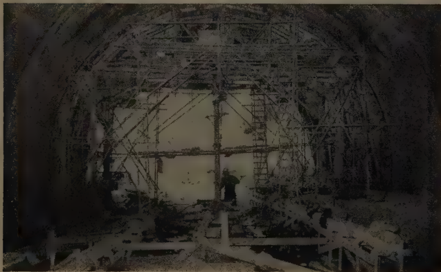
TUNNEL LINING FORM seen inside (left) and out (right). Smooth travel was assured by having concrete arch footings, curbs, and gutters poured before lining was started. Light tubular scaffolding added working space at ends of form for handling bulkhead work and maneuvering concrete pipe and slickline.
