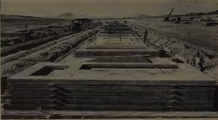
BARRACKS WALLS are stockpiled after casting on floor slab, which isn't big enough to cast all panels at once. Unlike the roof, wall panels come in many varieties, and exceptions exist within each variety.
