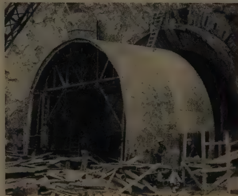
TUNNEL LINING FORM seen inside (left) and out (right). Smooth travel was assured by having concrete arch footings, curbs, and gutters poured before lining was started. Light tubular scaffolding added working space at ends of form for handling bulkhead work and maneuvering concrete pipe and slickline.
