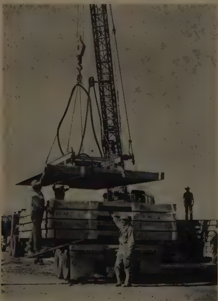
PRODUCTION LINE (top) of steel molds is fitted with re-bars and mesh before casting roof panels. Aggregates are produced locally by contractor, batched in Conveyco-equipped plant in background. The Monster (center) can stack 'em 7-high, using vacuum mats and electric hoists beneath a 12-ft. clearance. Machine can easily be restored to original status. Out of the stockpile, roof panels (left) are handled by vacuum-fitted truck crane. View shows frame for 4 individual lifting mats; also the waffled panel surface created by and of integrally cast ribs.
