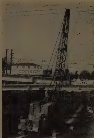
SQUARED AWAY (left) with an 18-ton beam after picking it up from casting area behind crane at right, the two cranes move out together under directions from boss rigger.
