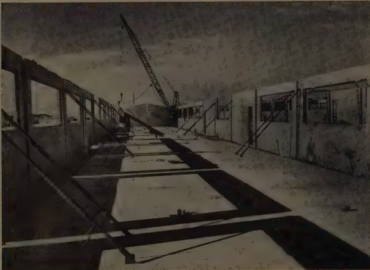
PANELS (above) come before frames on this barracks. Note adjustment on braces used to plumb the wall during erection. Wall panels (below) come in all shapes and sizes, with unsymmetrical openings as shown here.
