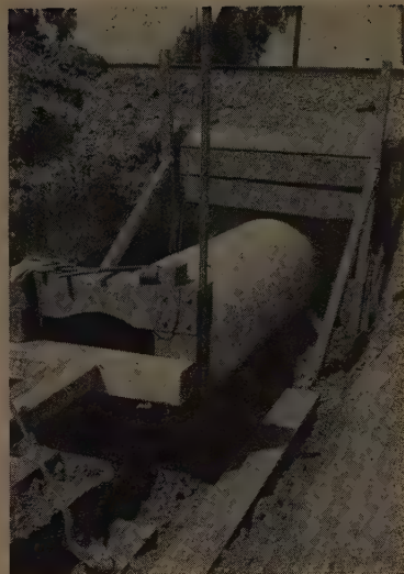
JACKS should have a minimum capacity of 35 tons. Those operated by compressed air have proved effective if a compressor is available on the job. The travel of the jack should be at least 13 in. to allow the use of 12 x 12-in. jacking timbers. At the start of any job the use of lighter and faster jacks may speed the work until resistance builds up.
