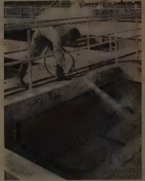
CLEANING dirt, grease, and scum from the sedimentation basins, digester tanks, and building walls at the EBMUD sewage disposal plant is no trick at all with this Malsbury high-pressure movable steam cleaner.
