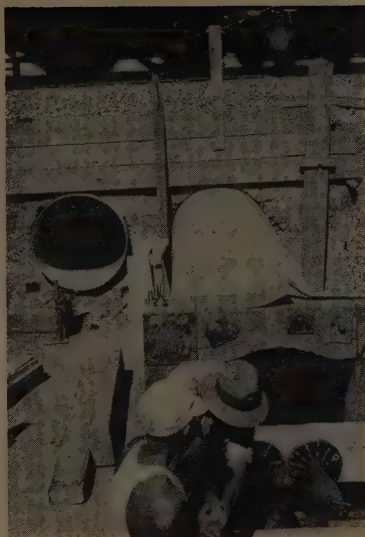
JACKS should have a minimum capacity of 35 tons. Those operated by compressed air have proved effective if a compressor is available on the job. The travel of the jack should be at least 13 in. to allow the use of 12 x 12-in. jacking timbers. At the start of any job the use of lighter and faster jacks may speed the work until resistance builds up.
