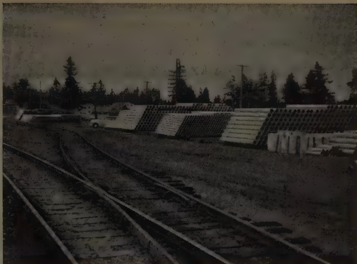
Stock of "Century" Asbestos-Cement Pipe
