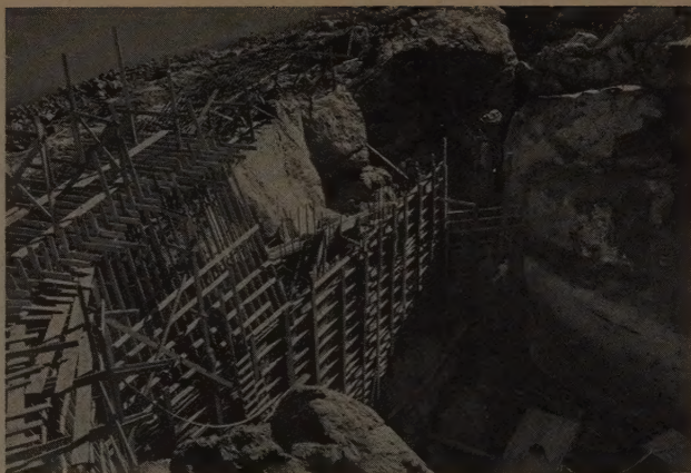
CONSTRUCTION of dam to provide stilling pool: (left) outer face of dam showing reinforcing of the discharge apron; (right) back side of dam showing depth of stilling pool.
