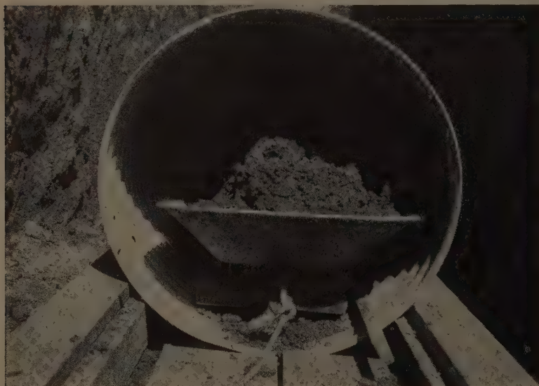
REMOVAL of the excavated material will depend on the size of the culvert being jacked. For pipe that is 48 in. in diameter or larger, a wheelbarrow can be used. For the smaller size pipe, a skip or some type of dolly-mounted dirt box is arranged and handled by rope from the face to the jacking pit. In either case, the loading at the head end is done by one crew member, while another does the actual digging.
