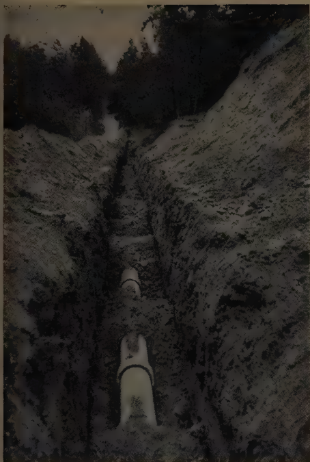
Part of a 13 mile installation of "Century" Asbestos-Cement Pipe, Lakewood Water District, near Tacoma, Washington
