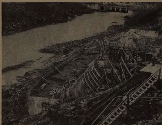
CONSTRUCTION of dam to provide stilling pool: (left) outer face of dam showing reinforcing of the discharge apron; (right) back side of dam showing depth of stilling pool.
