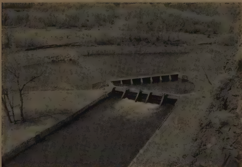
THIS GENERAL VIEW shows the diversion dam, drift guard, sluice gates, and canal headgates of the Rio Grande Canal water regulation system.
