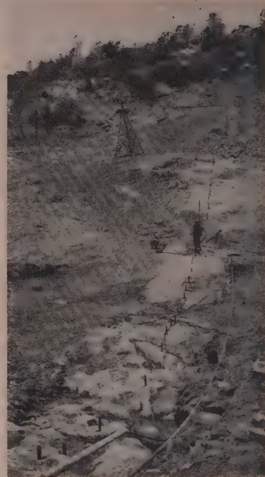
DIAMOND DRILLING and grouting of core trench for main dam was done last July, preceding the 8-month "big push" that has since topped out the structure.
