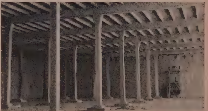
INTERIOR VIEW of completed reservoir shows detail of columns, beams and roof joists. Installed at lower right is a 42-in. butterfly valve at the inlet connection.
