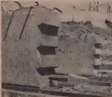
NOTCHED ENDS and dowels were provided at beam ends for connections over columns.
