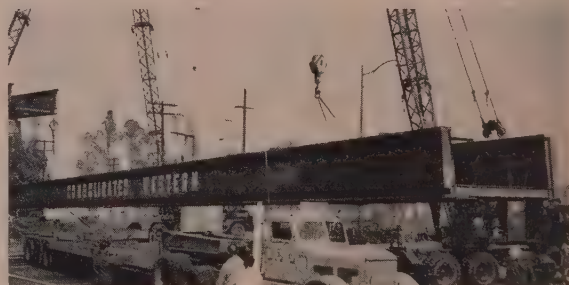
AT SITE. Three cranes slowly maneuver long span into place.
