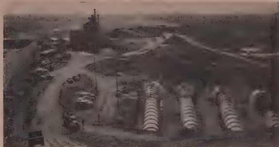
LOOKING DOWNSTREAM on left (U. S.) bank of river: spillway at left, U. S. penstocks in foreground. Single batch plant equipped with four mixers supplies all concrete for the work.
