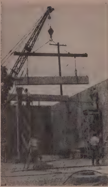
20-TON MOBILE CRANE handled erection of precast columns and beams, delivered to erection site by a lumber carrier.
