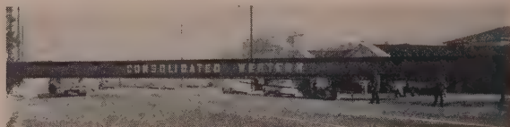
THE START. Leaving manufacturing plant 10 mi. from job.
