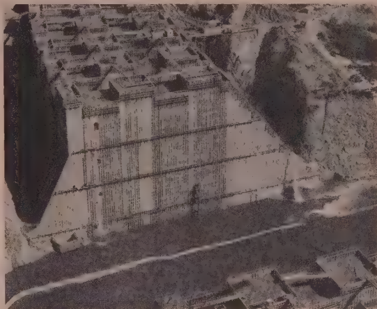
SYSTEM OF BLOCKS formed by longitudinal and transverse construction joints and the vertical keys along one of the transverse joints are shown in construction view at Shasta Dam during 1941.
