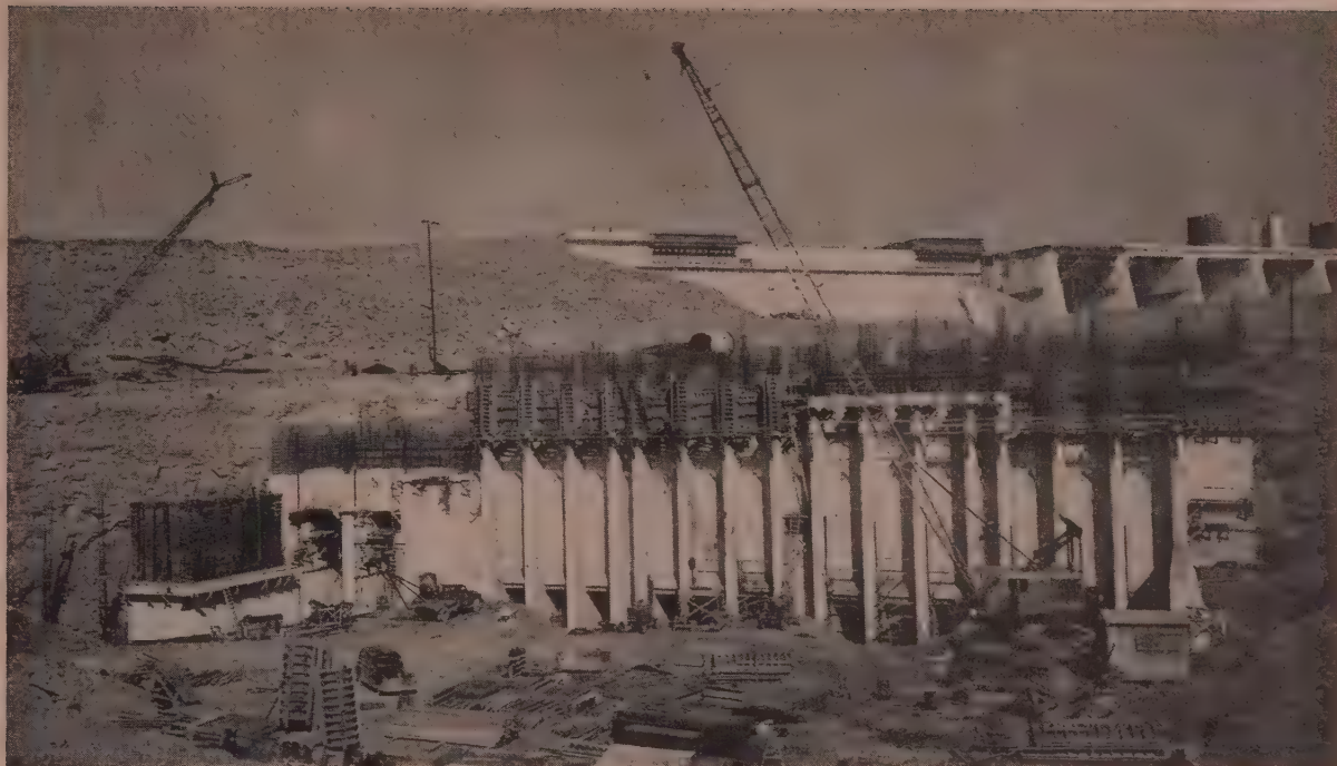
STATESIDE POWERHOUSE is virtual twin of Mexican facility. Intake structures vary, U. S. penstocks leading from concrete dam section seen in background adjacent to spillway structure. This view shows progress in December 1952, with entire project three-quarters completed.
