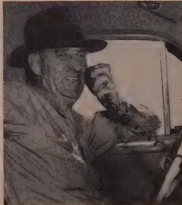
TUCKER kept things moving and under control by shortwave. Job had 10 General Electric mobile units, plus sets in the office and shop.
