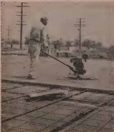
ROOF SLAB, placed on steel pan forms, was machine trowelled and then sprayed with membrane curing compound.
