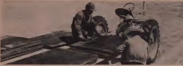
ASPHALT PLANK is provided in sheets 3 ft. wide in any length up to 12 ft.
