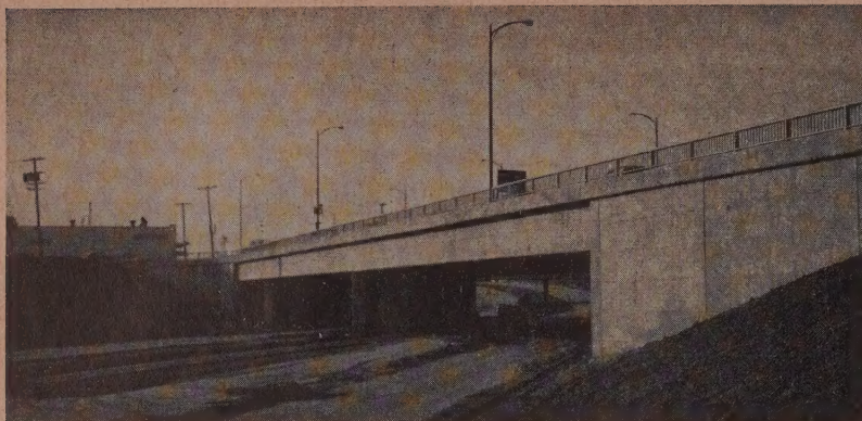
LONGEST of their type yet built in the Los Angeles area, these 146-ft. concrete box girder spans (left) carry Olympic Boulevard across the Santa Ana Freeway.
