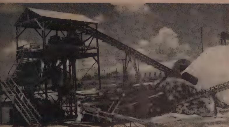
MODERN STONE-SAND PLANT, showing the relatively standard features of surge storage silo, raw feed conveyor, screening structure, rod mill, wet classifier, classifier waste launder, and finished sand conveyor.
