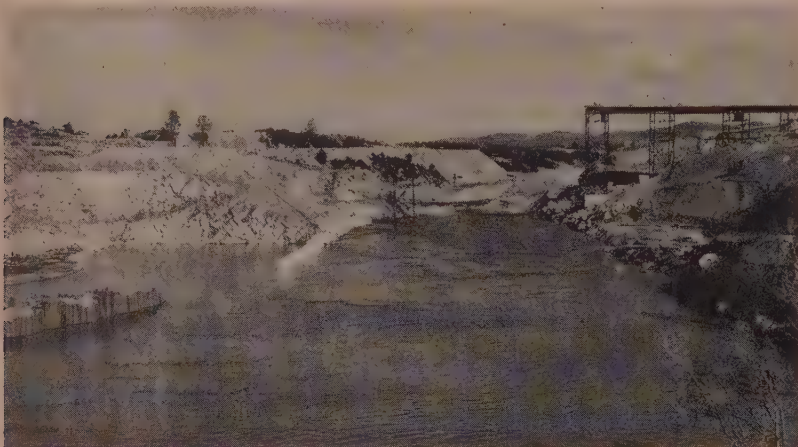
THE SEASONS are strikingly illustrated in these shots of the American River at Folsom Dam. Current photo (above) views site from a point below the powerhouse right after failure of the upstream cofferdam on January 9. Two trestle bents were lost along with five cells of powerhouse cofferdam at left. Photo of excavation last October (below) includes cofferdam in background for comparison.
