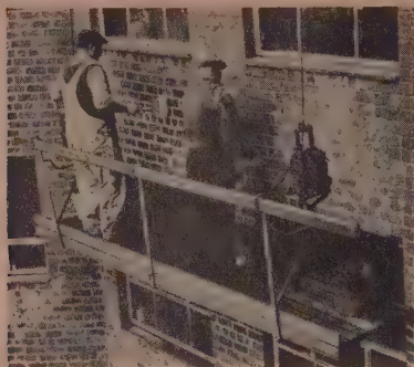
LIGHT-DUTY SWINGING scaffold must not be overworked. It is intended mostly for maintenance work by few men with hand tools—glazing, pointing up masonry, painting, etc.
