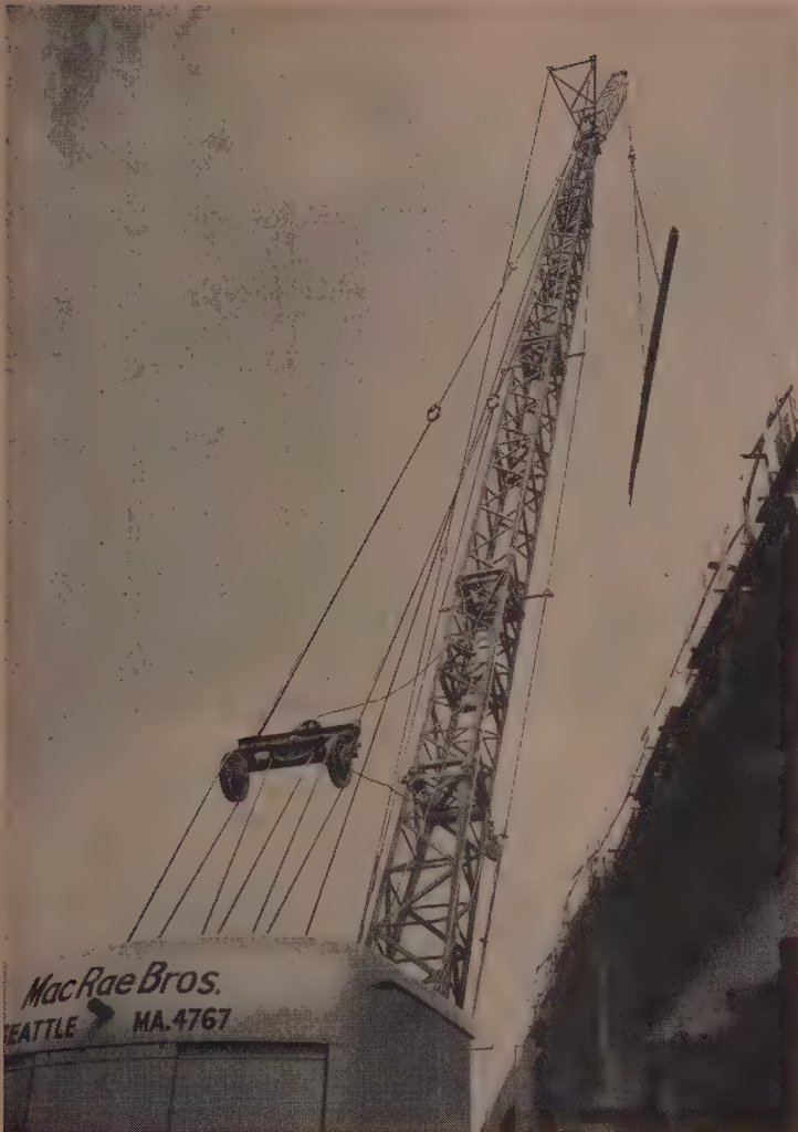
Load lines and boom lines on this 20-ton truck crane show some of the work Tiger Brand Wire Rope does for MacRae Bros. Contractors, Seattle. Rugged with 110' of "stick", the crane is moving steel "re-bars" onto Seattle's Alaskan Way Viaduct. Despite steady work on all types of jobs, its load lines last over a year apiece, boom lines about 6 weeks each under constant booming.
