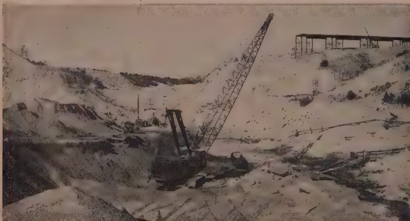
THE SEASONS are strikingly illustrated in these shots of the American River at Folsom Dam. Current photo (above) views site from a point below the powerhouse right after failure of the upstream cofferdam on January 9. Two trestle bents were lost along with five cells of powerhouse cofferdam at left. Photo of excavation last October (below) includes cofferdam in background for comparison.
