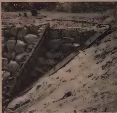
DETAIL AT ABUTMENT shows steel in position, form walers bolted to extensions of anchorage rods drilled into rock.
