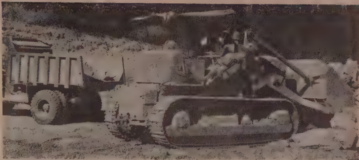
IN-PLACE YARDAGE (left), a hard blue limestone, was drilled on 5-ft. centers, wore out tungsten carbide drill bits in 80 ft. or less.
