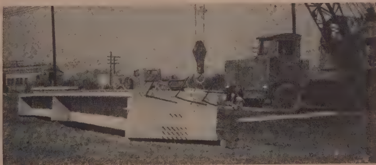
T-SLAB (below) for roof of Spitzer Electric Co. building is 39 ft. long. The units are getting bigger.
