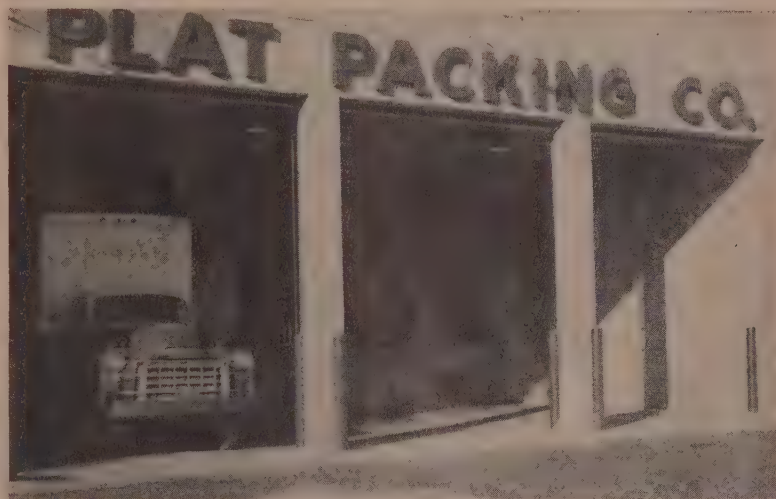
CLEAR AND OPEN dock area (above) for loading and unloading trucks was achieved by use of 41 ft., 6-in. prestressed beams.
