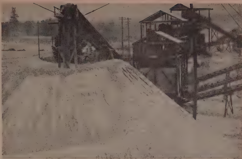
SEGREGATION IS APPARENT in this conical surge storage pile of feed material for a stone-sand plant.
