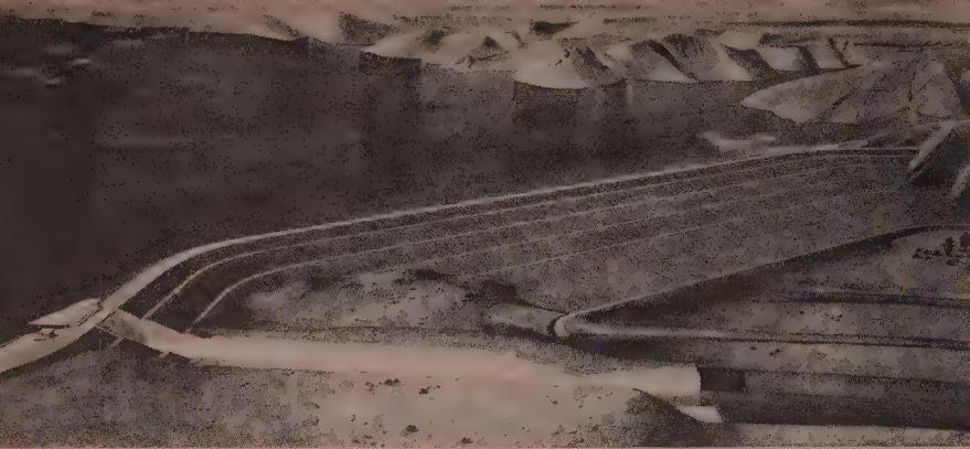
TIBER DAM , an upstream unit of the Missouri Basin project in Montana, got under way in September. Main dam will be 205 ft. high and 4,300 ft. long, accompanied by an earthen dike 17,000 ft. long. Location is Lower Marias River, near Chester.
