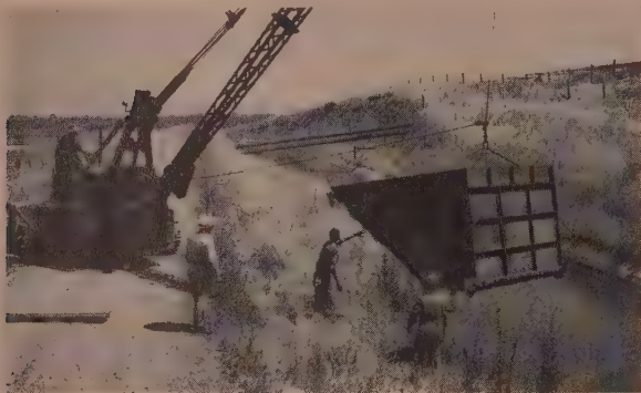
EASY TO INSTALL—Crane lowers cofferdam into position.
