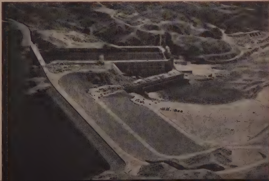
DAVIS DAM, on the Colorado River between Nevada and Arizona, was the scene of dedication ceremonies in December that marked virtual completion of the dam and its works. Some stilling basin construction remains, under contract to Grafe-Callahan Construction Co.
