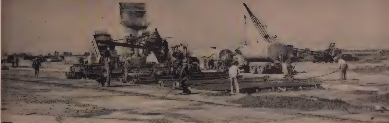
AIRPORT PAVING constitutes the largest volume of military work handled in the Southwest by the Corps of Engineers. Pictured are operations of Ball & Simpson, H. Earl Parker, Harms Bros., and Fred J. Early at Castle Air Force Base.
