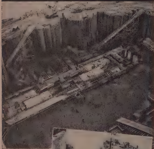
A McKiernan-Terry Pile Hammer helps build a cofferdam for the large Philip Sporn power plant on the left bank of the Ohio River near New Haven, W. Va.
