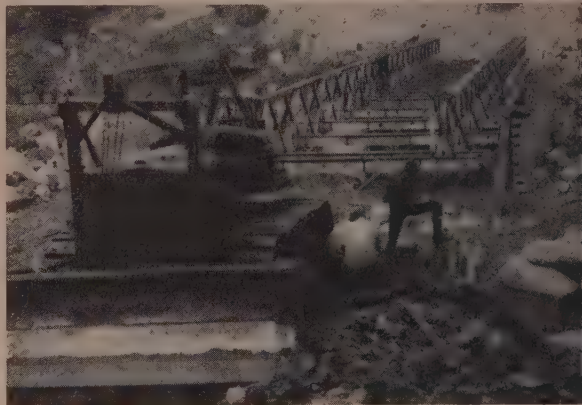
TRACTOR PULLS 80-ft. Bailey-type bridge and 50-ft. launching nose, all on rollers, across the gap. Bridge has 12 ft., 4 in. roadway and a safe capacity rating of 53 tons.
