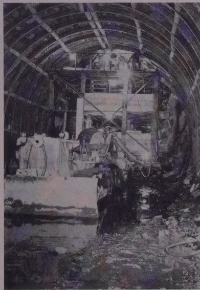
DRILLS are mounted on a truck frame moved by tractor. This outfit alternates in the two tunnels on a schedule that gives a complete round every 12 hours.
