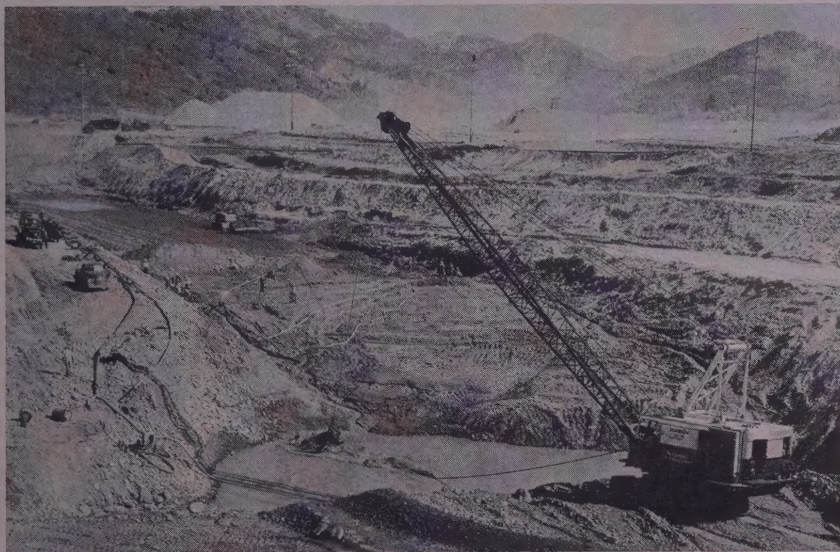
UPSTREAM CUTOFF excavation was complicated by a "glory hole" that tied up a dragline for an extra month while embankment placement was carried out on both sides.
