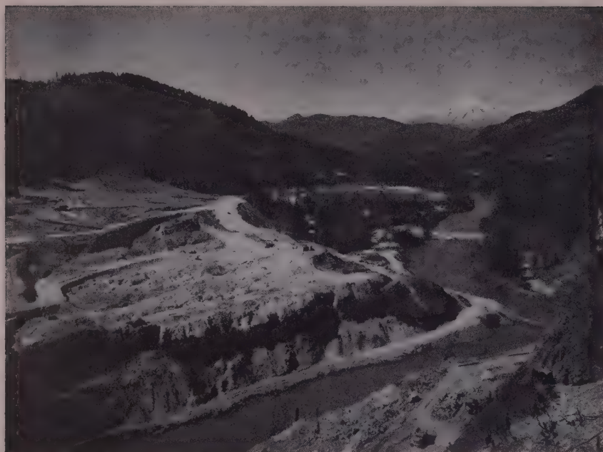
START —In July 1951 the site showed fast work in clearing and stripping to bedrock over much of the dam area. The diversion tunnel extends under the far bank of the Lewis River, with Mt. St. Helens in the distance.
