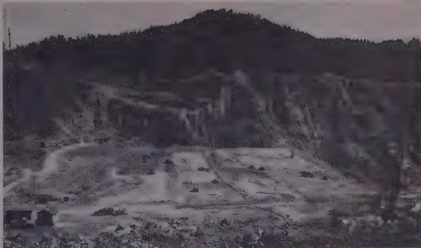
PROGRESS in placing earthfill reached a maximum on June 17, 1952 when the crews and equipment of Morrison-Knudsen put in 40,312 cu. yd. (24 hours) or at a rate of a truck dumping every 34 sec. around the clock.
