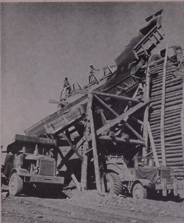
COMMON EXCAVATION out of stockpile was first run over a 5-in. grizzly, during this season, to secure material for Zone 2 (passing) and Zone 3 (scalped). Borrow pit yardage next year won't need this treatment.
