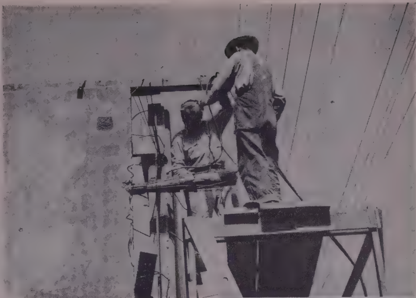
JACKING EQUIPMENT in position for applying a 135,000 psi. tension in the wires which extend through the entire length of the 100-ft. wall.
