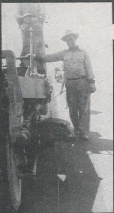
1—Cement-treated base and the plant-mix surfacing were compacted with the new type Buffalo-Springfield pad roller.
