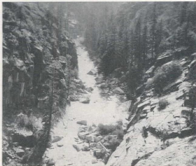
RUGGED SITE for Donnells Dam where a constant angle concrete arch will be fitted between granite walls. Height will be 288 ft. above streambed; concrete quantity will be almost 250,000 cu. yd.
