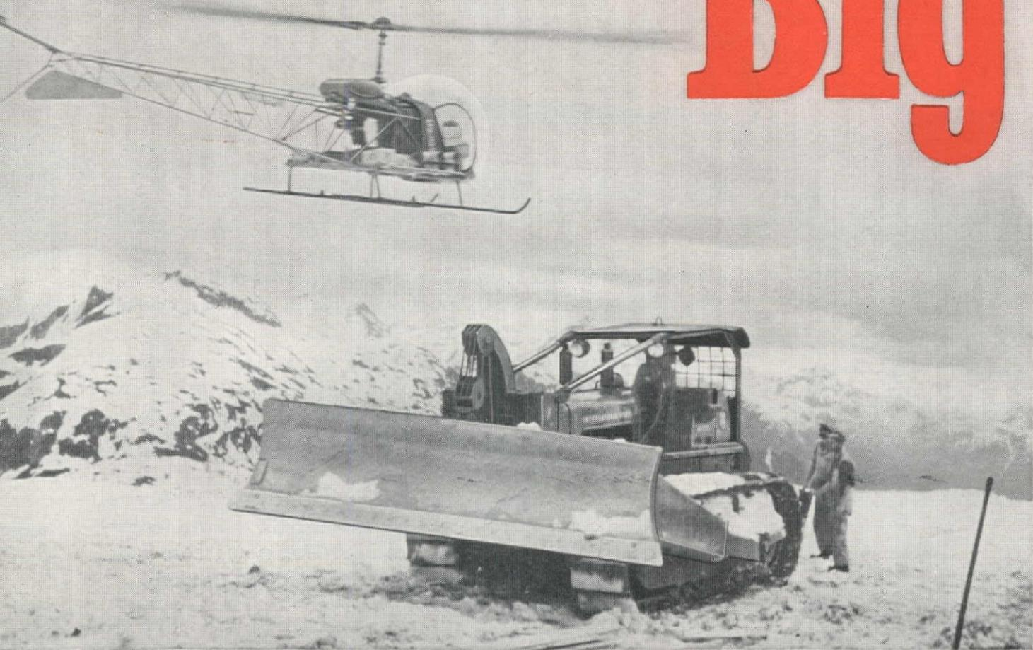
**1 RAISING KENNEY DAM** to fill the Grand Canyon of the Nchako River, workers sluice down some of the 3.8 million cubic yards of earth and rock it will eventually contain. Dam will form a reservoir with twice the capacity of Grand Coulee. TD-24 in foreground strips blasted rock from canyon wall abutment.
