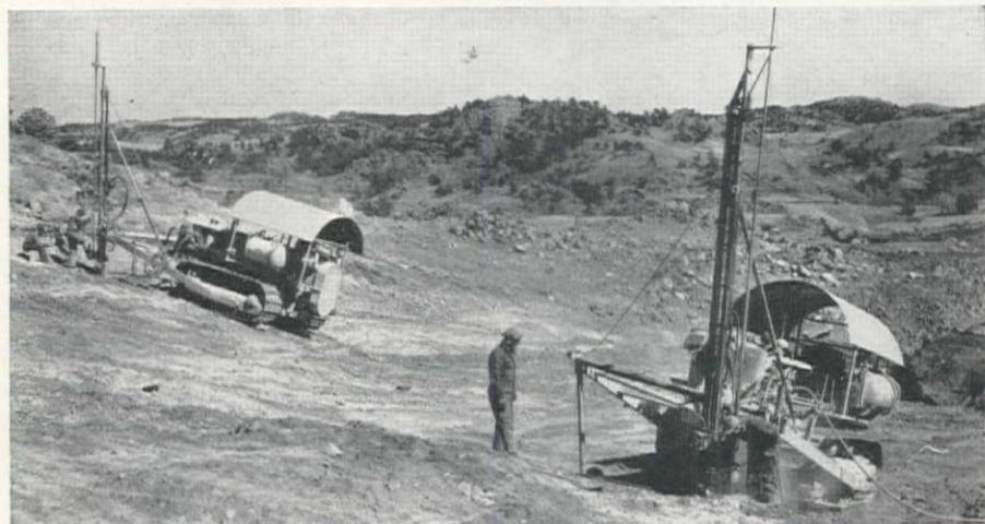
WEST END of the line cuts through granite, and rock work is scheduled for completion in June 1953. Typical rigs are Worthington drills and compressors mounted on Caterpillar D8's for mobility. About 3,000,000 cu. yd. of rock will be moved. Blasted rock is handled by shovel and trucks (see below).
