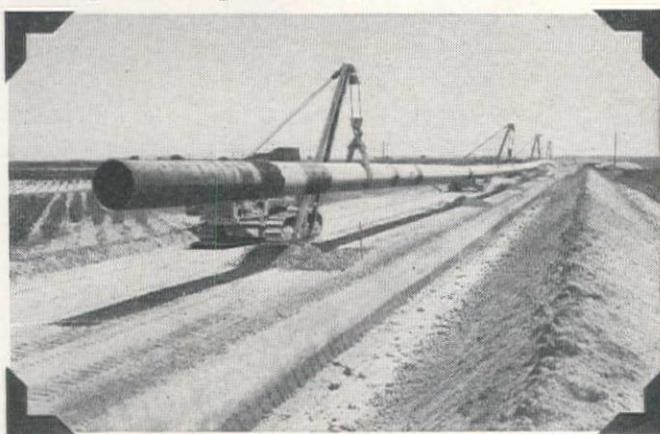
DIESELS OF ALL SIZES up to D-13000 models were on the job. Here four Caterpillar D-8's "walk" a pipe section into place along side the trench. There's an RPM DELO Lubricating Oil for every diesel.
