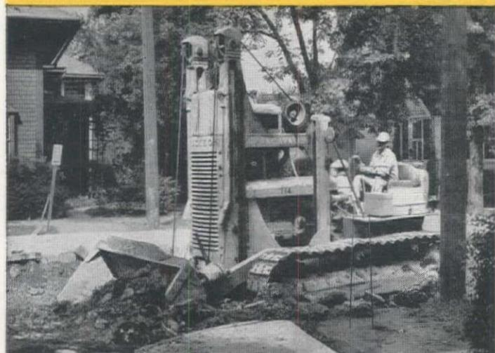
Paul N. Greene Co.'s T6 is here shown at work in Fort Wayne, removing old concrete and brick paving, crossties and other debris. The powerful lift and drawbar push tears up the old surfacing and puts a heaped 1½ yds. in the bucket each pass.
