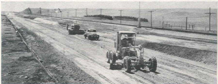
**GRADING** was relatively light where the line leaves Cheyenne on the eastern end and much was handled by elevating grader, with Caterpillar motor graders used for finishing. Side slopes of fills are not receiving special protection against erosion because the rainfall is light in the area.
