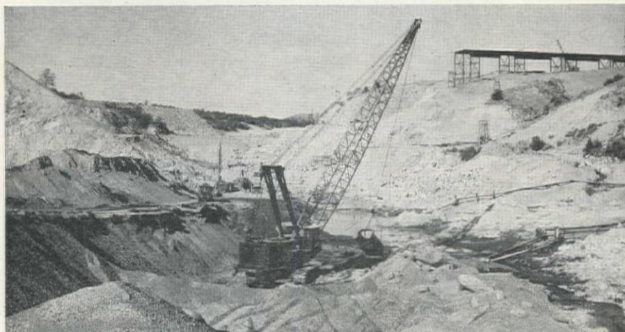
month to 350,000 cu. yd. Gravel will remain the biggest item, for hydraulic mining debris in the American River channel in this immediate area totals over 2,300,000 cu. yd. And it all has to come out during dam and tailrace channel excavation under the prime contract.
