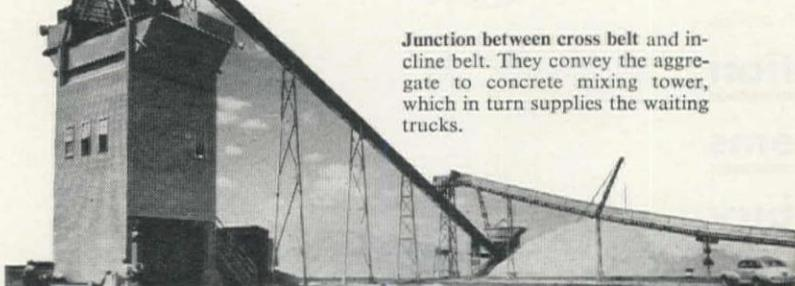
In a new concrete mix plant, original plans called for the installation of a 5-ply, 36 oz. duck conveyor belt to handle the aggregates. But United States Rubber Company engineers pointed out that their 4-ply, 42 oz. duck belt would not only cost less, but would be more flexible crosswise to trough, would train more easily and provide high-tensile strength as well. This 1,275-foot, 4-ply U.S. Giant Conveyor Belt was installed. It travels 300' per minute and delivers 294 tons per hour.
