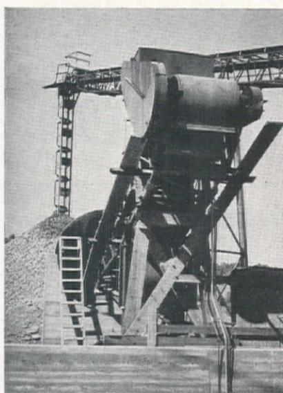
sand plant surge, all smaller than  $\frac{3}{4}$  in. Again, as in the preceding operations, there are two double-deck screens handling the screening. These are 4M and 8M, the former scalping all  $-\frac{3}{4} + 4$ M for conveyance to a stockpile of pea gravel. This stockpile has reclaiming facilities such as have been described for the coarse aggregate.
