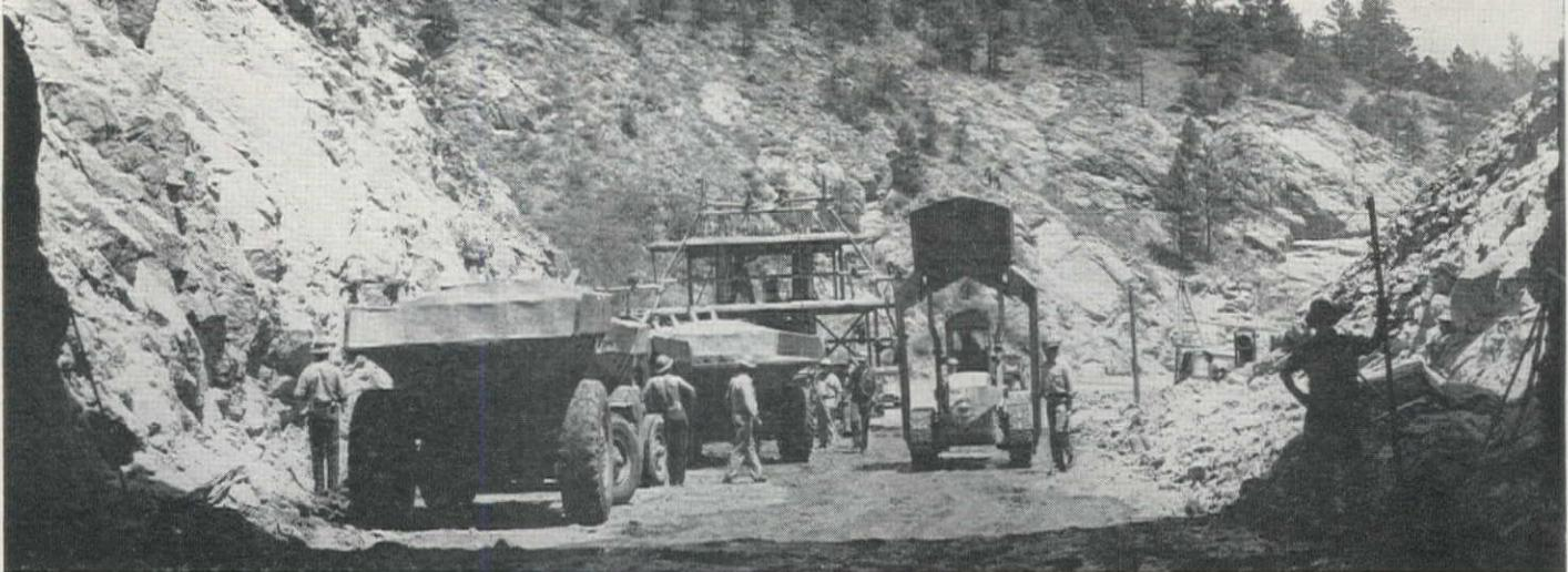
*Saving 1,600 ft. of distance and many thousands of yards of solid rock excavation, this 340-ft. two-lane tunnel was the solution to a tough relocation job in the mountains west of Boulder*
