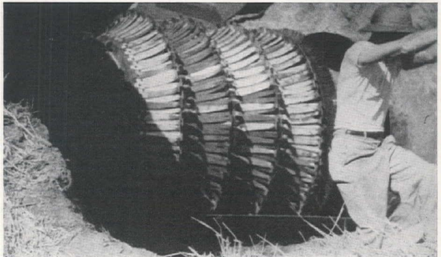
CLEANING TOOL being inserted into the 66-in. diameter steel pipe through a hole produced by cutting out a 7-ft. top section.
