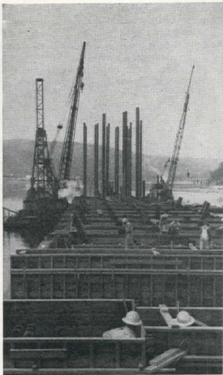
CONCRETE CAPS are formed close behind driving operation. Cluster of tall piles offshore is scene of production welding as many second sections are added to first 120-ft. length.
