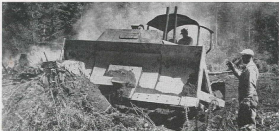
ABOVE: The Skinner gets an assist in lining up his quarry as the Scalzo stump splitter takes on a reluctant stump. LEFT: Bob Scalzo appraises the device that substituted for 5,000 lb. of blasting powder on one of his company's jobs.
