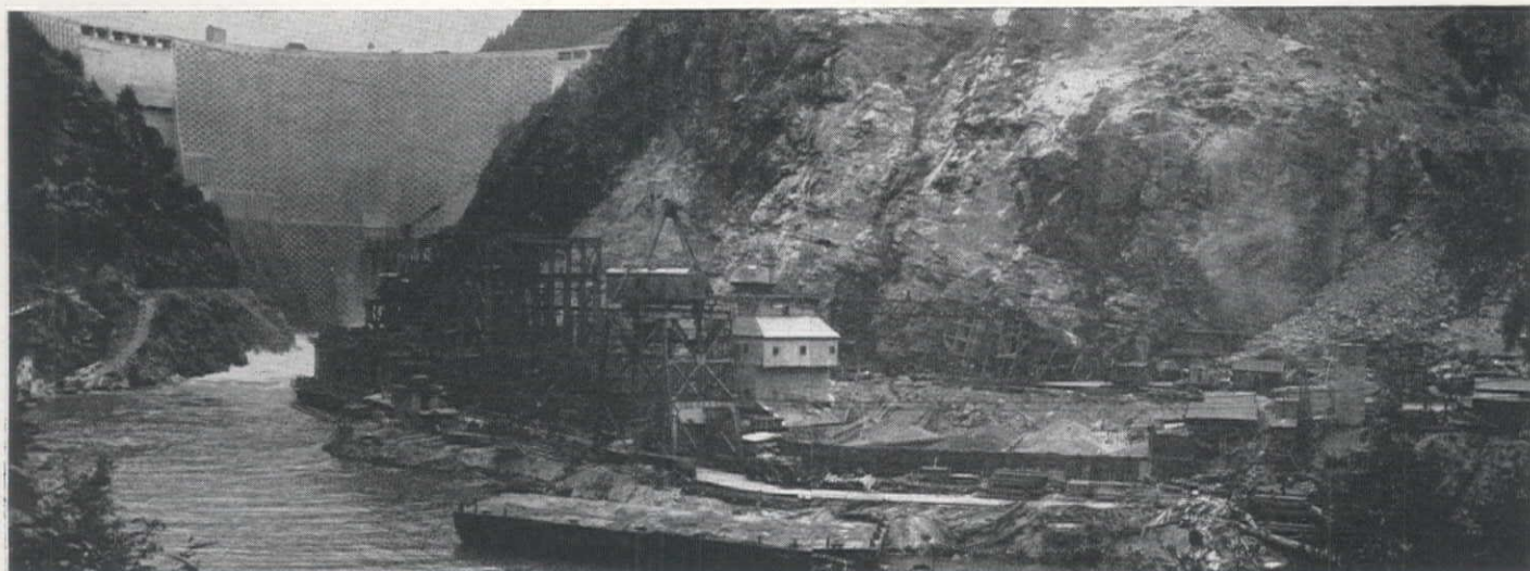
THE WHOLE PROJECT is parked on a narrow bench in the Skagit River gorge. Two gantry cranes ride ways in foreground to service powerhouse construction and handle concrete batching. Bifurcation forms are being built against cliff at right center. Barges can proceed to toe of dam for highline handling of material needed there.
