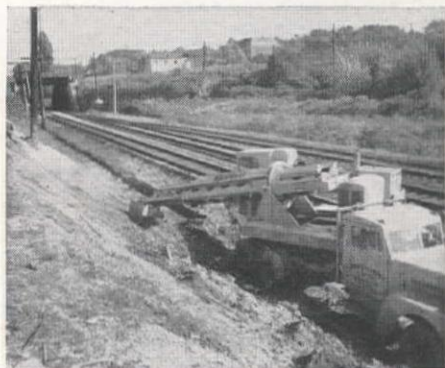
Hydraulic arm-action boom tilts bucket to work at any angle.
