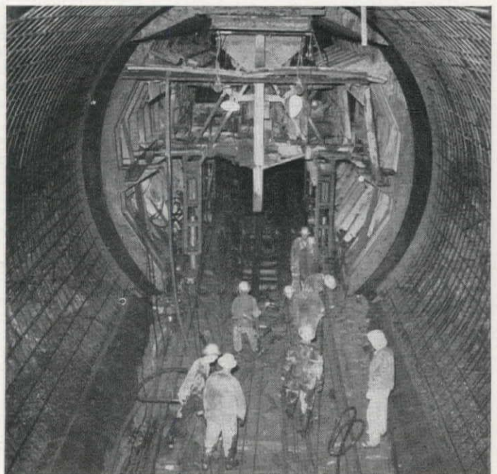
COLLAPSIBLE form shaped 25 ft. of lining in a single pour in upper part of Tunnel 2. Concrete was boosted through two Pumpcretes to reach work.
