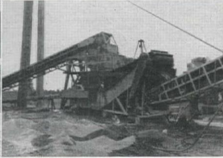
SAND WASHER agitates fines washed from pit feed, skims off mason sand to conveyor at right. Plant currently produces 5 aggregate sizes.
