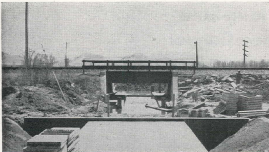
A COMPLICATION was to get the drainage through an existing railroad structure (shown in background). It was deepened 5 ft. by building a concrete-lined ditch in the bottom. End of box culvert under new section of highway appears in the foreground.
