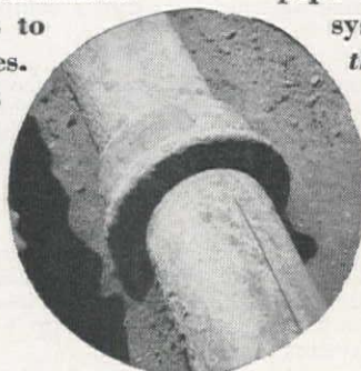
This cast iron water main installed in Richmond, Virginia, 120 years ago, is still in service. Over 35 other cities have century-old cast iron mains in service.
