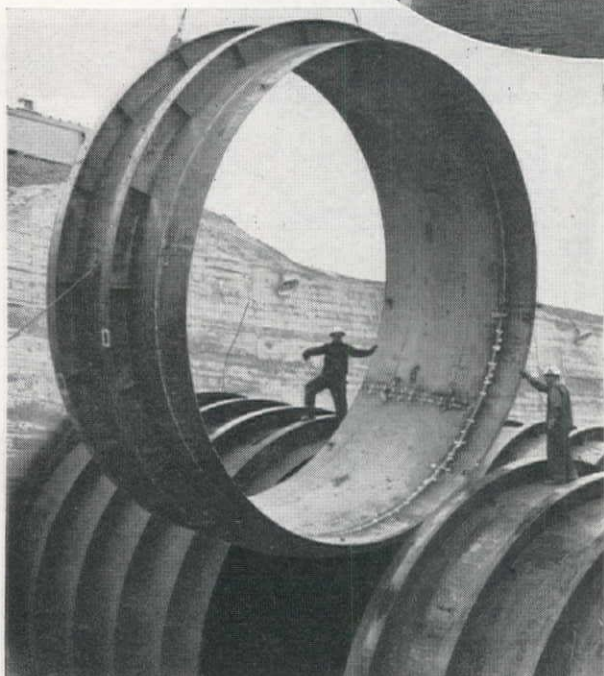
Above: Closing section of Horton steel penstock being lowered in position at the Snake River dam site.
