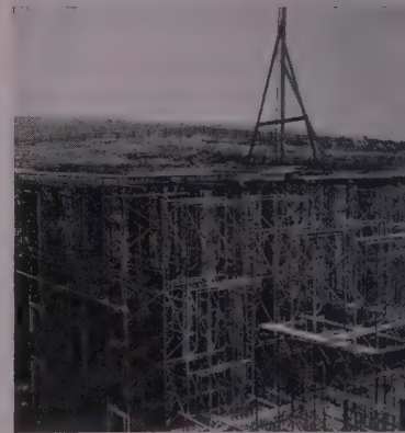
FOUR-HIGH steel scaffold system supports forms for concrete slab roof 6 in. thick.
