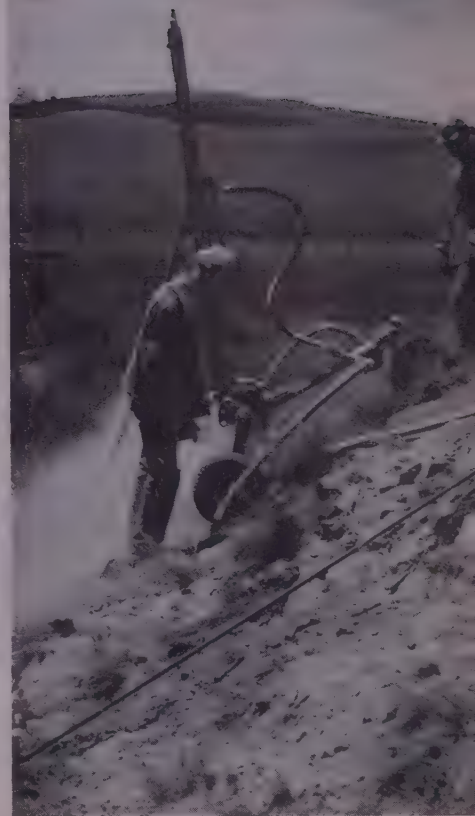
ROCK WORK on Montana highway cuts puts a wagon drill on a tough angle.
