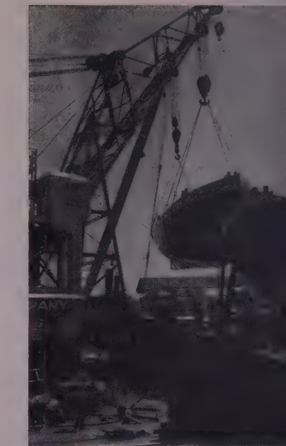
ABOVE—Prior to backing derrick barges away from dock to provide water area for floating steel hull craft being launched was aligned with edge of dock.
