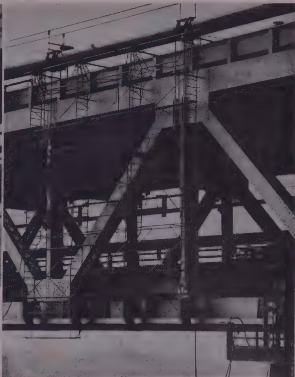
TRAVELING BRIDGE (above), used for painting the lower deck floor on the East Bay side, is 6 ft. wide by 77 ft. long, has open steel flooring, and is suspended from two lines and moved by taking up on one and slacking off the other.
