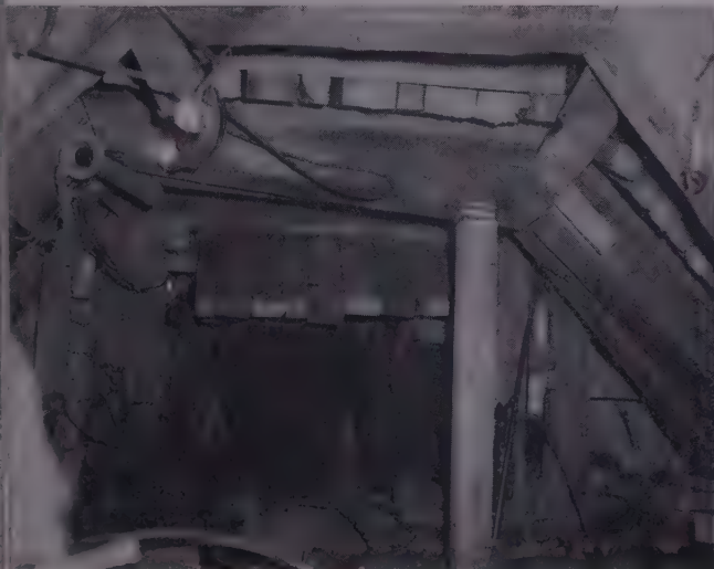
ENTER DRIFT penetrating plug in Tunnel 5, showing heavily timbered heading 230 ft. from the east portal on August 5, with the face 50 ft. into the caved material.
