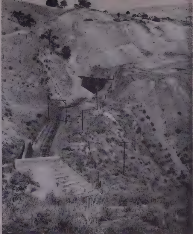
RIGHT —Daylighting of Tunnel 3 began two days after the earthquake. On the third day, as shown, a dozen earthmoving rigs attack the slope, which covers 230 ft. of the east end of the tunnel. The bow in the track is 22 ft. off line.
