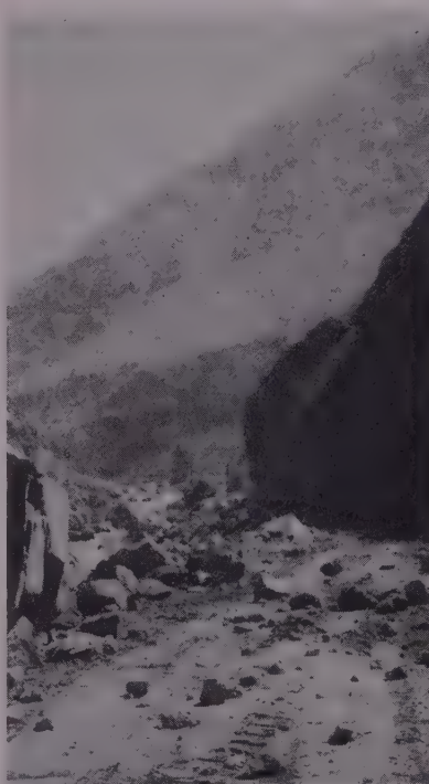
KERN CANYON road, State Highway 178 leading to Isabella Dam, remained closed long after quake as rain of boulders continued. Repairs here will be expensive, covering many miles involving rock slides.
