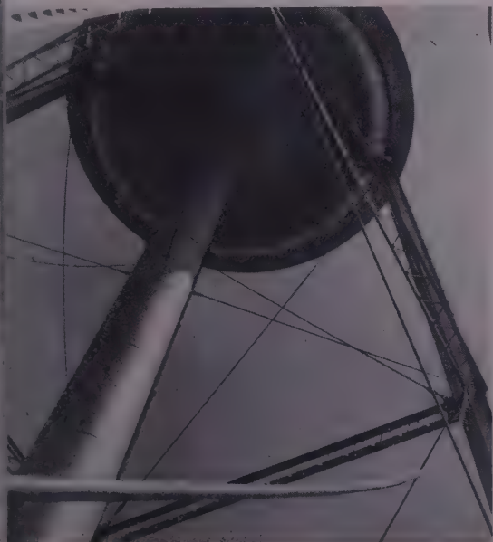
ELEVATED WATER TANK at Arvin (left) is of 75,000-gal. capacity. Designed only for wind loads, it survived, but with much stretching of tie rods (note sag) and twisting of columns. Repair will see heavier members and details used.
