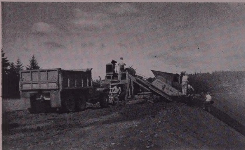
ARRIVING AT THE TOP of the slope, the paver was pulled up onto a timber skid-rig developed and built by the contractor. The skid was then pulled forward by truck for the width of the paved strip. The winch in the skid then lowered the paver down to the bottom of the slope.
