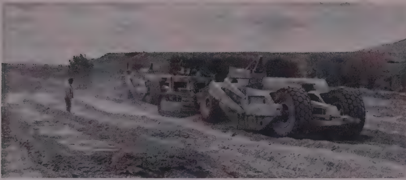
IN THE BORROW PIT, two rigs load for hauling to the fill. Much of this yardage went into embankment built over deep marsh.
