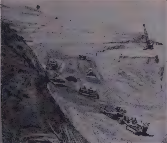
RIGHT —Daylighting of Tunnel 3 began two days after the earthquake. On the third day, as shown, a dozen earthmoving rigs attack the slope, which covers 230 ft. of the east end of the tunnel. The bow in the track is 22 ft. off line.
