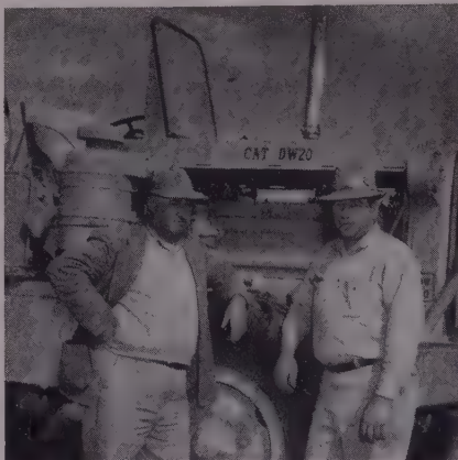
John Huggard , supt., left, and Don K. Kellogg , equip. supt. for M. M. Sundt Construction Co. on runway construction at Davis-Monthan Air Force Base , near Tucson, Ariz.
