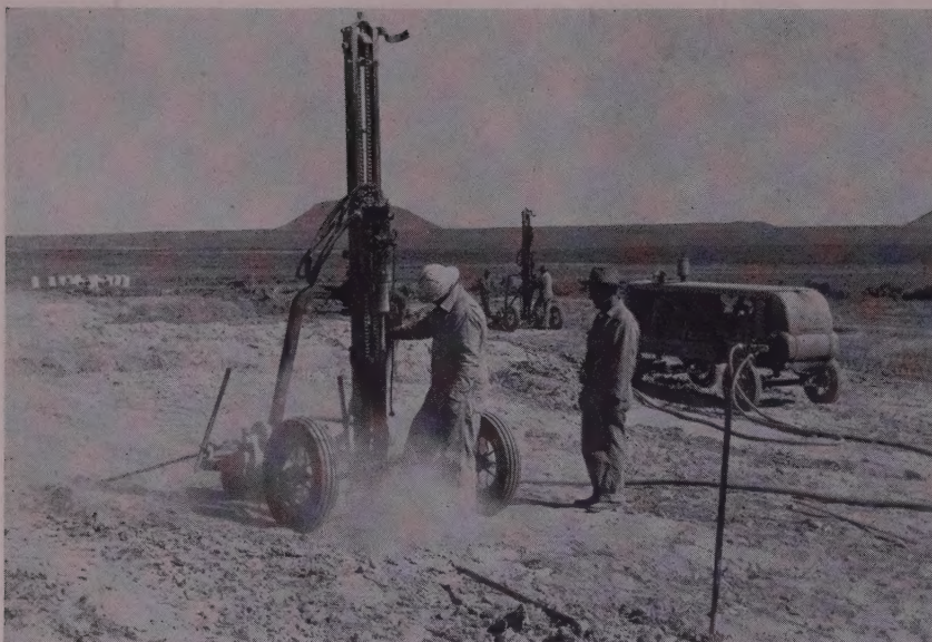
LEFT—Wagon drills set up a hole pattern of a uniform 5 ft. Despite abrasive seamed rock, each of three drills on the job is averaging up to 750 ft. of hole each 8-hr. shift.
