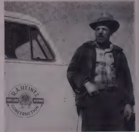
J. H. Wright is superintendent for R. A. Heintz Construction Co. on levee construction job near Richland, Wash.
