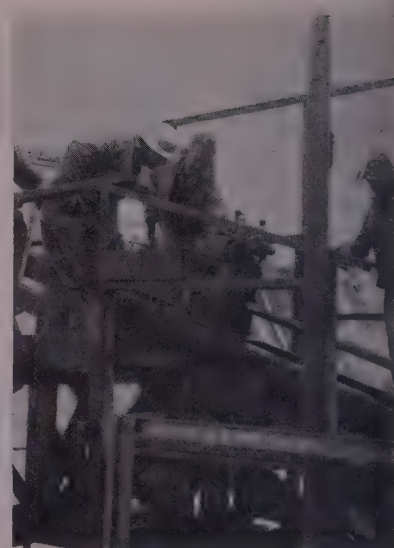
LEFT —Compact rig lies in framework and scaffolding built around it for drydock work. Gasoline engine and hydraulic pumps are seen at bottom of dock, connected to drill only by hose. Hand winches and cables were used to raise and lower drill between work locations. Framework was anchored against effects of drill thrust by bracket and stud in foreground.
