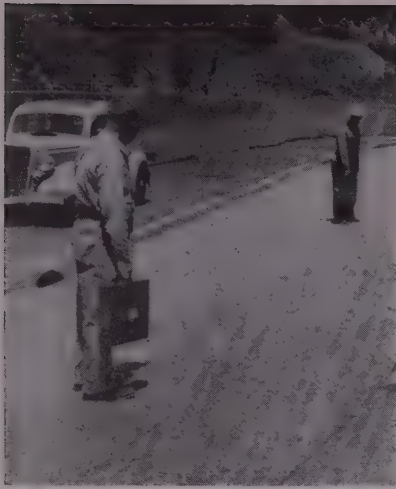
SEARCHING with a 2-part electronic finder that reacts to electro-magnetic field of pipe, operators maintain a 30-ft. spacing.
