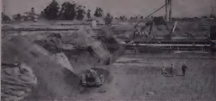
SPREADING AND COMPACTING crushed rock base course, small Cat stayed ahead of concrete operations at east end of plant. Depression in subgrade (rodman) is for sump installation. Excavated avenues at left are for stack foundations.
