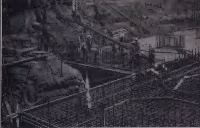
ABOVE: Four vibrators and a 16-man crew worked the concrete into place in the maze of reinforcing that runs through the 5-ft. mat. Wellpoints (left) skirted close to the excavation, drawing the water table down 11 ft.
