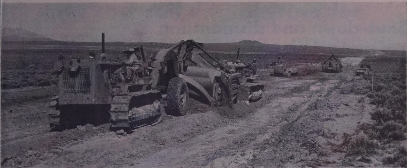
SCRAPERS are being used profitably on hauls of from 800 to 1,300 ft., by making sure, with pushers, that heaping loads are taken up with each pass. Double set of sheepfoot rollers can be seen in the background.
