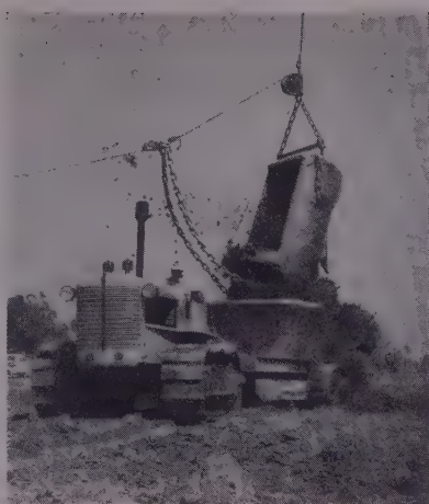
FED BY a 2½-yd. dragline, only these Athey trailers could navigate in waterfront mud until spring came to the project in mid-April.
