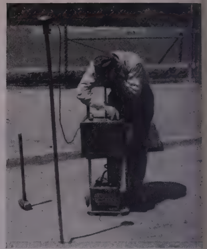
SOUNDING is taken by connecting detector to rod driven down on water main. Greatest noise level is found at leak source.
