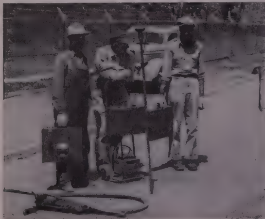
SAN FRANCISCO crew operates from compressor truck, does its own drilling for taking soundings. Hand truck eases reconnaissance and detection problem on city's many hills.
