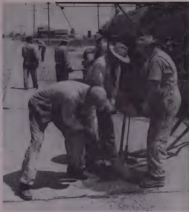
QUICK WORK is necessary to place spud with back surge of asphalt when injection nozzle is removed. Working ahead of crew, laborer swabs pavement around holes with water to break bond of spilled asphalt.
