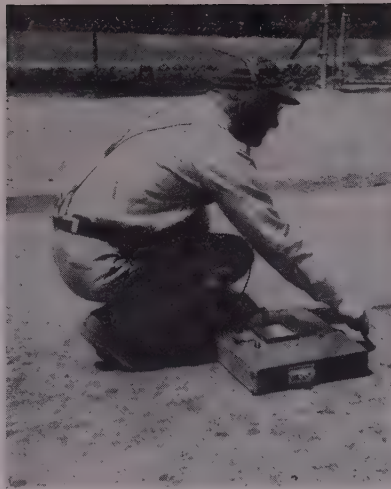
TRACING exact alignment of pipe, the pavement is marked at intervals to establish sounding points for detector.
