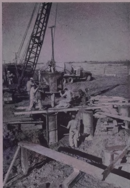
SPEEDING check construction by use of portable steel forms. Concrete is placed in form as it hangs from horizontal steel beams supported by timber cribbing.
