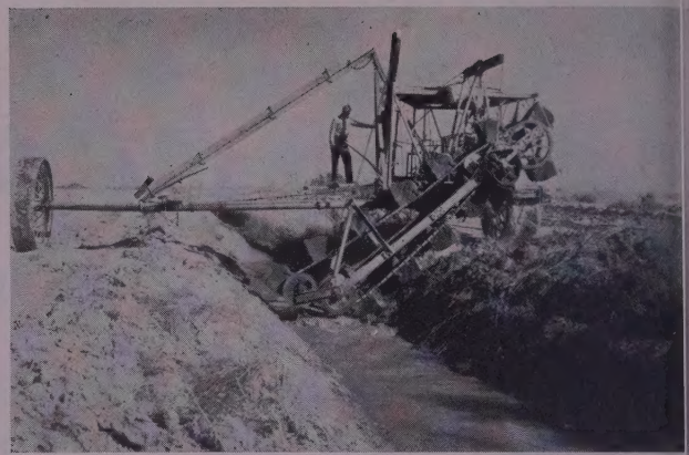
IN DITCH MAINTENANCE a Ruth bucketline dredge is used to deep and clean ditch bottoms. Recently, mule pulled tow cable out snubbing was replaced by a small tractor.
