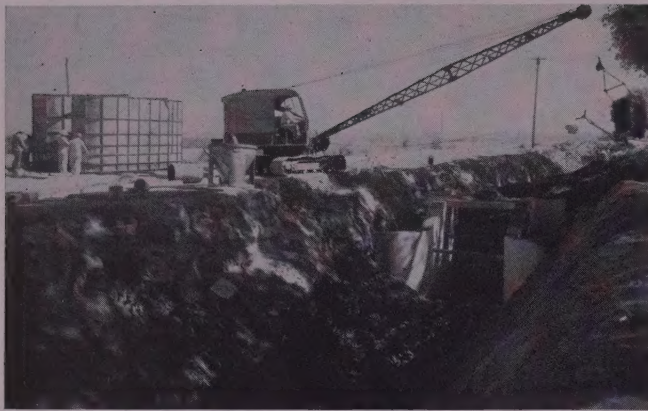
AS DRAGLINE BACKFILLS around completed check, workmen re-assemble steel form. Thus, time is saved at the next job location. Form shown here is 10 ft. high and 20 ft. long.
