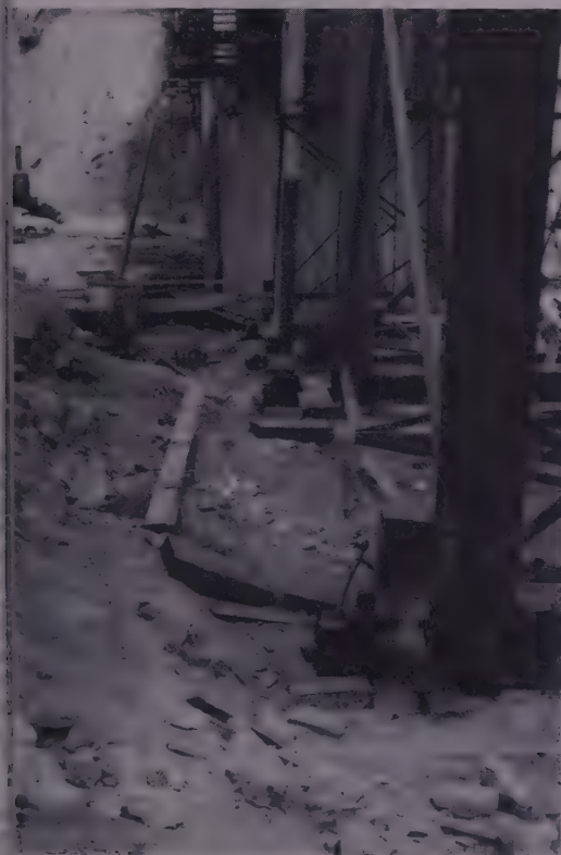
BOXES welded to column legs (view at left) provided bearing for 50-ton hydraulic jacks. These relieved screw jacks for easier lowering of falsework. Placed during the move in the manner pictured, they decreased friction for each increment of falsework motion along skids.
