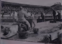
Whiteman Power Buggy on bridge section of New Jersey Turnpike.
