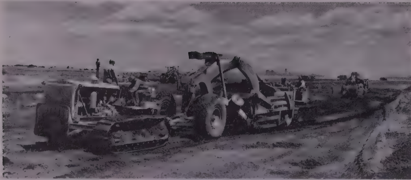
STRIPPING of unstable material from runway area preceded placement and compaction of imported borrow. Work covered 213 acres and involved 500,000 cu. yd. of material.
