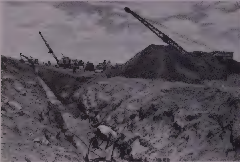
MAN-MADE DRAINAGE establishes pattern where none existed before. Major item was installation of nearly 25,000 lin. ft. of 12- to 42-in. diam. reinforced concrete pipe.
