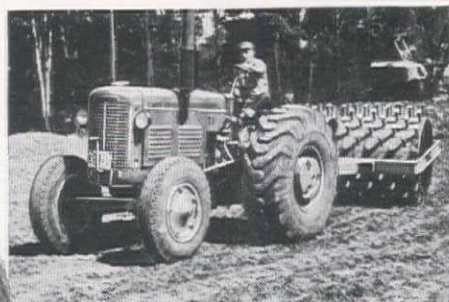
Sure-footed traction of the "LAI" Tractor pulls sheepfoot roller preparing grade for new paving of Highway 6 at a relocation in New Jersey.
