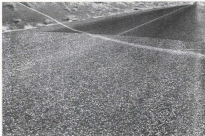
WASHINGTON —A light surface treatment applied to U. S. 10 last year. This was the second seal coat applied since the highway was built in 1933. The route carries the bulk of cross-state car and truck traffic. Detail of texture (right) shows cover of crushed gravel in foreground and crushed ledge rock in background.
