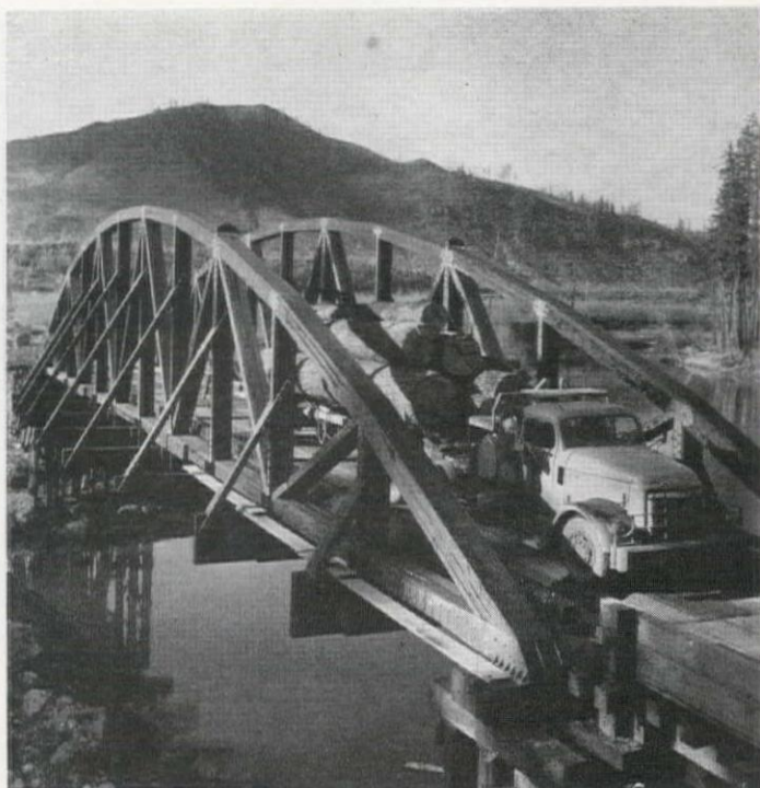
TYPICAL LOAD on the completed bridge. In addition to gross loads of 100 tons, bridge was designed to carry heavily concentrated loads induced by 70-ton track and wheel-mounted loaders used by logging company.
