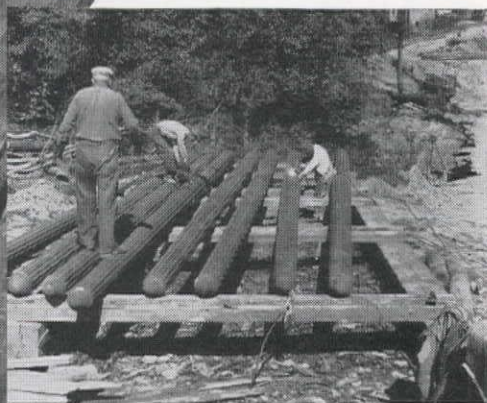
Above: Speedy nesting and welding operations on an assembly rack in the field. Tailoring piles to the required length, on the job, minimizes cut-off waste.
