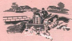
Backfilling foundations
