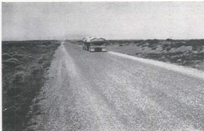
WASHINGTON —A light surface treatment applied to U. S. 10 last year. This was the second seal coat applied since the highway was built in 1933. The route carries the bulk of cross-state car and truck traffic. Detail of texture (right) shows cover of crushed gravel in foreground and crushed ledge rock in background.
