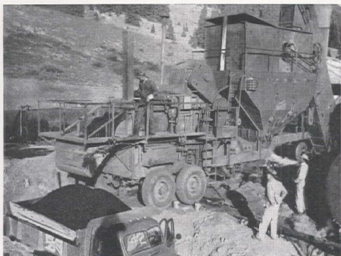
TODAY, modern plant-mix pavement is the standard on the main highways of the Mountain States with continuous plants (left) getting increased recognition and lay-down machines (right) completing the process.
