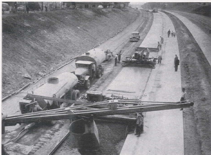
UNDER CRITICAL observation by local interests (under boom at right of screed), freeway construction employs extensive train of equipment. Specially-built tank trailer is towed by paver, supplied by tank truck.
