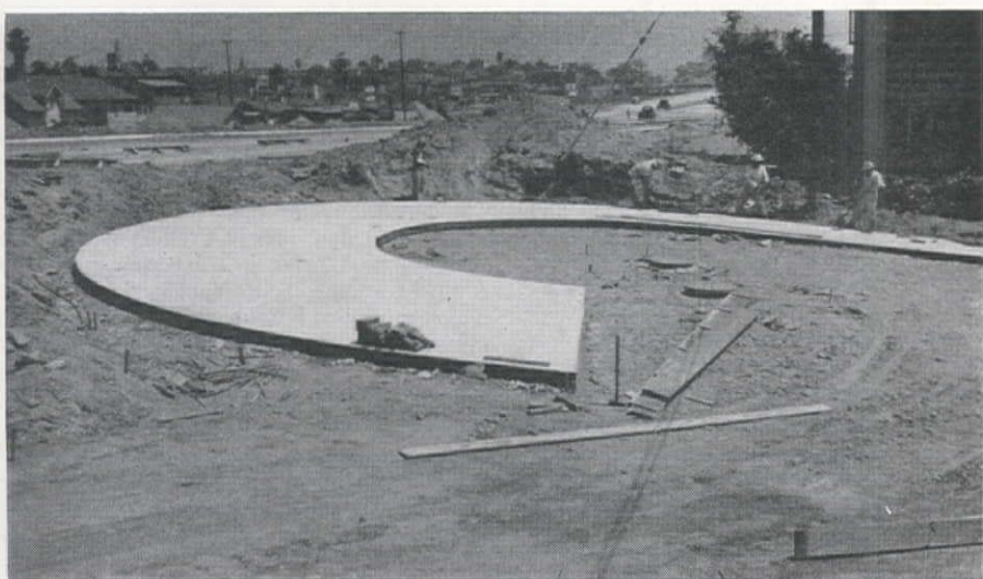
TIGHT RAMP CURVATURES and super-elevations cramp machines and call for slow, costly hand finishing—another characteristic freeway construction problem.
