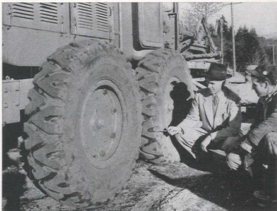
Universal Tires—These new BFG Tractor Grader Universal tires have rolled 240 hours for the N. Fiorito Company. This operator particularly likes the non-directional Universal tread.
