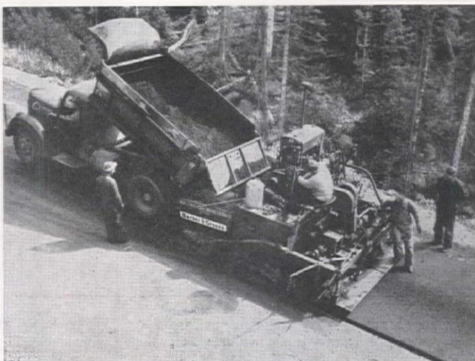
TODAY, modern plant-mix pavement is the standard on the main highways of the Mountain States with continuous plants (left) getting increased recognition and lay-down machines (right) completing the process.
