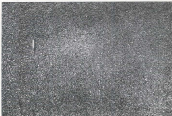
OREGON —Cinder aggregate was used for this seal coat on U. S. 20, Bend to Burns highway. Detail of texture (right) shows the surface of the \frac{1}{4} -in. to #10 mesh cinders. Skid tests showed this surface to have the highest coefficient of friction of all tests made.
