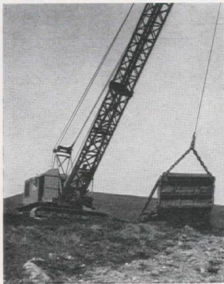
MORMON BOARD performed rough backfilling (left and below) along most of section A-1, was followed by bulldozers and grader to restore original contour.
