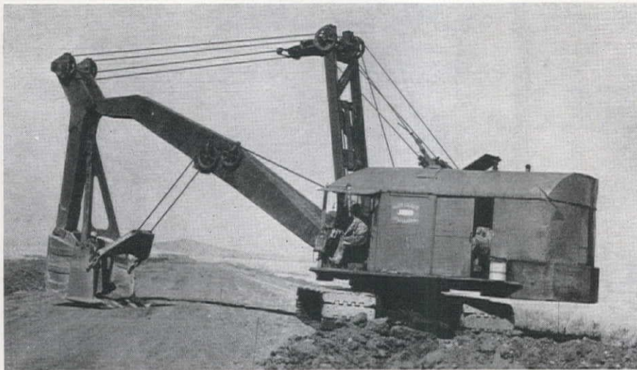
BEEFED UP Lima (left) followed blasting to excavate trench in rugged upper reaches of United Concrete Corp. contract. (Photo by Gene Edwards.)
