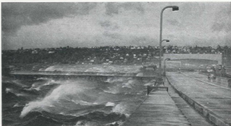
PROVING THE STABILITY of the concrete-barge bridge, which has a flotation depth of 7\frac{1}{2} ft., the structure is shown being buffeted by a 60-mph. wind.
