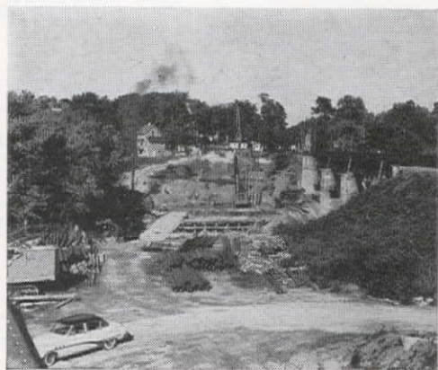
Overall view of foundation work for new bridge showing storage yard, pile assembly rack at left, and driving operation in background.
