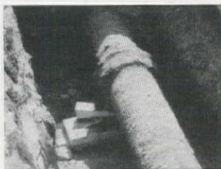
One of a number of cast iron water mains which have been in service in New York City for more than a century. Over 35 other cities have century-old cast iron mains in service.
