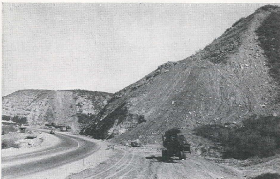
AT THE SITE, plant is ready to process the rock in this sidehill cut that will provide added width for two more lanes. One set-up will be made at each end of 700-ft. length of cut without stockpiling.
