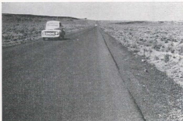
OREGON —Cinder aggregate was used for this seal coat on U. S. 20, Bend to Burns highway. Detail of texture (right) shows the surface of the \frac{1}{4} -in. to #10 mesh cinders. Skid tests showed this surface to have the highest coefficient of friction of all tests made.
