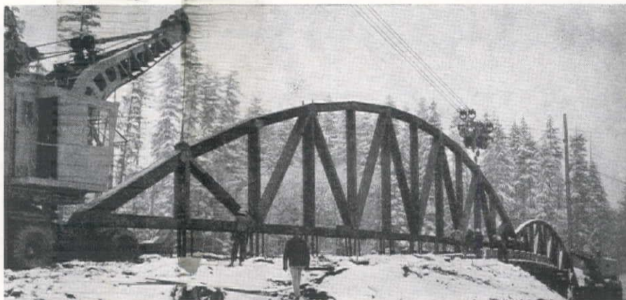
ERECTION of 30-ton trusses was carried out using four 1\frac{1}{4} -in. cables as skyline attached to a self-propelled "sky hook." Another view of completed bridge is shown below.
