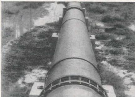
Over swamps and marshy ground, where earth movement must be considered, Dresser Couplings keep Savannah's new 14-mile, 42" water supply artery completely tight.
