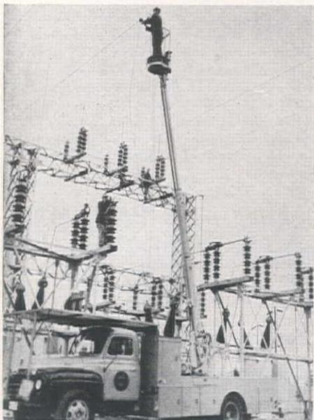
The "monkey" (see cut) consists of a hydraulically operated telescoping boom with a self-leveling cage that takes a workman directly to the spot where he must do his high work. In operation, the
