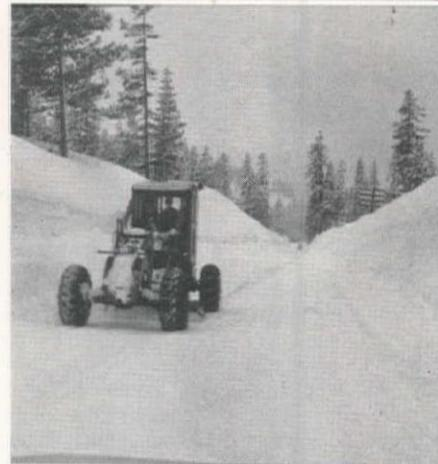
WITH SNOW STILL falling, a push plow shoves a windrow to the side with normal traffic on the highway.
