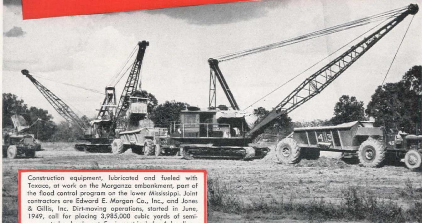
Construction equipment, lubricated and fueled with Texaco, at work on the Morganza embankment, part of the flood control program on the lower Mississippi. Joint contractors are Edward E. Morgan Co., Inc., and Jones & Gillis, Inc. Dirt-moving operations, started in June, 1949, call for placing 3,985,000 cubic yards of semi-compacted embankment. Equipment includes 4 draglines, 9 tractors and 53 trucks — all of which are lubricated with Texaco exclusively.
