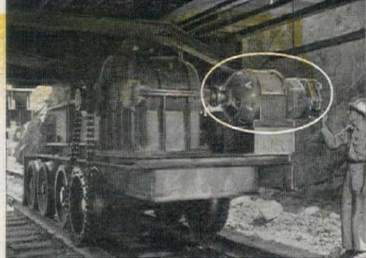
Under the head tower, this G-E 75-hp wound-rotor induction motor is one of two that drive the tower. Motors for head and tail towers are controlled by a single master switch in the operator's station.
