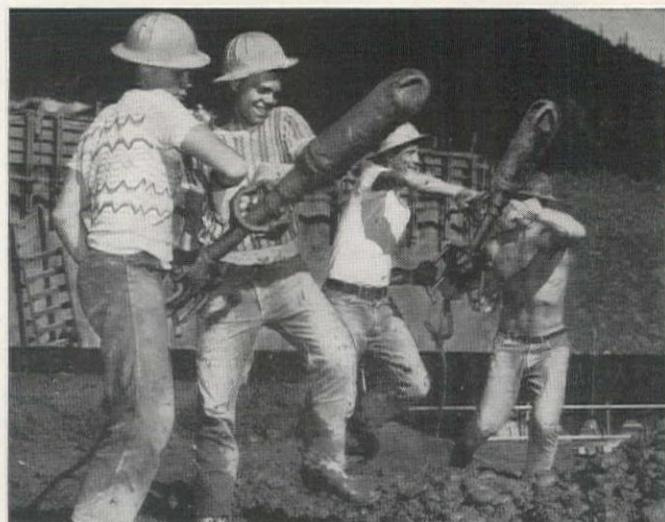
Seven different models of CP PNEUMATIC and ELECTRIC VIBRATORS enable the contractor to select the proper model for any specific job. Two-man vibrators speed the heaviest mass concrete placement. For reinforced walls, columns, floors, and similar work, there are small diameter pneumatic and electric models for one-man operation.
