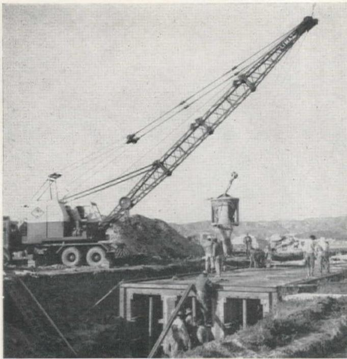
POURING a 75-ft. section of culvert from 1-yd. bucket supplied by transit-mix. After concrete had set, forms were stripped and re-set in one shift.
