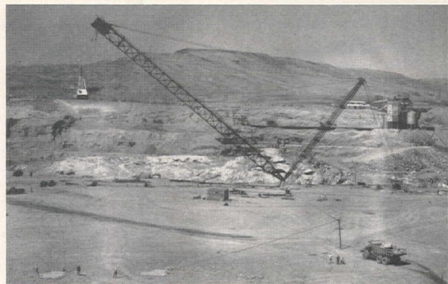
TAIL TOWER MAST, weighing 118 tons, was completely assembled in a horizontal position and raised in a few minutes' time by the use of two crane booms which were set up on either side of mast base as erection poles. Tractors were used to pull booms down and mast up.
