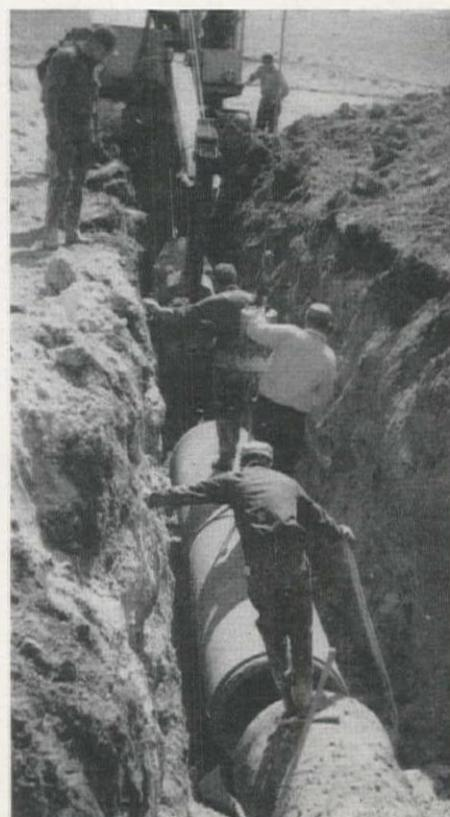
stressed concrete cylinder pipe.
