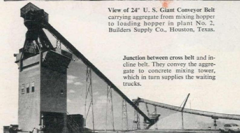
Junction between cross belt and incline belt. They convey the aggregate to concrete mixing tower, which in turn supplies the waiting trucks.
