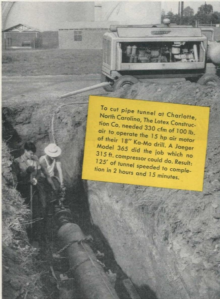
To cut pipe tunnel at Charlotte, North Carolina, The Latex Construction Co. needed 330 cfm of 100 lb. air to operate the 15 hp air motor of their 18" Ka-Mo drill. A Jaeger Model 365 did the job which no 315 ft. compressor could do. Result: 125' of tunnel speeded to completion in 2 hours and 15 minutes.
