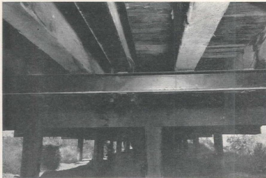
**COMPLETED JOB** showing transverse channels brought up to contact with timber bridge stringers by means of U-bolts, which pass through a hole in the I-beams.
