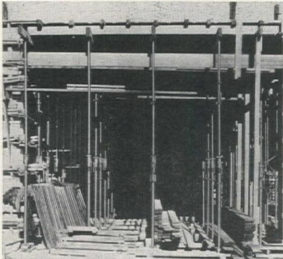
adjustment, and only three sizes cover a range all the way from 6 ft. to 15½ ft. above the mounting surface. The three sizes of Safway shores have height ranges for 6-11 ft., 8-13 ft., and 10½-15½ ft., respectively. The special sleeve nut design makes possible heavier load-carrying capacities to as high as 9,900 lb., with adequate safety factor. No jacking devices or other separate accessories are required. For rough adjustment the upper telescopic member is easily raised to
