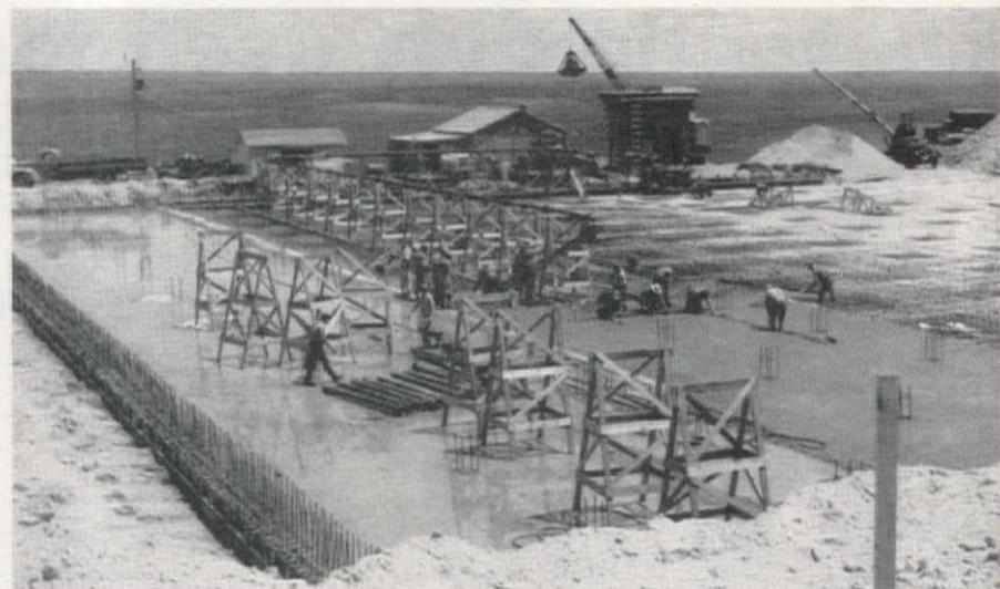
CONCRETE for the 5-mg. covered reservoir was distributed from pump set-up (left) by elevated pipe to the point of pour on the slab (above). Primary function of the reservoir is to regulate and store output from the fourteen new wells. The structure adds 50% to Cheyenne's total storage facilities.
