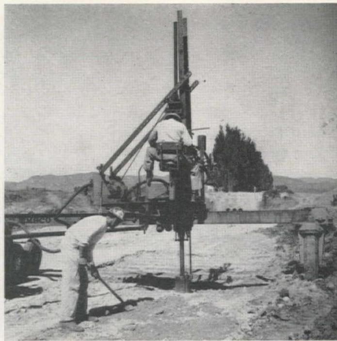
TAMPING 900 sq. ft. per day to 90% optimum density, this rig worked on 2½-ft. backfill lifts. Hammer was powered by a truck-mounted compressor.
