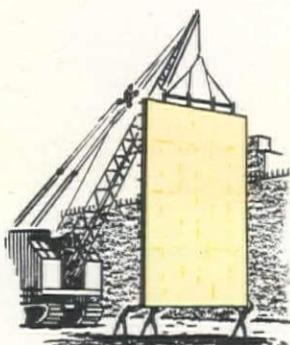
**COVER ILLUSTRATION:** Artist's conception of Exterior plywood form sections used for foundation walls of Port Authority Bus Terminal, N.Y.C. Consultant Engineer Jacob Feld, N.Y.C., who designed 28'-high by 24'-long pre-assembled plywood sections, reports "forms very successful. Six re-uses on walls, plus re-use on other parts of building, but forms could have been used indefinitely." Contractor: Foss, Halloran & Narr, Inc., Long Island City, N.Y.
