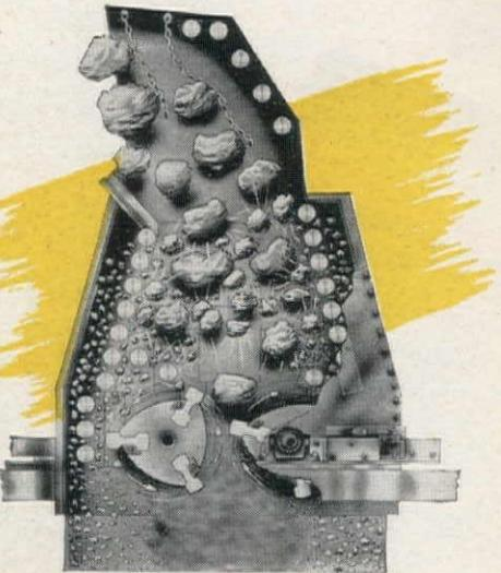
Approximately 50% less contact of stone on metal, because such a high percentage of material is broken in suspension.
