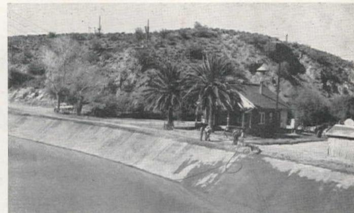
**BEFORE AND AFTER.** Unlined bank of canal (left) prior to start of work, showing porous type of material and large trees which aggravated the seepage problem. Completed section (right) near same location with banks graded to smooth 1:1 slope and gunited.
