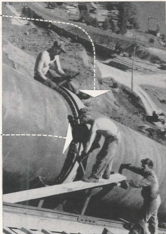
75" penstock of the British Columbia Electric Co. One of three installed at Bridge River, using Dresser Couplings specially designed for the job. With Dressers, construction time was cut from months to weeks, due to simplicity of installation. And penstocks have remained bottle-tight under very high pressures, despite severe weather conditions.
