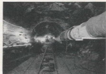
Under New York Harbor, construction of the Brooklyn Battery tunnel was simplified by using Dresser Couplings to join air and water supply lines.
