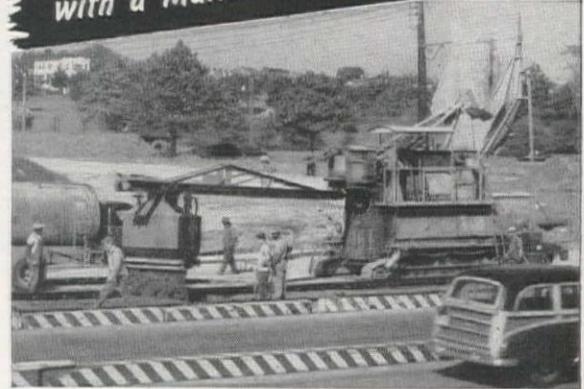
MultiFoote 34-E DuoMix getting out 50 batches an hour even with difficult traffic conditions impeding trucks.
