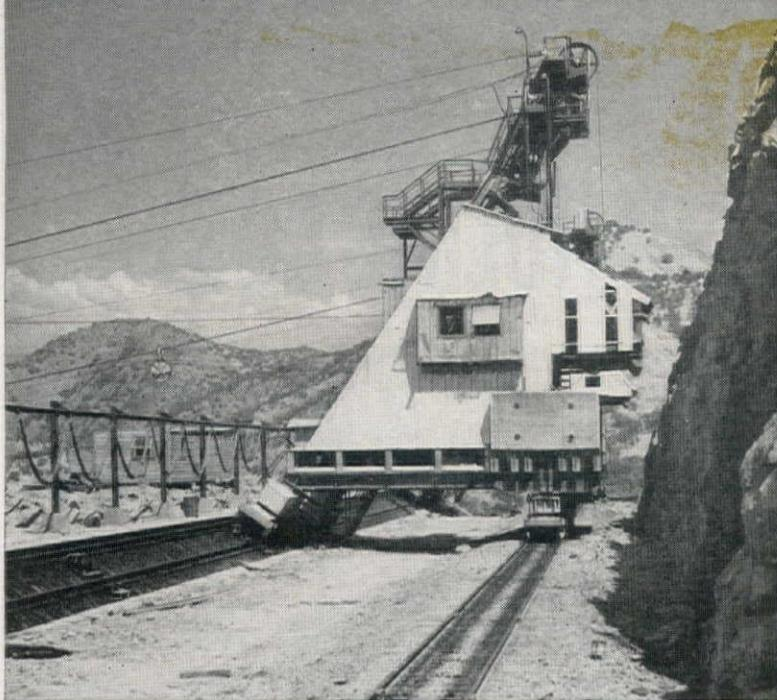
Cableway head tower, and tail tower across the canyon, are both driven on straight parallel tracks by G-E drives. Another set of towers for the service rig operates on the same tracks. Main cableway was built by Willamette Iron and Steel Co.
