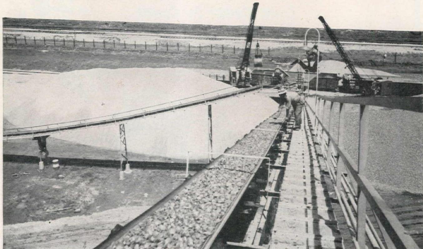
View of 24" U. S. Giant Conveyor Belt carrying aggregate from mixing hopper to loading hopper in plant No. 2, Builders Supply Co., Houston, Texas.
