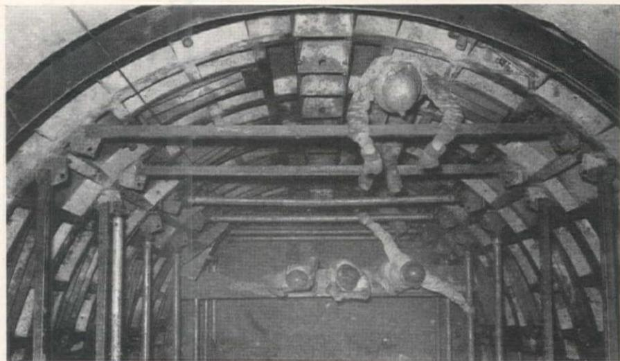
STEEL FORMS followed excavation as 25-ft. vertical segments of concrete shaft lining were poured. Shaft was never mucked more than 30 ft. below completed lining, a precaution against possible hydrostatic pressure effects on the protective ice wall.
