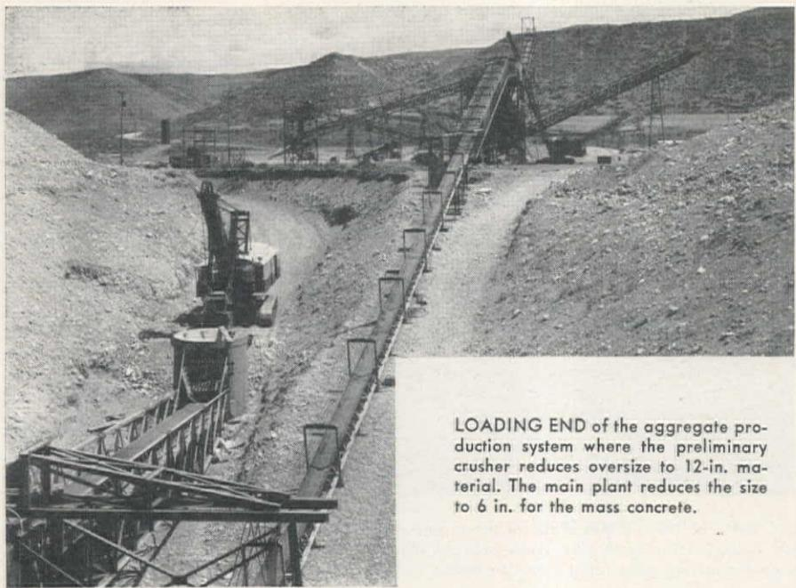
LOADING END of the aggregate production system where the preliminary crusher reduces oversize to 12-in. material. The main plant reduces the size to 6 in. for the mass concrete.
