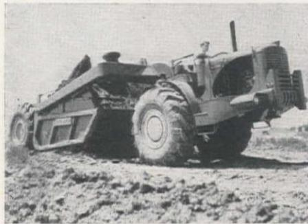
equipped with a 13-cu. yd. scraper for contractors, and others who require such a machine for maintenance, stockpiling, etc. The model has the exclusive Hydro-Steer, unobstructed visibility, big, safe, heavy-duty 2-shoe air brakes synchronized on both the tractor wheels and the trailing unit wheels, and speeds up to 25 mph., even when loaded. A 165-hp. Model HRB600 Cummins diesel engine powers the 500 Heiliner (pictured above). The Heil Co. is the manufacturer.
