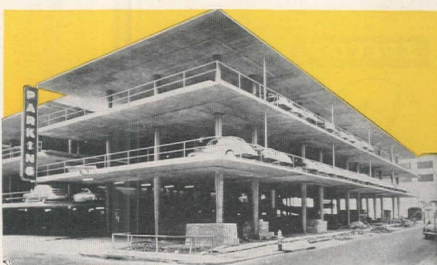
New Orleans parking garage, built in 30 units, cost only \$400 per car space. Unit is a 32' slab cantilevered on columns spaced 16'. Overlapped cantilevers between units span 32', make space for another car. In cross section slabs are 66'3".
