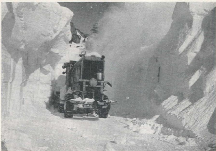
OVERHANGS were a constant threat to working equipment. Best method used to cut them down was the use of a cable looped between two tractors.
