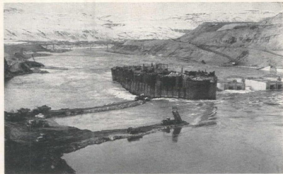
**CLOSURE BEING COMPLETED** for the second-stage diversion. The Columbia is flowing through low blocks on the north side. Area between the two rock arms was filled to provide a working area for driving piles for the cells to extend cofferdam to the south shore.
