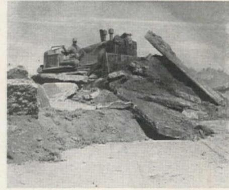
Between Colorado Springs and Pueblo, Colo., Schmidt Construction Co. has this Gar Wood cable-operated dozer blade on an Allis-Chalmers HD-20, tearing up old concrete slab.
