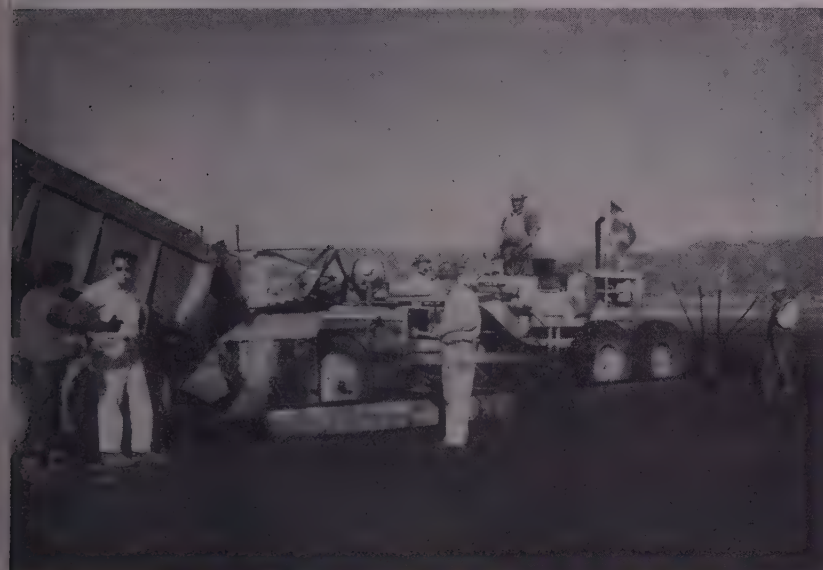
DB-DEVELOPED SPREADER and leveler for plant-mix base course. This motor grader was equipped with an 18-ft. width of screed and was able to spread up to 200 tons of material per hour.
