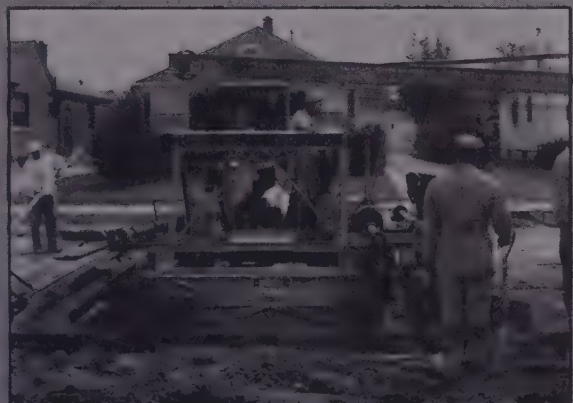
Ruggedly constructed, the Detroit Special has reversible screeds that are mounted outside the frame for greater accessibility.
