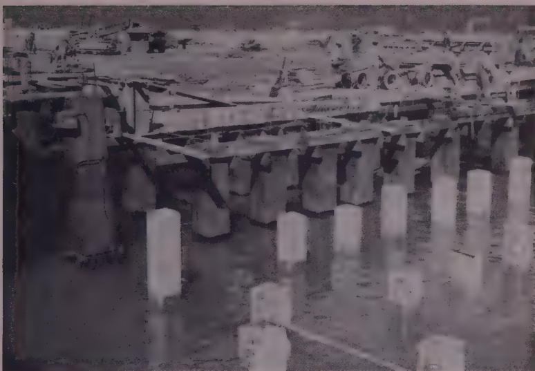
JACKETS slipped down over concrete piles provide protection in the tidal range and also allow for establishing grade without cutting off piles.
