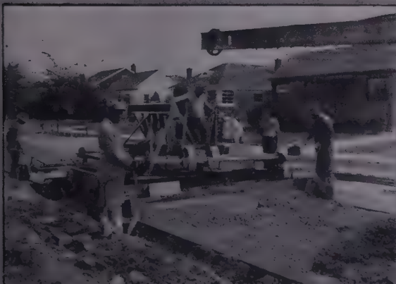
Note compact, low slung design. Transportation wheels are retracted. Heaviest masses of concrete are handled with ease.
