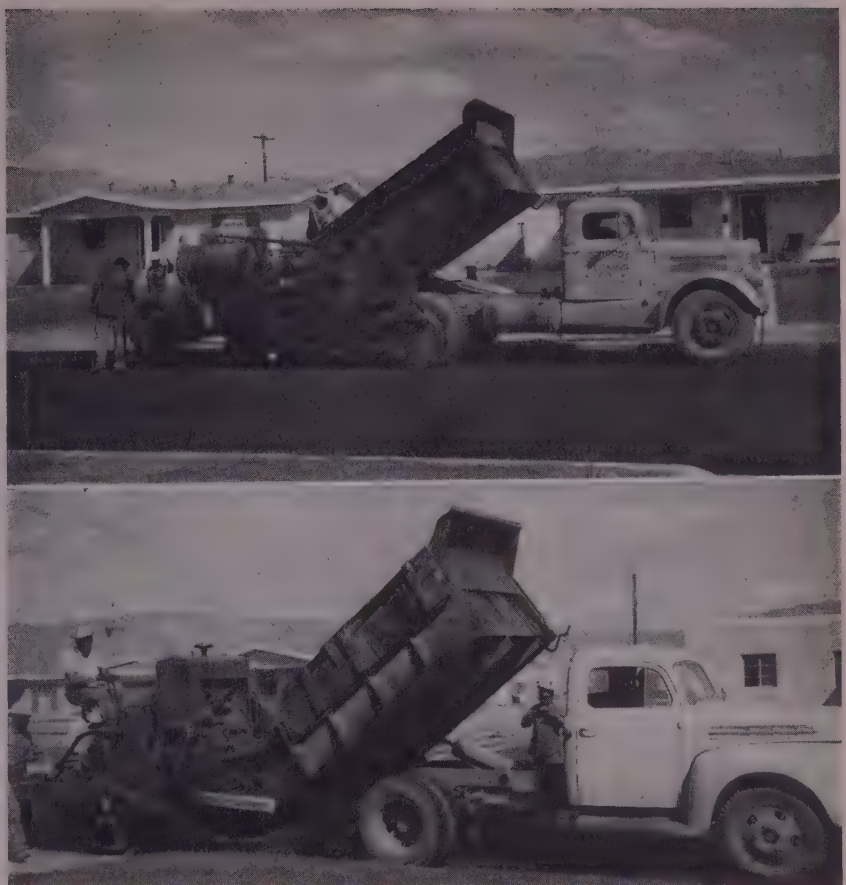
TYPICAL OPERATIONS on the street. Top—One of the two Adnun machines of Allison & Haney which were often worked in tandem. Bottom—Barber-Greene operated by Wylie Brothers.
