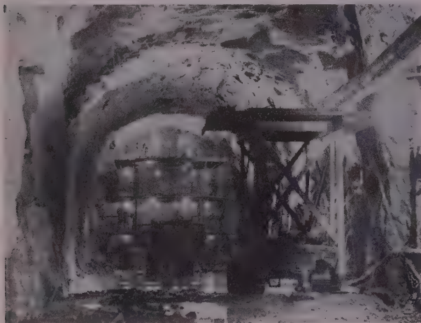
WORK on a drill jumbo advances the tail-race tunnel that will extend from the powerhouse inside the mountain to the Kemano River.
