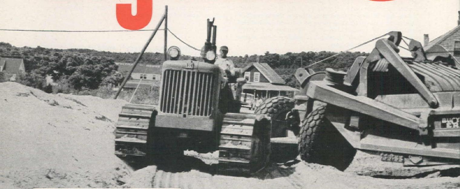
**TIGHT TURN AT THE TIP** of old Cape Cod, a big International TD-24 crawler with a 21-yard heaped-capacity scraper wheels around to start another 1,800-foot haul on the new Mid-Cape Highway extension, near Truro, Massachusetts.
