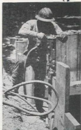
**Powerful Driving** — with Gardner-Denver Sheet Driving Drivers. Adjustable jaws. Safety latch. Removable foot rests.
