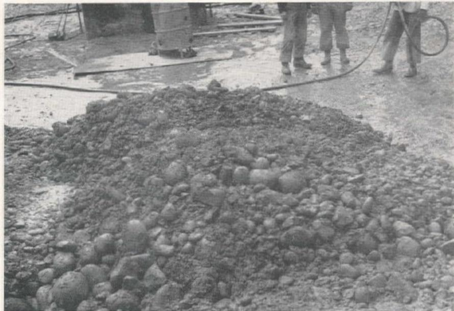
INTERIOR MASS CONCRETE at Pine Flat, a 2-bag mix, looks like this when discharged from 8-yd. dual compartment controlled-dump bucket.
