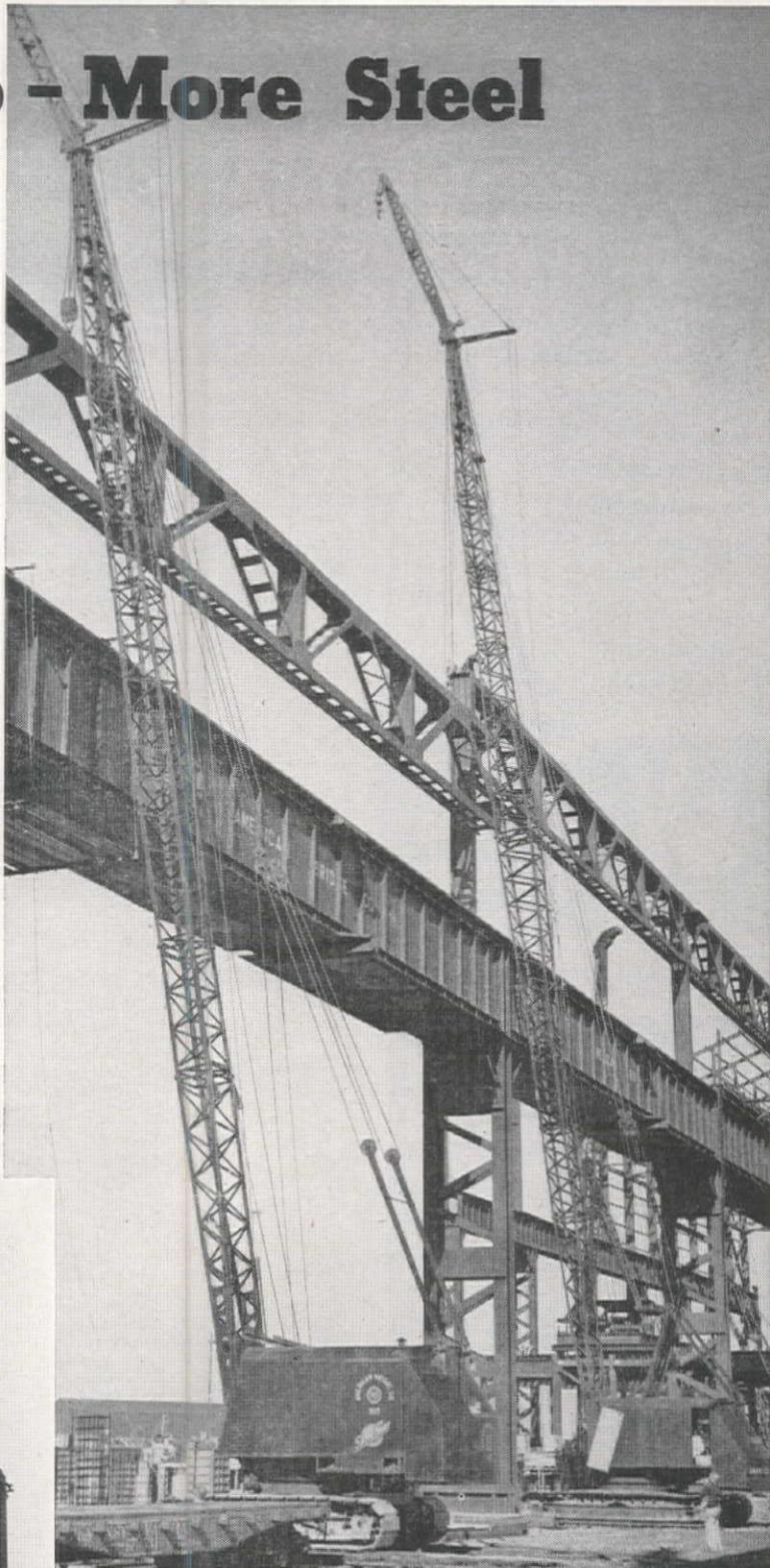
American Bridge uses a Model 3500 and a Model 3900 Speedcrane to set a heavy girder for the Open Hearth building. Reach plus stability means speed and safety.
