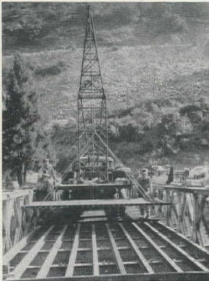
PRE-CUT PANELS of open-mesh decking were laid from truck rolling over earlier work.
