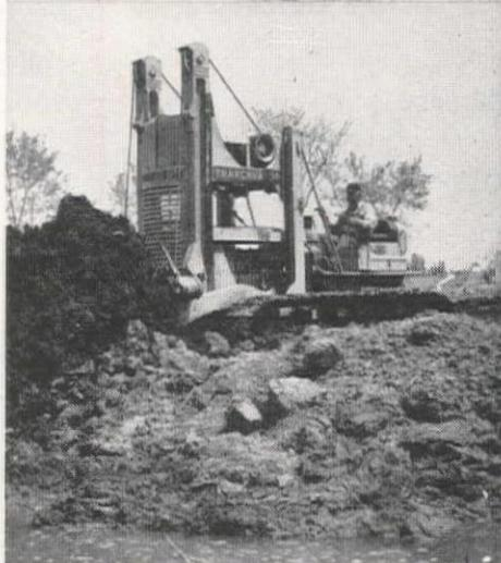
• A heaped load of wet, gummy topsoil is dug and dumped into an old creek bed by the T6 TRAXCAVATOR, owned by SMH. The work is in connection with a new housing development.
