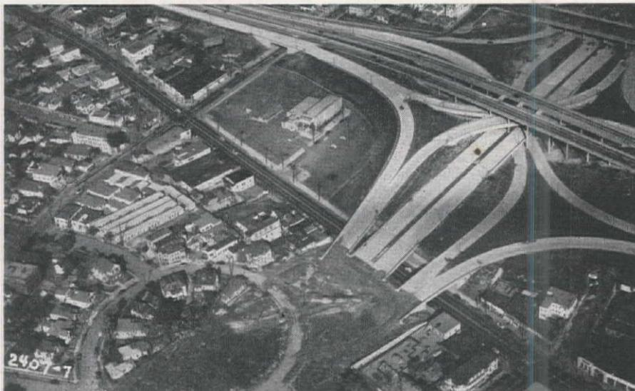
LEFT—Four-level grade separation on the route allows motorists access to adjacent residential districts. Work in foreground shows the pattern of right-of-way from which houses were removed.
