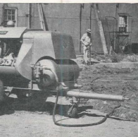
**Full Air Capacity** — at any altitude — with the Gardner-Denver Two-Stage WH-105 Gasoline Powered Portable. Fully water-cooled cylinders for dependable operation, regardless of weather or temperature extremes.
