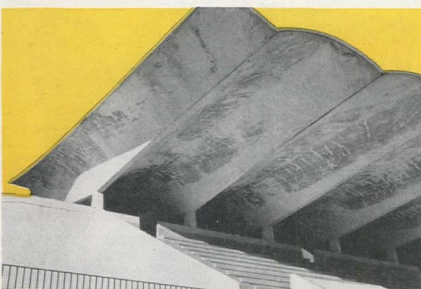
In this shell-concrete roof, each scallop serves as a beam, permitting a 42' cantilever over spectator stands.
