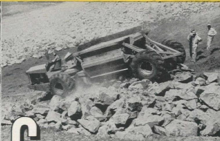
**FAST DUMPING — NO GATE DAMAGE** — Clamshell-type gate action clears load, eliminates gate damage when dumping rock. Independent electric power opening allows rig to stop over hopper, dump without having to be in motion.
