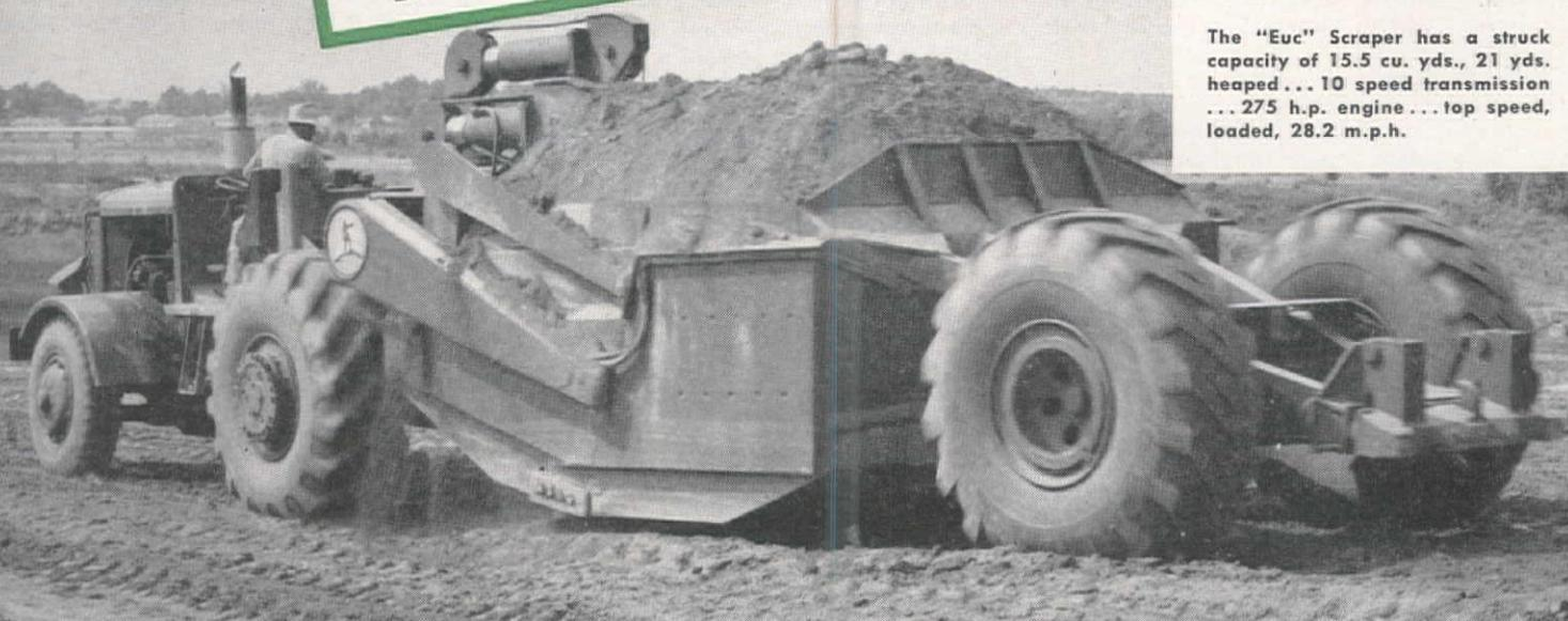
The "Euc" Scraper has a struck capacity of 15.5 cu. yds., 21 yds. heaped... 10 speed transmission... 275 h.p. engine... top speed, loaded, 28.2 m.p.h.
