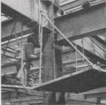
Fig. 2. Detail of Girder running through column. Column top and base are welded to beam flange. Vertical stiffeners provide continuity to column.
