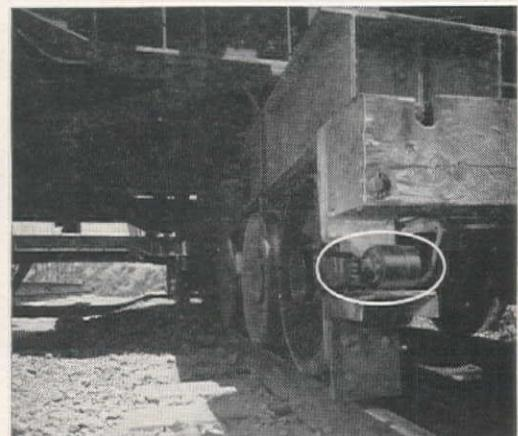
Tower alignment is maintained automatically. This selsyn generator, connected to a head-tower wheel, and another on the tail tower, feed signals to a differential selsyn which controls speed of the tower-drive motors.
