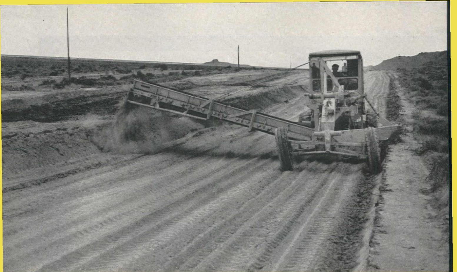
This "Cat" No. 12 Motor Grader, equipped with DoMor elevating grader, is side burrowing at the rate of between 500 and 600 yards per hour.
