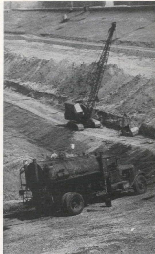
ASPHALT IS APPLIED in the excavated trench between the sheetpile cutoff and the toe of the dam. This general view shows the two access roads on dam, stockpiled spoil, line of sheet piling and equipment at work.
