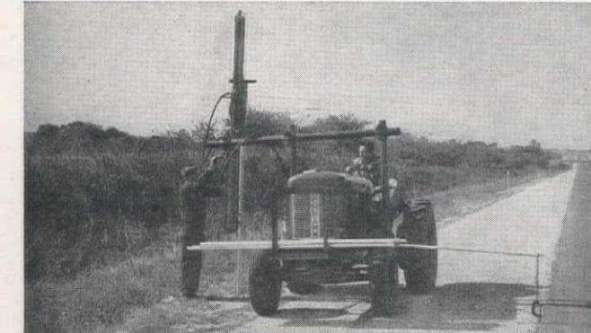
that are to be driven. The Pneumadriver, mounted on the Schramm Pneumatractor is used for the driving of steel or wooden fence posts in 1/10th the time required by the old hand method. On-the-job this machine with a two-man crew was able to drive 350 stakes per day. Schramm, Inc. is the manufacturer.
