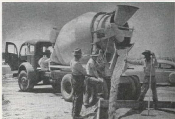
with "dual-mix" action, to which any additional equipment may be added to meet each operator's particular service requirements. Drum, frame, front trunnion and drum roller assemblies, in all models, are designed to handle the maximum volume of material which operators may wish to carry. All models also are equipped with mudguards and catwalks and the 3-piece "Swing-Away" chute which meets all discharge conditions.
