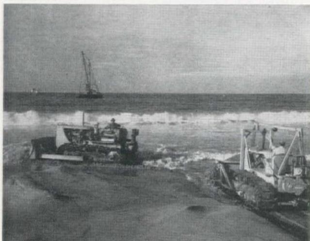
TRACTORS bathed in the surf to extend the trench on rough grade to breaker line in the surf.
