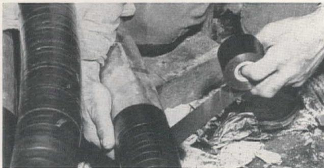
new Scotch brand tape No. 21 offers more-than-average strength. Minnesota Mining and Manufacturing Co. also recommends this new tape for protecting and insulating cable and high tension leads subject to wear, abrasion, rough handling, and for bus bars carrying high voltage. The tape has a black, vinyl plastic backing that is 20 mils thick—more than twice the thickness of previous tapes of its type. It has a dielectric strength of 22,500 volts, an insulation resistance
