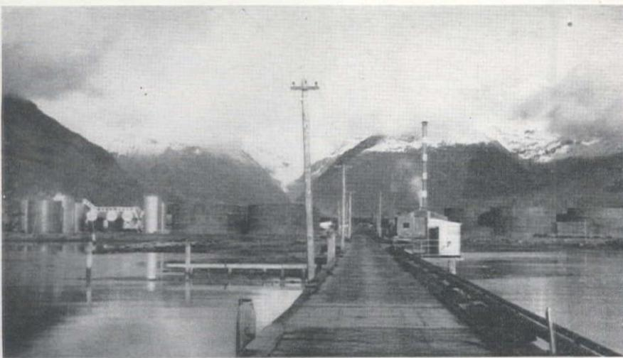
ARC's tank farm at Valdez houses fourteen 10,000-bbl. units, which is a year's supply of liquid asphalt. Use of RC-3 grade avoids shipping and handling asphalt cement in drums.
