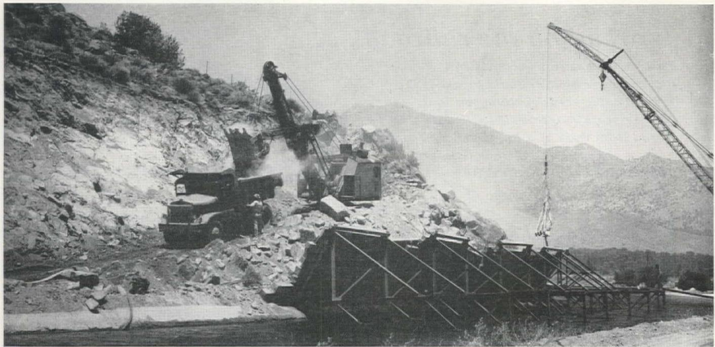
**ADJUSTING THE ANGLE OF REPOSE** of banks bordering Southern California Edison Co.'s Borel Canal without hindering canal operation presented a problem to Bechtel Corp., second stage construction contractor on the project. To keep debris from falling into the canal, which delivers water to Borel Powerhouse, the firm erected portable steel bulkheads (pictured above) to catch rocks and dirt which ordinarily would
