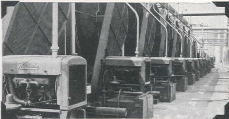
144 HIGH-SPEED BEARINGS in 72 magnetos on various types of engines required servicing at 1- to 3-month intervals until Calol O.H.T. Grease was used on them. Now they are serviced only at intervals of 3 to 6 months, although heat from the continuously operating engines keeps "drive-end" bearings at an aver-
