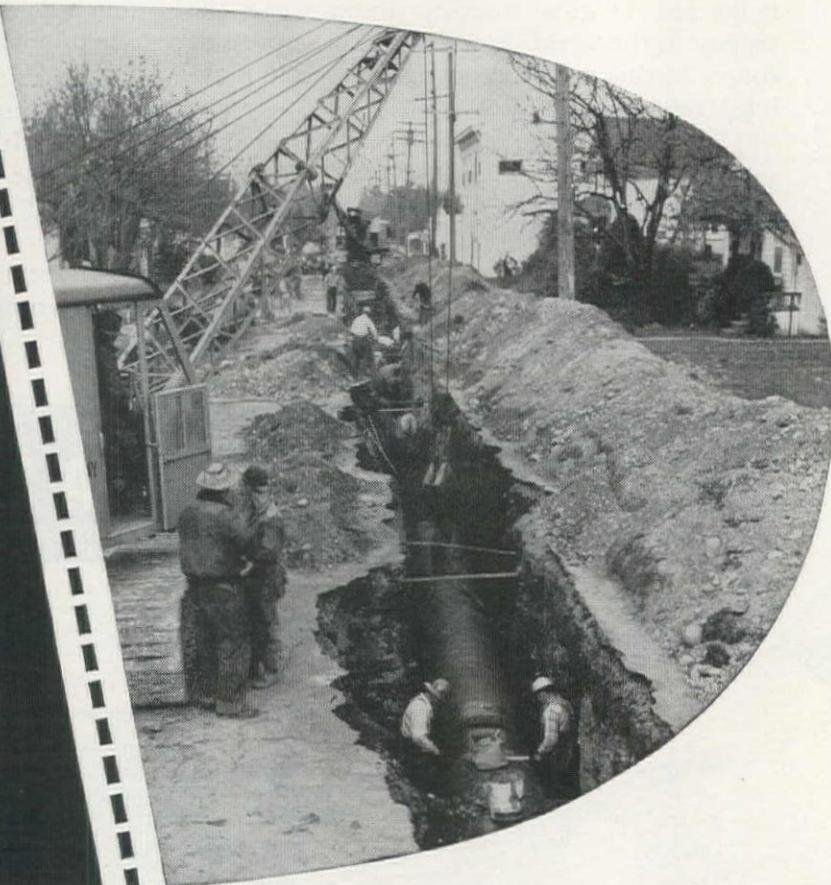
The cheapest way to deliver water to the place where it turns into revenue is with a Dresser-Coupled steel line—the line that cuts *installation* costs, *leakage* losses and *maintenance* costs.
