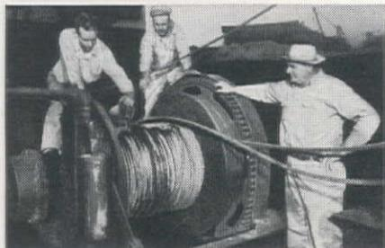
For longer rope life, Mr. Billi's advice is regular lubrication with a good grade of wire rope dressing. He says: "Pile-driving operations in the salt air here are plenty hard on lines, so that even rope as tough as Tiger Brand needs this extra care. We find that it definitely prolongs rope life."
