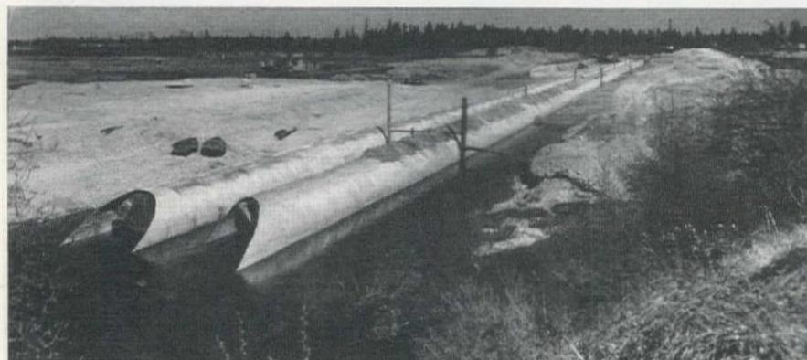
**SIDE BY SIDE**, the two giant culverts lie in the channel where they will carry the waters of Clover Creek under the extended runway of McChord Air Force Base.
