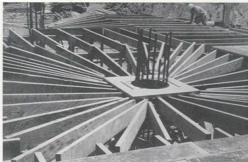
FRAMING for a haunched column with the 2 x 8 joists in place ready for the metal slab forms. A special sheet-metal valley is used down the four corners. The transition section extends the 26-in. round column to a 4-ft. square.
