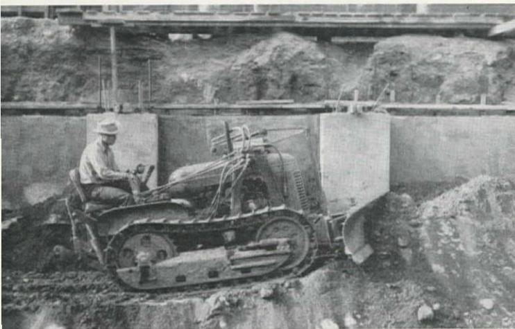
WALLS are extended downward by dozing out the berm in 4-ft. lifts (left) and then shooting a 5-in. gunite wall between the precast columns. This sequence was extended down to the bottom floor.
