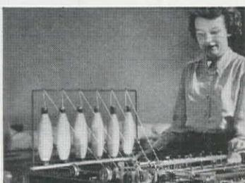
One of a series of comprehensive laboratory controls throughout production to assure uniformity in all Mt. Vernon-Woodberry products. The unit shown automatically tests 6 strands of yarn at one time.
