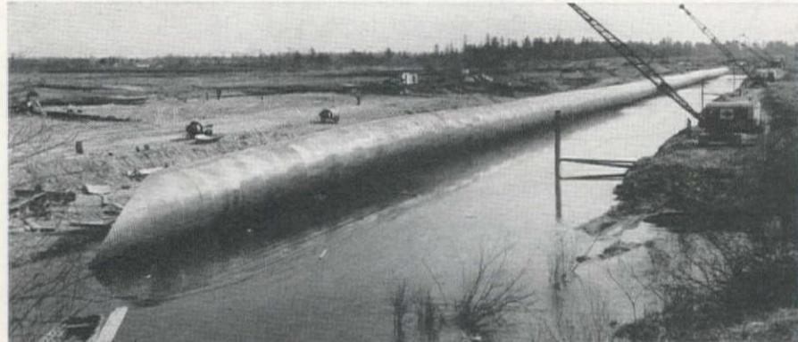
**TEAMWORK** of seven tractors on the left bank and four cranes on the right bank is used in the launching. Following instructions relayed by radio and from loudspeakers, the tractors pulled the chocks from under the culvert and the cranes took up the slack in cables to haul the unit into position against the pilings.
