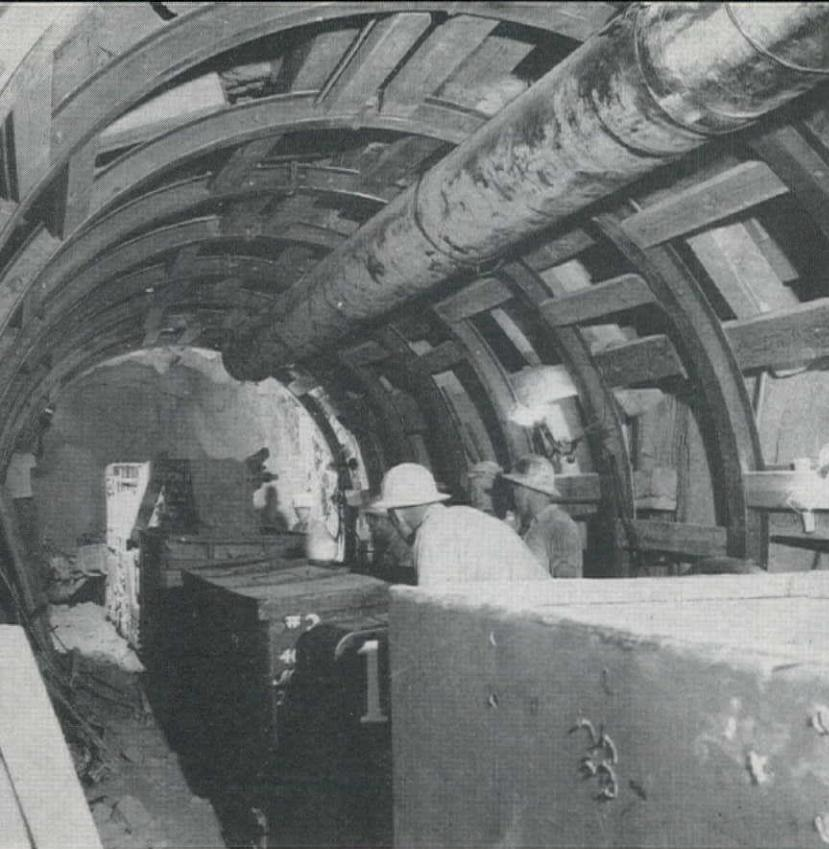
**Holing through of 6-mi. bore for Los Angeles hydro project completes driving on last of three tunnels — Mucking operation (left) removed 357 cu. yd. per day, or a 78.77-ft. advance, for 31 consecutive working days. Best 24-hour advance was 104 ft. It all adds up to . . .**
