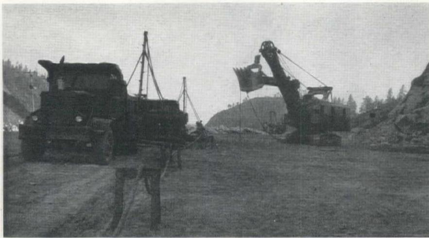
PARADE OF EQUIPMENT leaves quarry prior to blast. Trucks are hauling tower sleds used to keep electric power cable in clear, while shovel "picks up its skirts" and follows.
