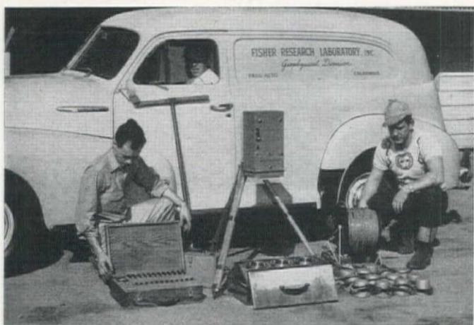
REFRACTION seismic equipment, compact and portable, is shown here, left to right: amplifier case (open), recording galvanometer (on tripod), geophones and connecting cables.
