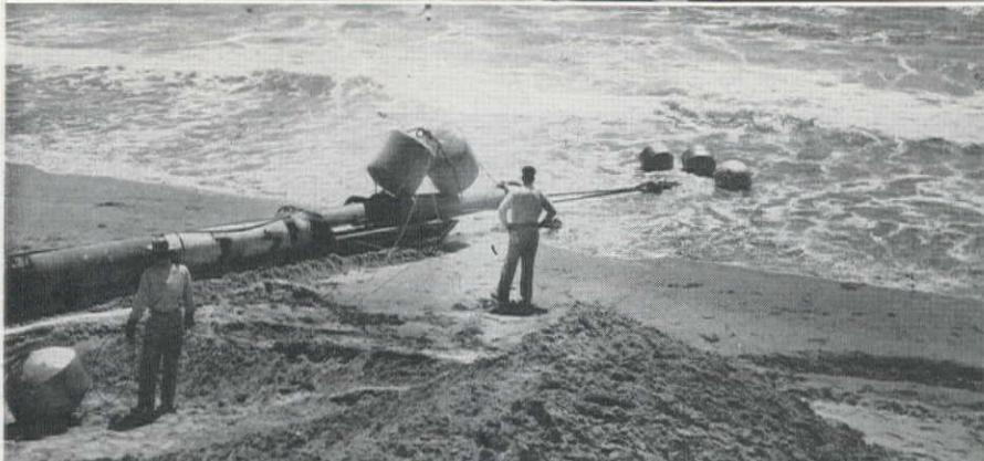
TOP—View of Caterpillar side-boom tractor units used for laying part of the submarine pipeline for Union Oil Co. near Ventura, Calif.
