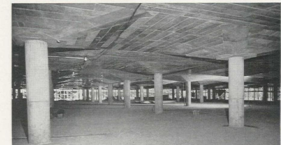
placed in the forms. Later the lower mat of reinforcing slab steel was set, followed by conduit installation and upper steel mat. Round steel screed posts with steel spikes were set in small holes already in the metal pans. Later a cast arm which supported a 2 x 4-in. guide was set to establish finish floor grade. Steel inspection, clean-up and the installation of 5-ft. wide runways for motorized buggies prepared the area for placing the concrete.
