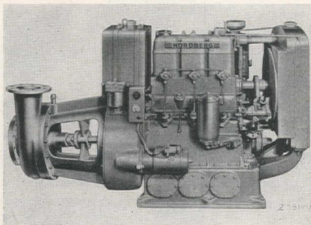
stationary and portable applications. The engine features a 4½-in. bore and 5¼-in. stroke. It is available as an electric generator set, pumping unit and with clutch or stub shaft power take-off for direct connection or belt drive. Can be obtained, ready to connect to a load, in direct or alternating
