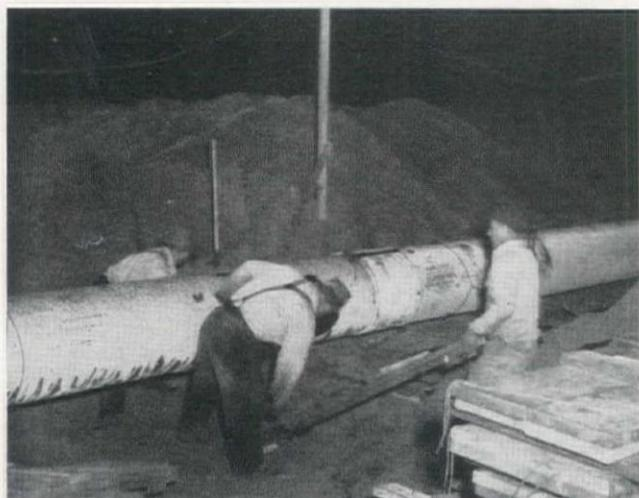
SKIDS were removed during the pulling operation when they reached a depression previously excavated at the end of runners.
