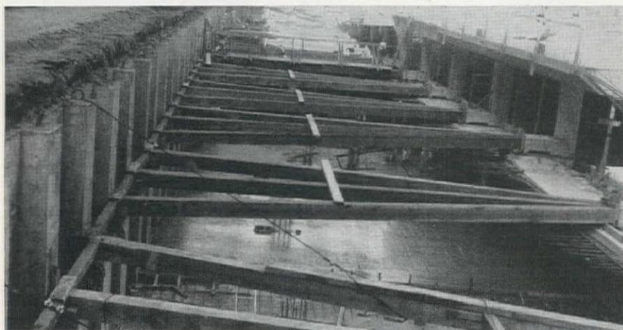
BELOW—Haunch columns provide a streamlined appearance to the second sub-floor ceiling, with a pleasing pattern produced by the metal pan forms.
