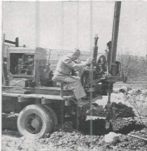
•HBR Earth Drill drilling large diameter hole.
