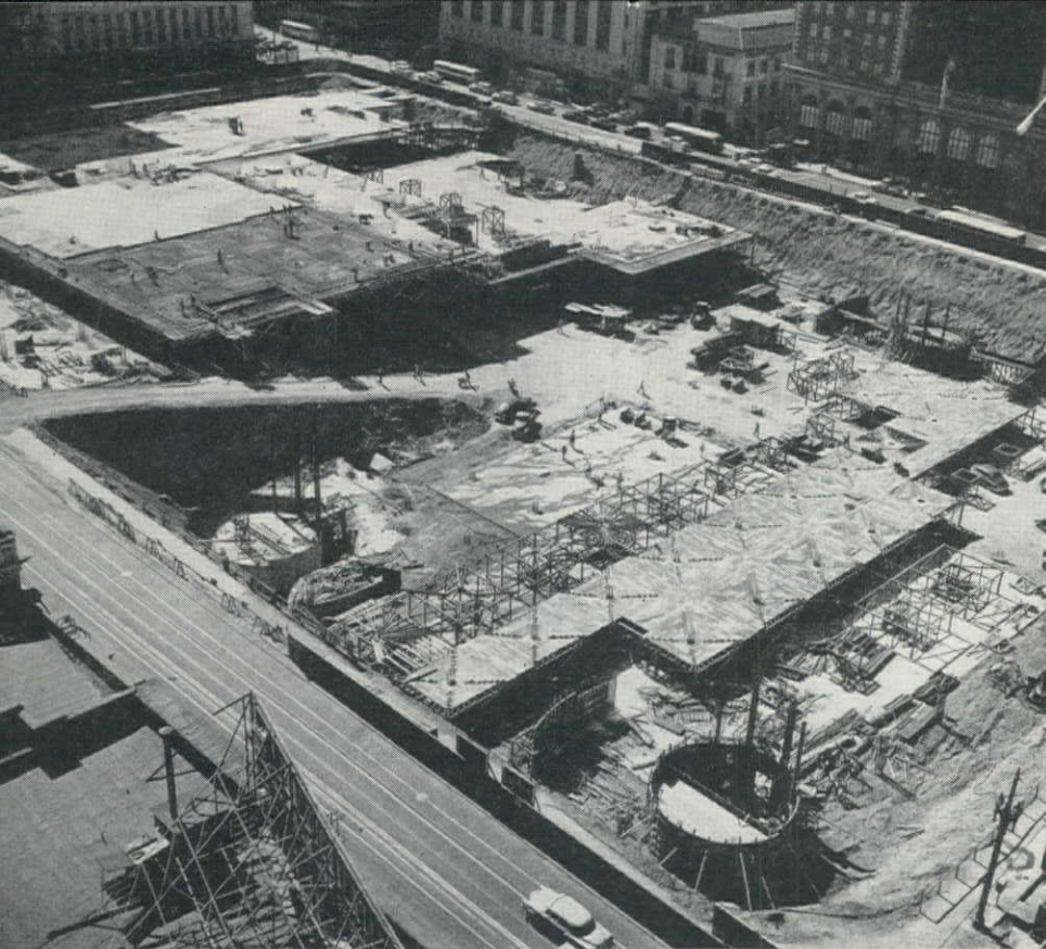
Municipal parking feature is Los Angeles' 2,000-car subterranean Pershing Square garage covering a full city block and estimated to cost about $5,000,000. With excavation completed, activity now centers in formwork and concrete placement.
