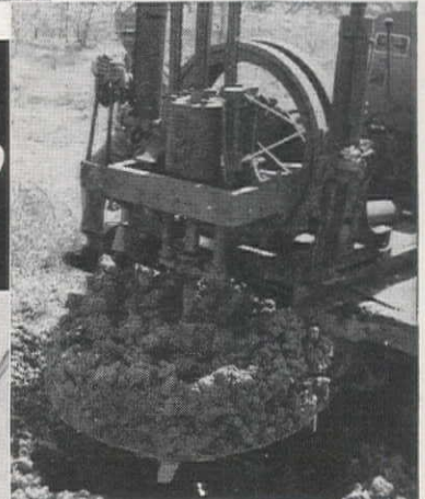
View showing helix loaded with dirt withdrawn from hole.
