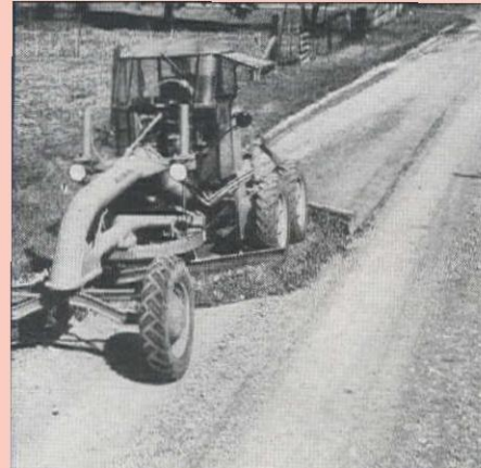
Maintains roads and streets. Windrow eliminator feathers out windrow.
