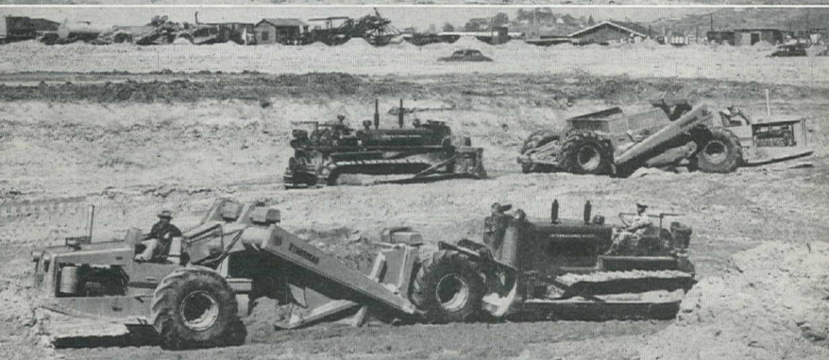
On this 4200' cycle, 6 "C's" delivered about 62 loads per hour... their total production per 8-hour day was 5020 pay yards of sandy clay.
