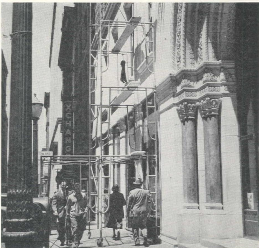
LIGHT STEEL scaffold has open frames that give clearance and double as ladders.
