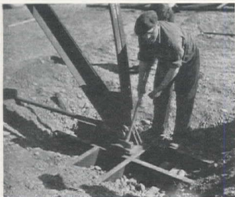
DETAIL of bottom pin connection (left) shows bearing plate, and tie rod leading to opposite end of truss. Crown-pin connection (center) was assembled on one truss section, joinery made by bolting angles to
