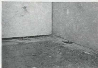
ERECTION CREWS (top) make fast work of positioning a carport roof slab handled by 25-ton truck crane. Slabs are seated on sponge rubber seals nailed to top of wall, are later bolted down and grout poured to make reinforced joint. Bottom, interior view at corner shows leveling bolts that support panels on footing until connection is welded and gap gunited. Steel bearing plates are cast in footing. Floor slab will completely cover gap.
