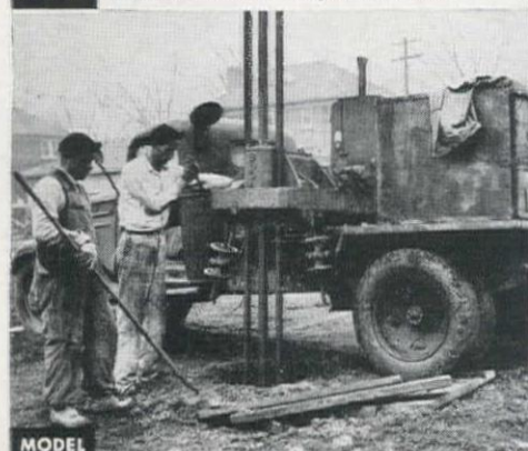
MODEL HBD 12" to 42" dia. - Depths to 24 feet
