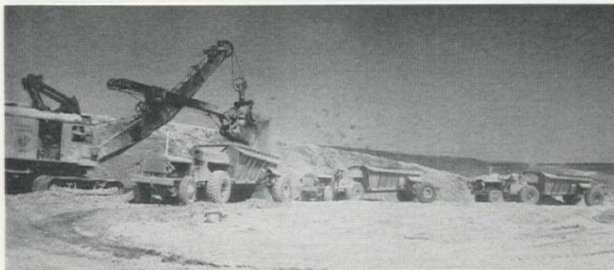
BOTTOM-DUMP Euclids momentarily gang up on loading shovel (above) as they helped maintain the 18,000-cu. yd. per day earthmoving schedule. Bottom-dumps were used primarily to transport material for the upstream and downstream shells of the embankment.
