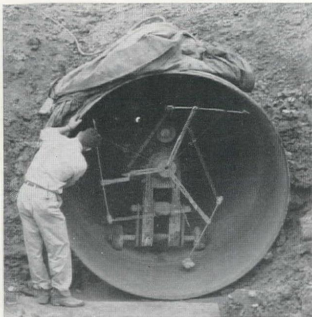
CENTRILINING MACHINE began at west portal and worked east, applying \frac{1}{2} in. of mortar to pipe surface. Tunnel is 90-in. I.D. after lining, has capacity of two 72-in. pipes, providing for future expansion of system.
