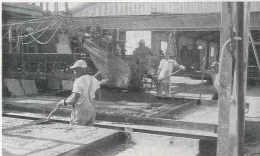
FIRST AND LAST STEPS of casting plant operation are seen at upper left, as power broom cleans form cars upon their return from panel stripping by girder crane in background. Successive crews on assembly line ready the forms for casting. At upper right, reinforcing steel is placed in a roof slab. Note insert in foreground, providing hole for eventual assembly bolt. East of the assembly shed (lower picture), form cars roll under traveling concrete conveyor, are poured in two passes, using lightweight pumice concrete.
