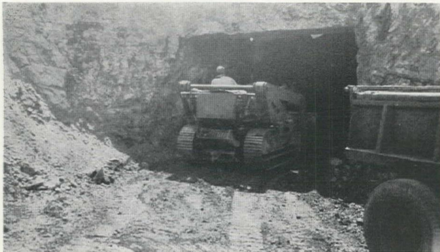
START OF DIGGING the reservoir under the roof. This loader is excavating an adit to provide access to the main body of earth.
