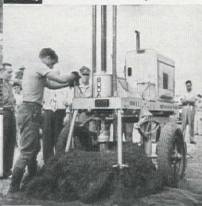
MODEL HBB 12" to 30" dia. - Depths to 16 feet
