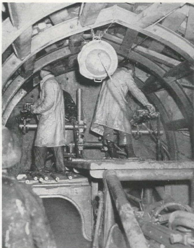
AT THE FACE in a typical Western tunnel with a column-and-arm type jumbo mounting two drills worked from the platform. Steel-rib supports and other features of modern tunneling practice are shown here.
