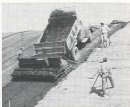
SPREADER BOX being filled from truck. Two rollers in rear of box assisted in controlling the thickness of the spread layer and in giving a light initial compaction to the mix.
