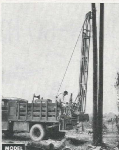
MODEL HBQ Diameters to 42" - Depths to 16 ft.
