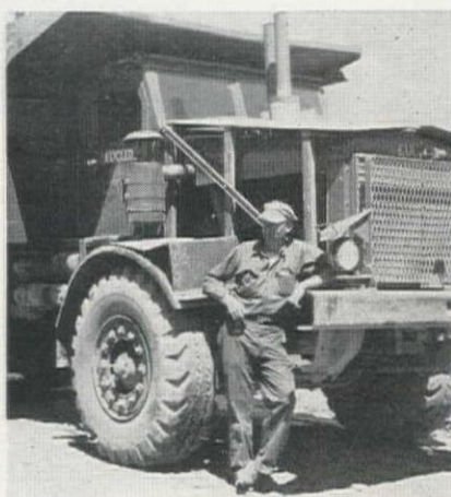
M. M. Moorehead, master mechanic for Utah Construction Co., at Bear River Dam near Jackson in Northern California. He's leaning against one of four big Euclid rear-dumps on the job, which are powered by the new NVH-1200 Cummins diesel engines (12 cylinder, rated at 400 hp.). Dam is being built for Pacific Gas and Electric Co.
