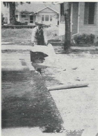
BUILDING PAPER assures neat joints between units receiving seal coat, keeps excess penetration emulsion off completed work.
