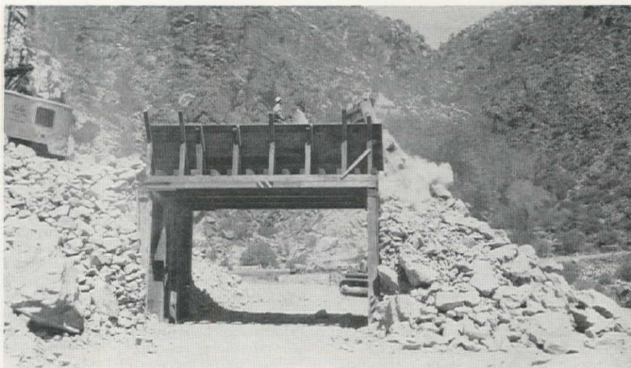
TO DISPOSE OF ROCK from the north portal of the tunnel without interfering with traffic on the existing highway, this bridge was built to get rock into the fill.
