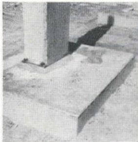
DETAIL of interior footing shows column base plate bolted and dry-packed in position.
