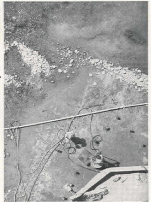
ABOVE—Jetted material ranges from fine clay to 1/4-in. gravel, is mostly sand as shown here.
