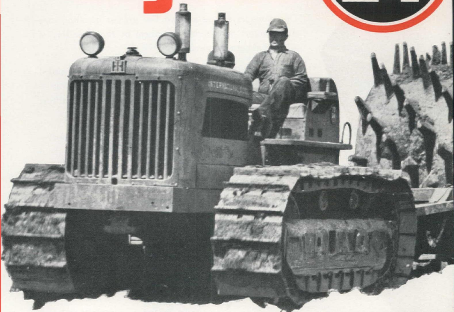
BREAKIN' SHALE ON THE BERM. TD-24 pulls a 60,000-lb. capacity spike-tooth roller, evening surface of uncompacted berms. Five TD-24s are literally "all over the place" on this big project's toughest jobs.
