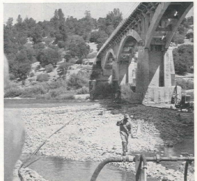
VIEW from mixer platform on left bank shows length of grout line, deterioration of caissons exposed by riverbed degradation.
