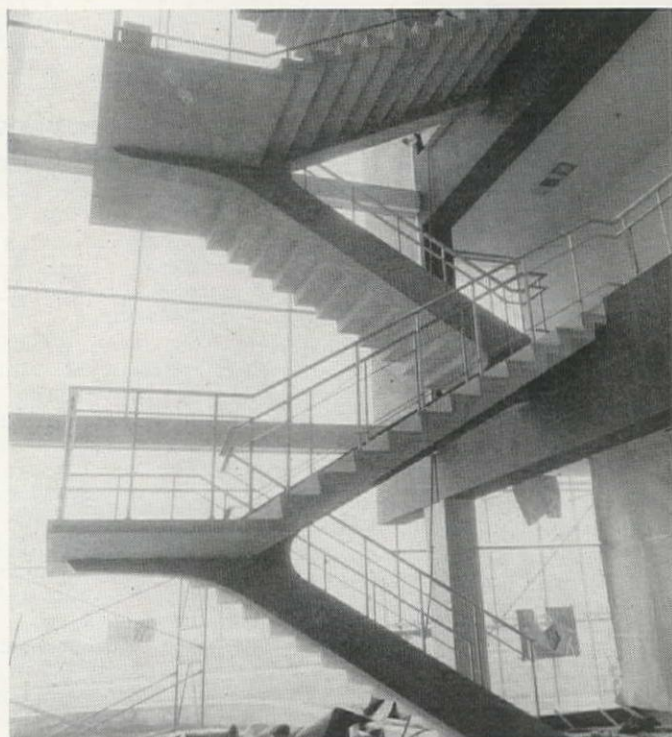
CUTAWAY of cantilevered central beam that extends upward four floors in jack-knife fashion. Reinforcing bar for each tread and riser was carried back and interlocked into this main beam.
