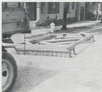
DRAG BROOM evens surface before street is opened to traffic. Slow speed is necessary to avoid jiggling of broom that would cause ripples in roadway.
