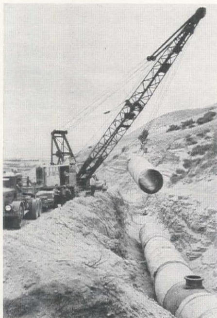
HIGH PRESSURE sections of the aqueduct totaling 5.49 mi. were of steel design.
