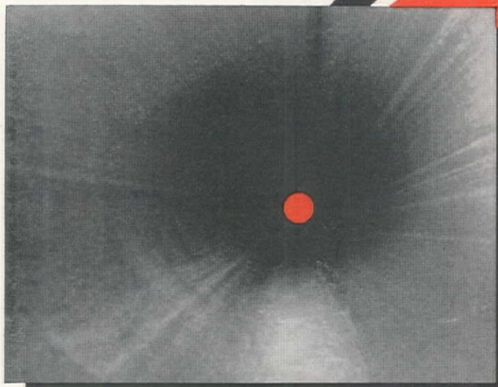
Old pipe reconditioned by cement mortar lining.
