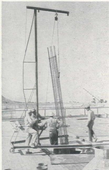
On the terminal reservoir of the Salt Lake Aqueduct project (see p. 80) Peter Kiewit Sons' Co. used this movable hand-hoisting rig to lower the cages of column reinforcing from the roof forming.
