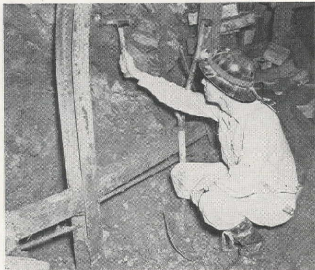
SHEARED and slicken-sided clayey siltstone was a common formation before the north heading passed through the Santa Ynez fault.
