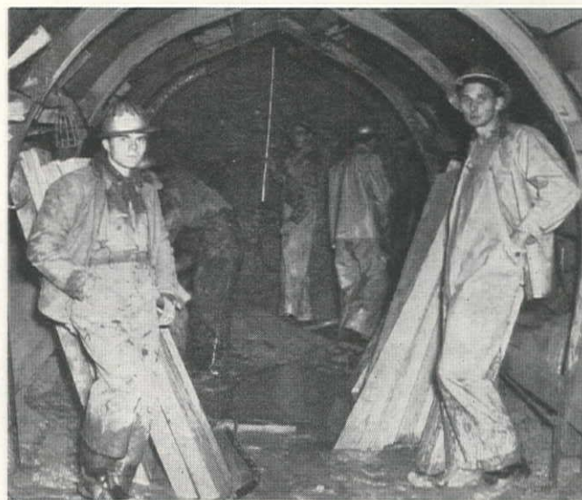
WATER in the north heading has never been a serious problem as to volume, but softens the shale and siltstone, as indicated, to make the tunnel floor difficult for track laying and maintenance.
