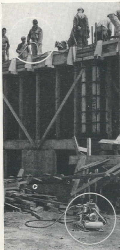
CP Hicycle Vibrator can be used anywhere within a 400-foot radius without moving generator. The motor is in the vibrator head—no flexible shafting is used. Vibrating frequency 10,000 V.P.M.
