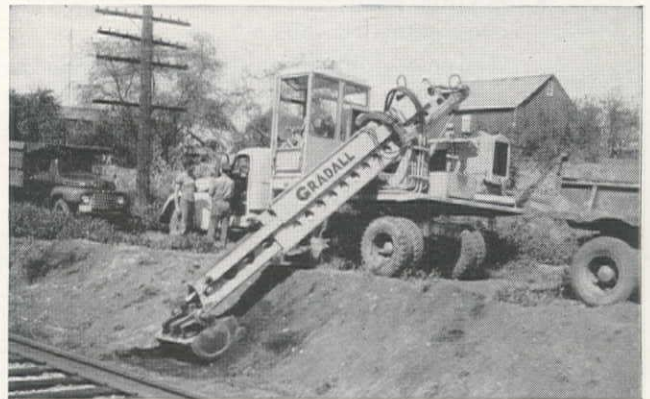
↑ In this restricted location working under low-hanging power lines the Gradall widens bottom and does a precision job following contours of this ditch.
