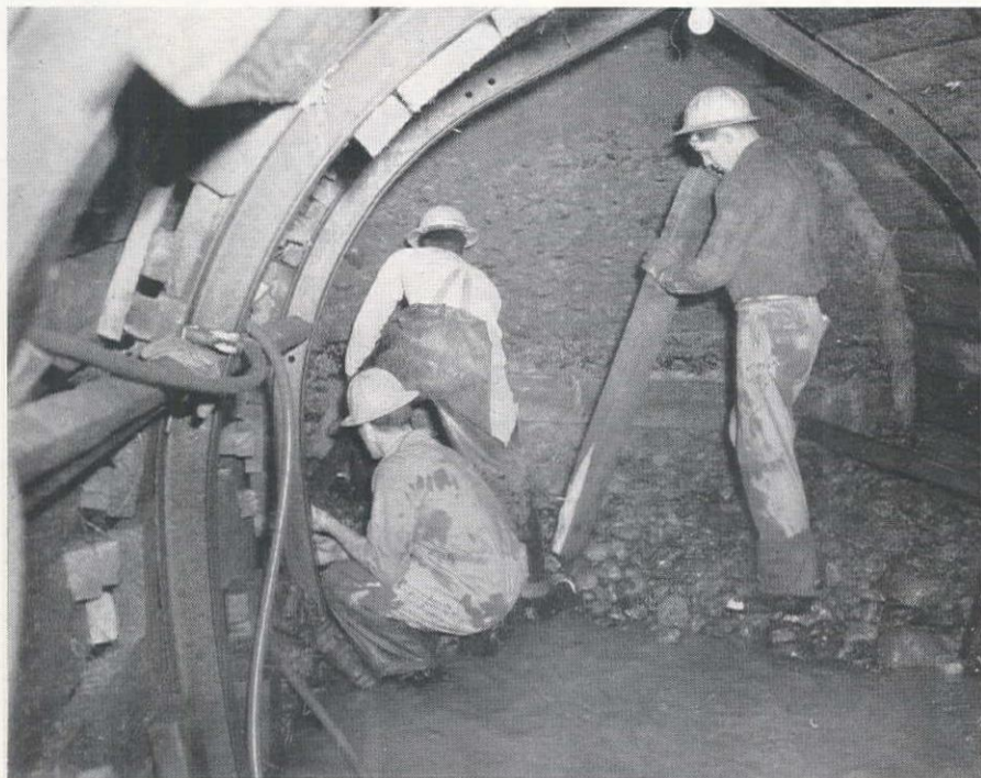
INSTALLING breast boards in the Portland interceptor sewer tunnel. Tunnel foreman Don R. Hawe stands by to hand sprag to workman bracing breast board against ring
