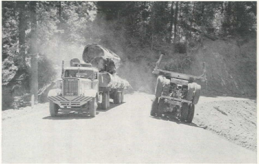
SUPER-ELEVATION design permits truck climbing hills under load to remain level while making curves, provides "super" for unloaded trucks traveling downhill.
