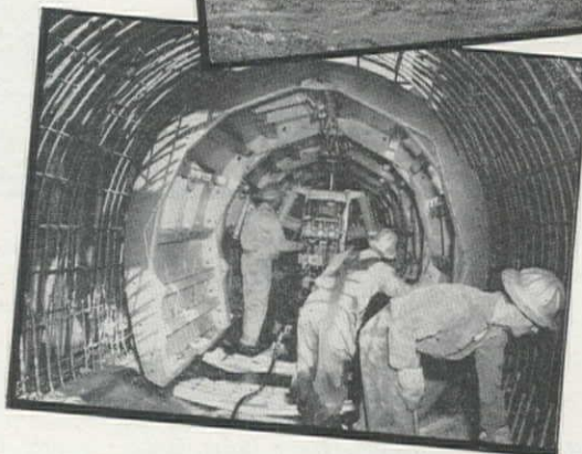
Oakland Outfall Sewer—NOBLE jumbo and 105" telescoping tunnel form, horseshoe type, Stolte, Inc.
