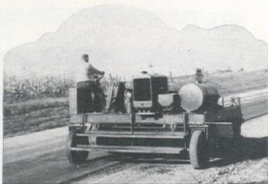
Rear wheels down and the machine is off to start the parallel course.
