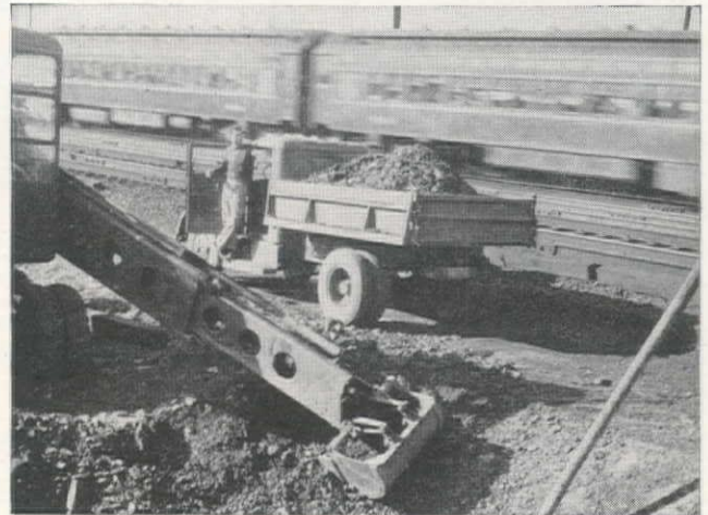
"Arm action" tilts the bucket laterally to dress side slopes of drainage ditch.
