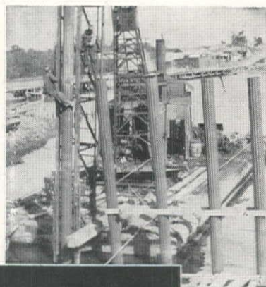
Looking at 65 feet of Monotube pile straight up from the water. Approximately 10,000 feet of 7 gauge and 3 gauge piles were used for the Tuckahoe River bridge, built for Maryland State Roads Commission by Tidewater Construction Company, under direction of Walter C. Hopkins, Deputy Chief Engineer.
