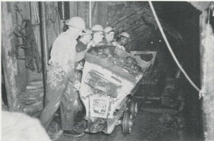
WELL RUBBERED UP for protection against flow of water, tunnel crew dumps muck car at shaft. Muck is removed from shaft by clamshell bucket.
