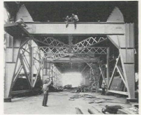
Test assembly in shops of Gunderson Engineering Corp., Portland, shows size of 25-ton gantry slated for McNary Dam Contractors. Four of these units, 35 x 40 ft., and 20 ft. high, will support Clyde Whirley cranes having a capacity of 35 tons at 75-ft. boom radius.
