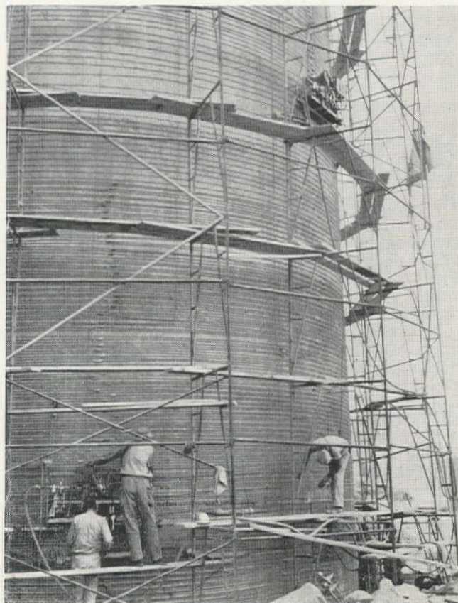
PRESTRESSING progresses with all four machines working on one silo. Second man of team (at left) handles telephone to coordinate jacking with crew on opposite side of silo.
