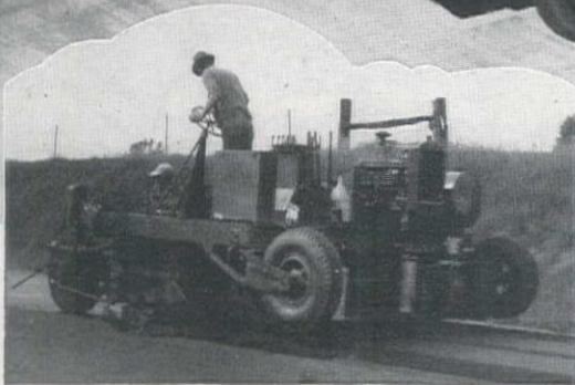
Laying a half-inch top course of hot mix.
