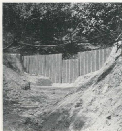
FIG. 4—Dam of Armco-sheet piling set in soil-cement in excavated trench.
