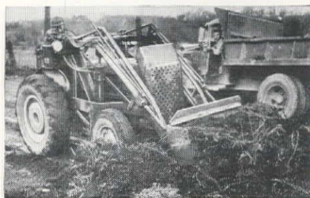
ROAD MAINTENANCE. Loading debris into trucks after grader has scraped ditch—cuts time and man hours. Shown on the job for a town in Pennsylvania.
