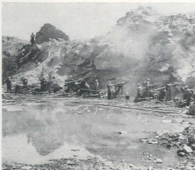
BATTERY of wagon drills receives real workout as they drill through hard "tombstone" granite for excavation of intake channel at Chief Joseph Dam. Over 1,500,000 lb. of powder was used to remove 3,500,000 cu. yd. of material.
