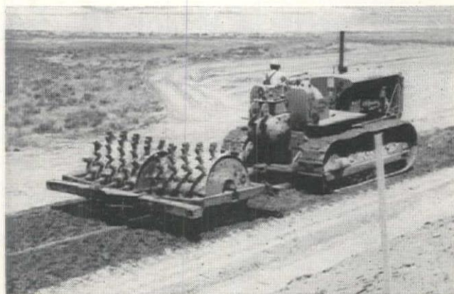
COMPACTING mixture with a sheepfoot roller loaded with sand.
