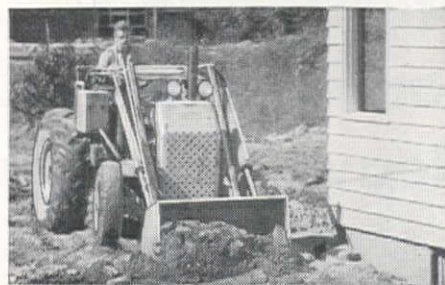
CONSTRUCTION WORK. Case "SI" Tractor completes grading and backfilling work at Bon Ami Homes project in New York. Moves over 200 yards per day.
