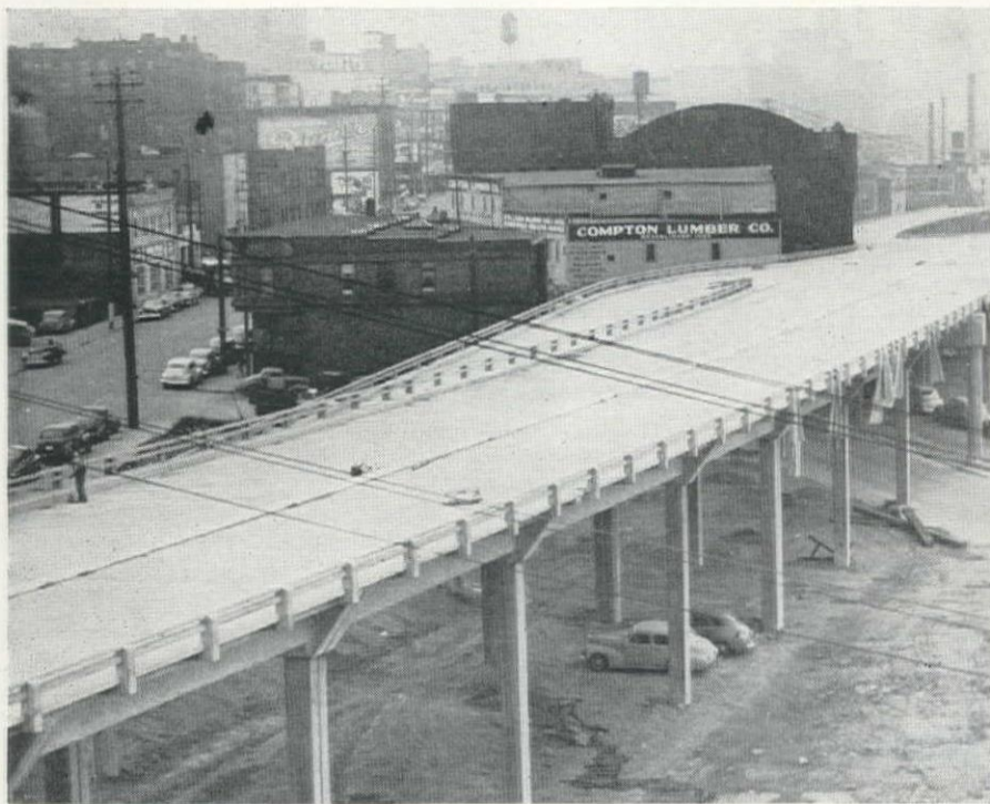
FOUR TRAFFIC LANES are accommodated by this finished section of viaduct, plus extra acceleration lane at ramp connections. Note split columns at ends of three-span rigid frame units.
