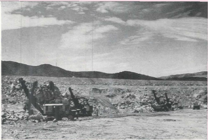
EACH of the four shovels wore out two buckets while working in "tombstone" granite during excavation of intake channel for Chief Joseph Dam powerhouse.
