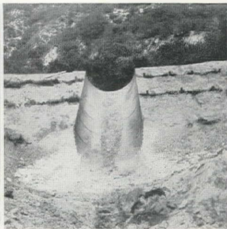
FIG. 12—Corrugated apron spillway over an earth dam.
