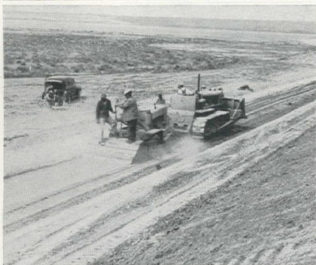
MIXING soil-cement with a rotary speedmixer pulled by a crawler tractor.
