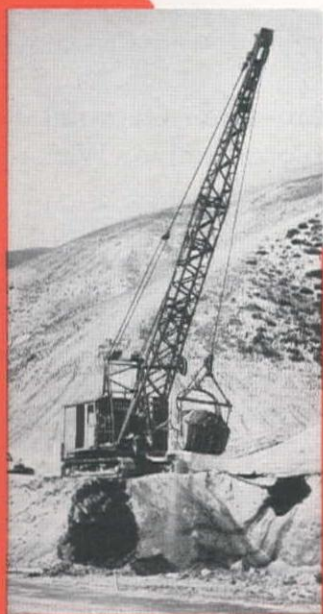
Northwest Drag-line excavates shoulder of highway. These units are in operation the year-round.
