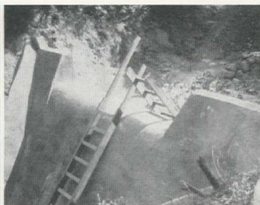
FIG. 2—Gravity dam of soil-cement (cement proportion slightly more than 10%).
