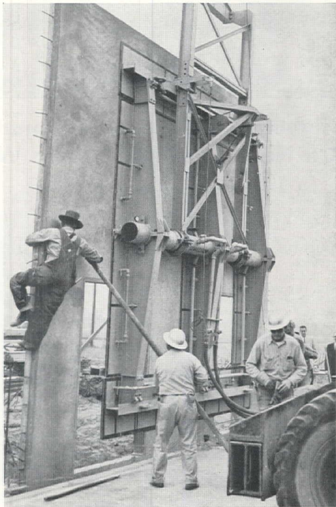
BRACING IS SECURED while vacuum lifter holds panel. Turnbuckles provide adjustment as required for transit alignment. Vacuum mats coinciding with panel openings are isolated from vacuum line by control valves.
