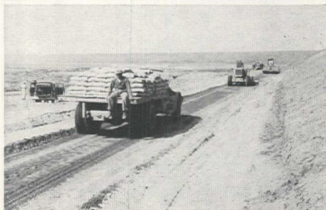
FINAL ROLLING over surface mulch by a flat-bed truck loaded with cement.
