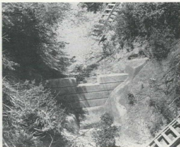
FIG. 11—Dam constructed of 12 x 12-in. precast concrete members anchored in soil-cement.
