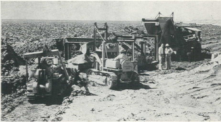
BACKFILLING by bulldozer constitutes final step in drain-laying operation, shown here in entirety. Trencher at right drags sled (center), from which hangs the working shield. Skip loader is charging gravel hopper from stockpile at right.
