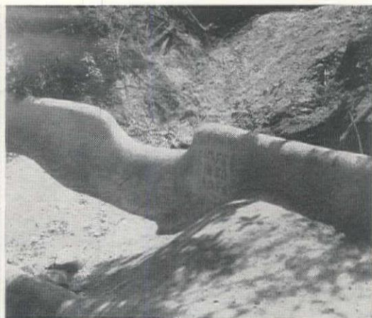
FIG. 9—Small gravity dam built up by gunite without forms of any kind.
