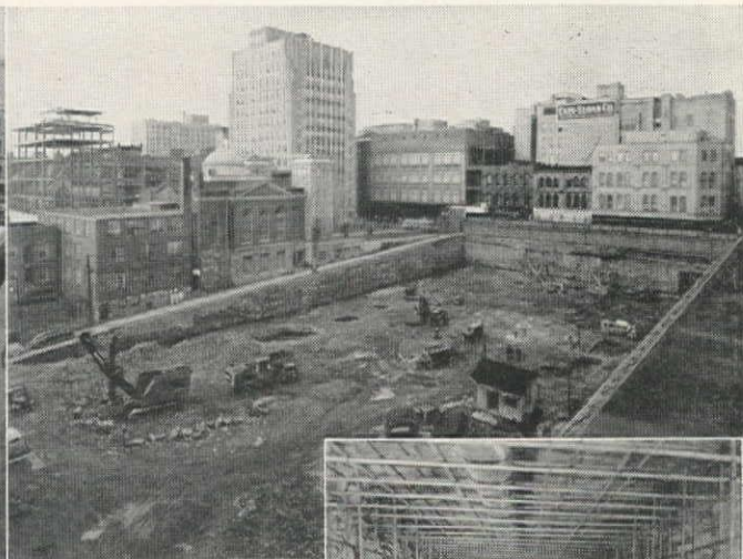
Final stages of excavation. Entrance to utility tunnel in right hand corner.
