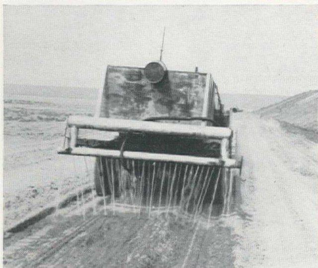
ADDING WATER to the layer from a 1,600-gal. water truck mounted on a flat-bed truck.
