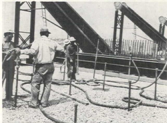
**TOP FORM** is placed and held down by heavy I-beam, and grout is brought up against the form. This form has a lower facing of screen and cloth to permit escape of air and surface water, while it is vibrated.
