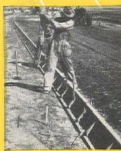
Blaw-Knox Steel Road Forms are self-aligning, easy to set and strip.
