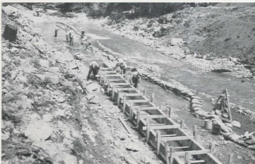
Inlet form section, weighing 5 tons, arrives at culvert location and is moved into place by crane. Inlets are flared with 24-ft. opening decreasing to 20-ft. diameter.
