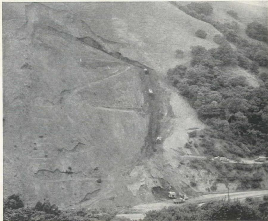
VIEW of clean-up operations on the Tunnel Road slide in late April 1951. Slide began December 9, 1950, temporarily blocking four-lane highway between Oakland and Orinda, Calif. Loose material from the estimated 330,000-cu. yd. slide was bulldozed down the slope to be hauled away for use as road fill.
