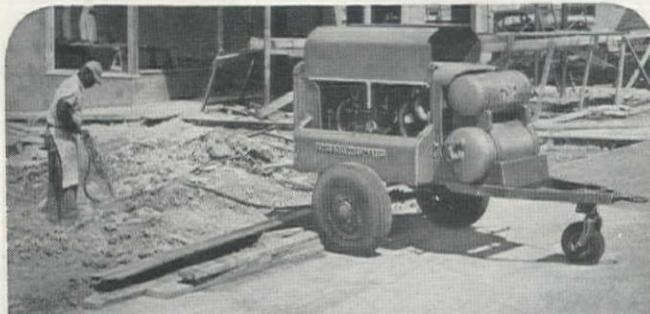
**CP PORTABLE COMPRESSORS**, notable for dependability, low maintenance; available in gasoline and Diesel driven models, 60 to 600 c.f.m. CP Gradual Speed Regulator minimizes engine wear, saves 15% to 35% in fuel.
