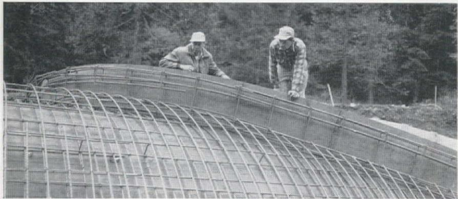
TOP—Workmen put finishing touches on form. Doors along center of form are for placing concrete below that level. Doors are closed as concrete is placed above that point.
