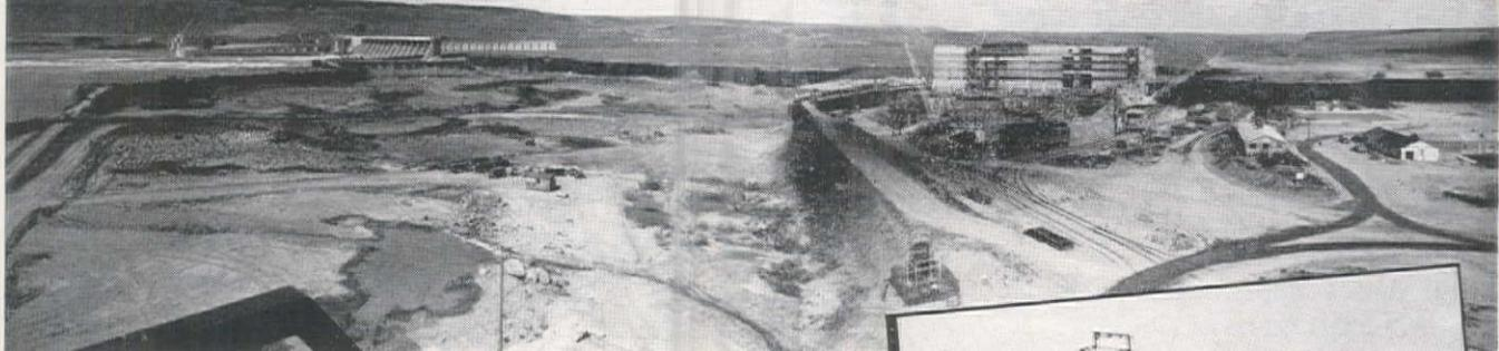
**Noble plant batches 958,000 cu. yds. of concrete for first and second sections at McNary Dam; now batching 816,000 yds. for third section.**
