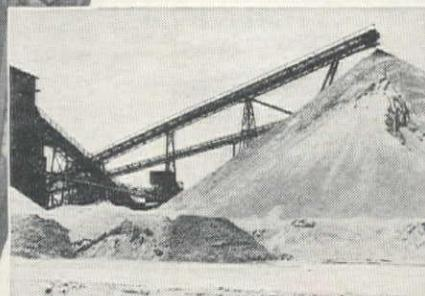
GRAVEL PLANT that handles up to 150,000 tons of wet sand per year. The "U.S." belt on the outdoor installation above has been working steadily on this job for over 8 years and is still going strong.
