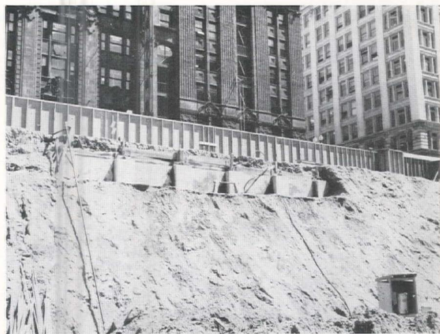
AS A TEST, excavation along the wall line was carried down one-half a floor and a 5-in. gunite wall shot directly against the ground in these five panels.
