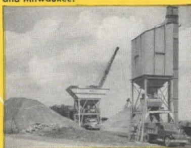
Blaw-Knox Portable Aggregate Batching Plants and Portable Bulk Cement Plants on the Pennsylvania Turnpike.
