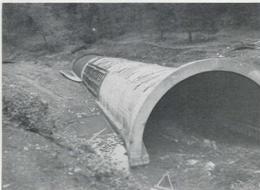
View of partially-completed culvert shows stages of construction. First section, in foreground, is completed. Outside forms at second section will be moved into position for third section where reinforcing steel has been set. Note that water is already flowing through the culvert.
