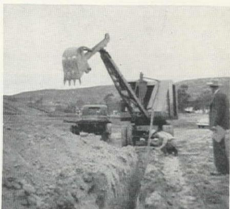
TO HANDLE trenching for new sewer connections on the Brookside housing project in San Diego, subcontractor H. J. Wulf of Long Beach drove in a Schield Bantam Back Hoe mounted on a G.M.C. 6 x 6 truck. The Back Hoe, working in sandstone material, was used to dig 5 to 6-ft. depths and averaged 100 ft. per hour.
