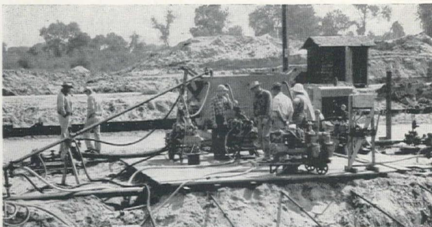
**BATTERY OF FOUR** secondary pumps delivering grout into pipe lines. An important characteristic of the grout is its ability to maintain the sand in suspension in long delivery lines.
