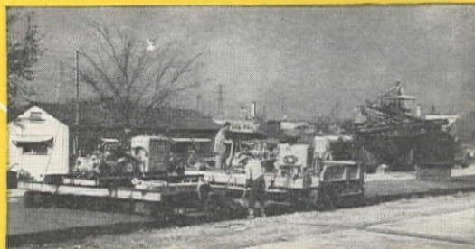
Blaw-Knox Paving Spreader and Finishing Machine at work on Edens Superhighway between Chicago and Milwaukee.
