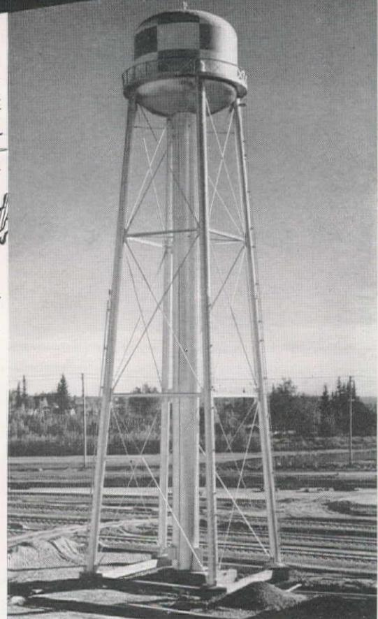
As part of the rehabilitation program, a 90-acre area in Fairbanks was cleared and a complete new terminal yard was constructed. To serve this new yard, a 50,000-gallon Horton elevated water tank, and two Horton 2,500-bbl. diesel oil storage tanks were erected. Together they provide modern, long-lasting storage facilities that assure efficient year 'round service.
