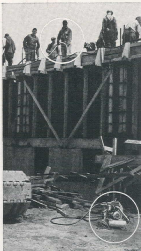
Homelite Generator on ground powers vibrators on top of forms.
