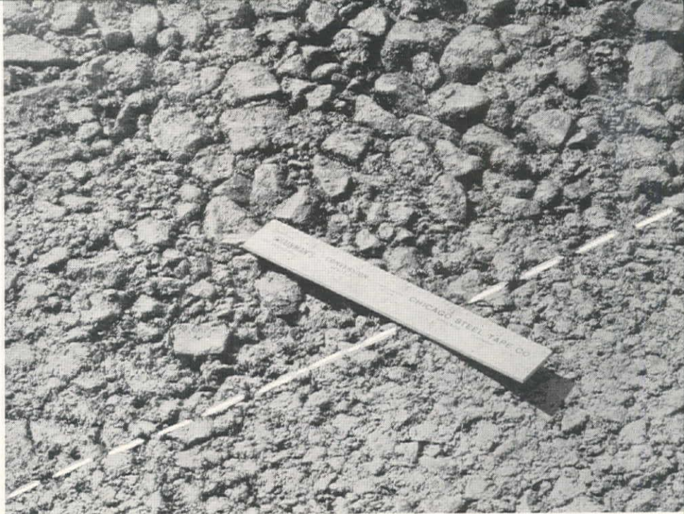
SURFACE OF PAVING for a residential street shows distinction between base (above dashed line) and top course. This asphalt pavement had been in place two days when picture was taken.
