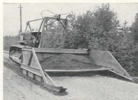
BASE COURSE SPREADER used by Williams Equipment Co. and Reed & Martin, Inc., on the Fairbanks-College paving contract.
