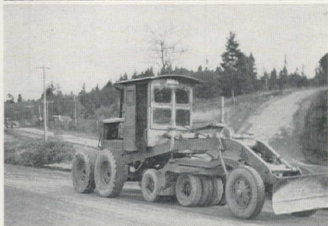
FINISH compaction of cement-treated base was accomplished with a 9-wheel Bros roller suspended on the circle of a motor patrol.
