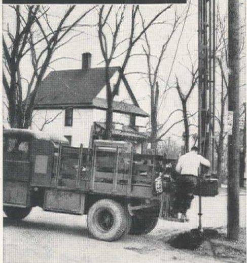
Fine control of tower adjustments permits working in close quarters.
