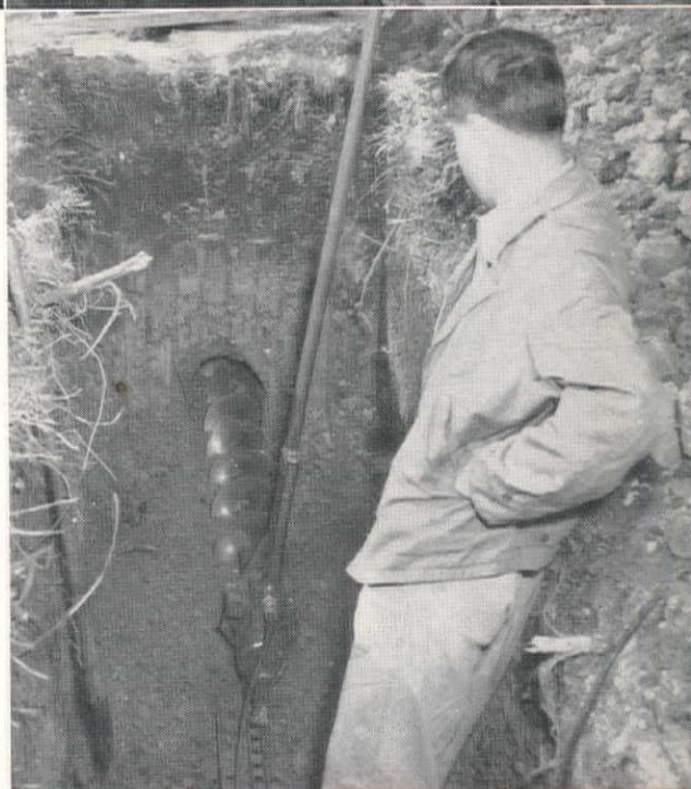
EARTH BORING TOOLS — Thor pneumatic drills for driving augers or "fish tail" bits in laying of gas and water lines, electric conduit and cable under paved roads, alleys, driveways, etc. Also widely used for down-hole drilling of post holes, trenches, etc.
