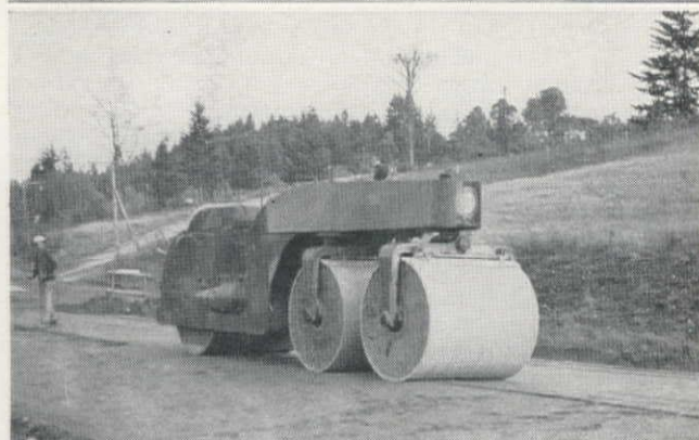
BREAKDOWN compaction was carried out by a 13-ton 3-axle Buffalo-Springfield roller.
