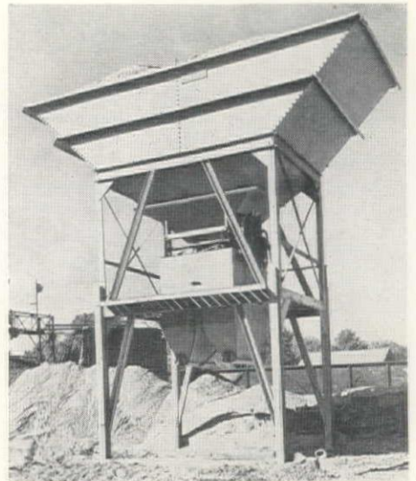
TWIN weighing batchers discharging a double charge of aggregate into the batch truck speed up concrete paving work on highways and airports.
