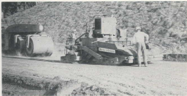
LAYING the first lift of cement-treated base. Roller closely followed Barber-Greene asphalt paver.
