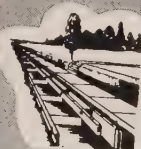
STEEL STREET FORMS
