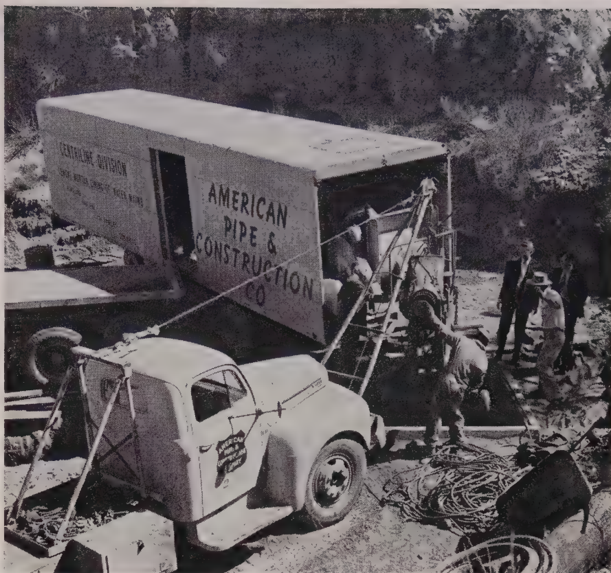
MORTAR for lining was supplied by a plaster-type mixer mounted in mobile van, which also housed generator and supplied storage space for sand and cement. Mortar was dropped through manhole into buggy inside pipe. In this view, lining machine is being lowered into pipe.
