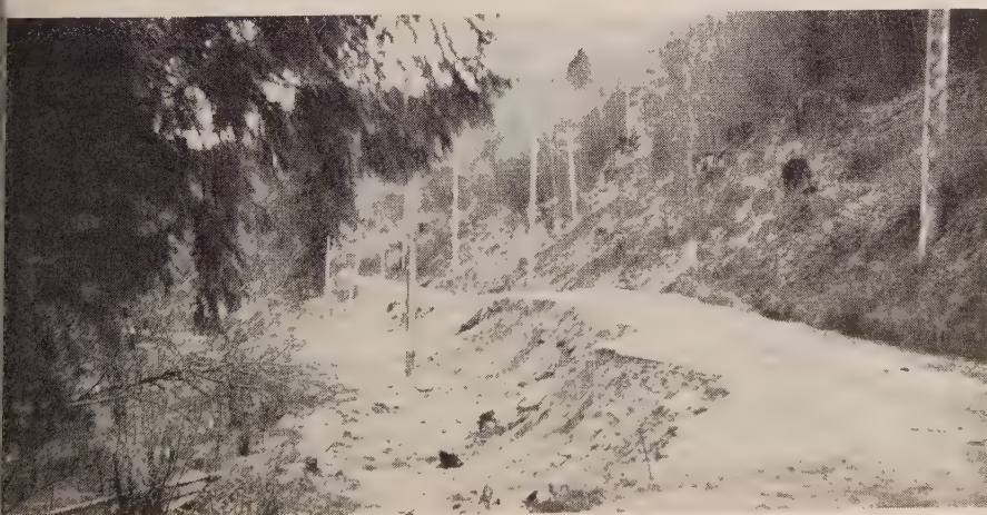
20-FT. vertical displacement was found at the top of the steel side-hill slope. System of transverse ditching removed water at the base of this slip (drawing above). Section of road as it appeared shortly after the earthquake is shown below.
