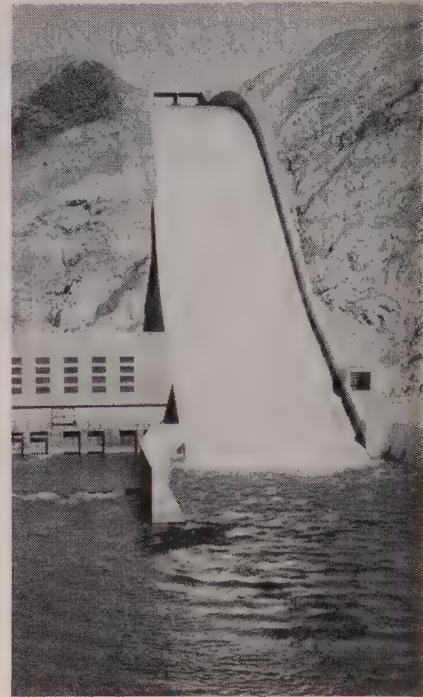
ANDERSON RANCH SPILLS —A cascade of water plunged out of the Anderson Ranch Reservoir near Boise, Idaho, April 10 when Bureau of Reclamation engineers released the discharge for the first time over the 330-ft. high concrete spillway. At the left of the spillway is the 40,500-kw. power plant, in which the first of three 13,500-kw. generators is turning.
