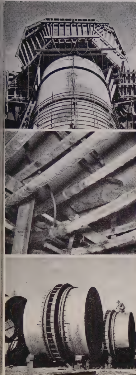
TOP—Special forms were used where penstock passes through dam's longitudinal contraction joint to make joint normal to the pipe.
