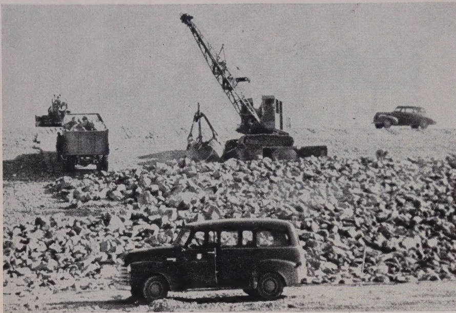
FOR PLACING RIPRAP , tractor equipped with winch lowered end-dump trucks down slope on plank mat. Orange-peel bucket dragline supported on wedge-shaped Navy pontoon sections then "hand-placed" the rock. Dragline moved extra pontoon to provide continuous level platform.
