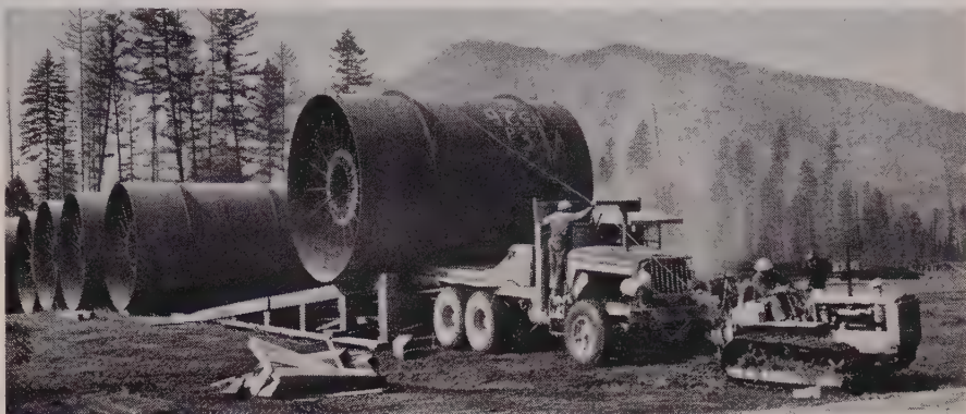
SMALL TRACTOR LOADS 13 1/2-FT. PIPE. The fabrication yard for penstocks at Hungry Horse Dam was 3 1/2 mi. away from the dam site, so the big pipe sections had to be trucked to the site as they were assembled. A small tractor was used to roll the 20-ft. long sections up an inclined ramp onto a timber cradle mounted on the flatbed trucks.
