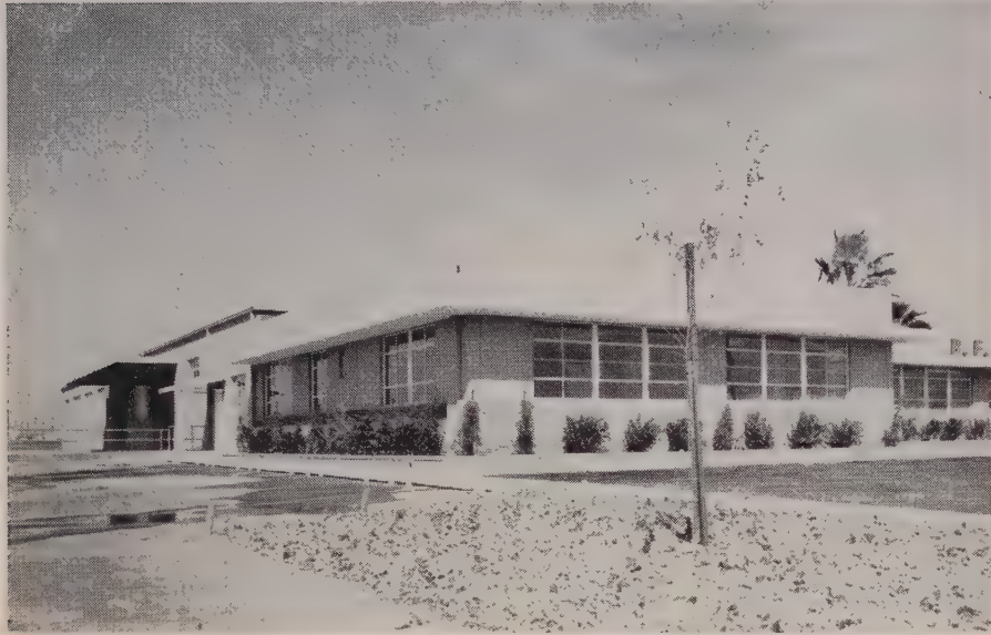
COMPLETED building has undersides of panels (as precast) used as exterior wall face.
