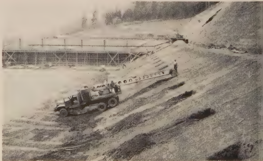
TWO ROWS of holes, 5½ ft. square, 3 ft. deep and running around the entire reservoir, are being excavated for foundations of 500 columns to support roof.
