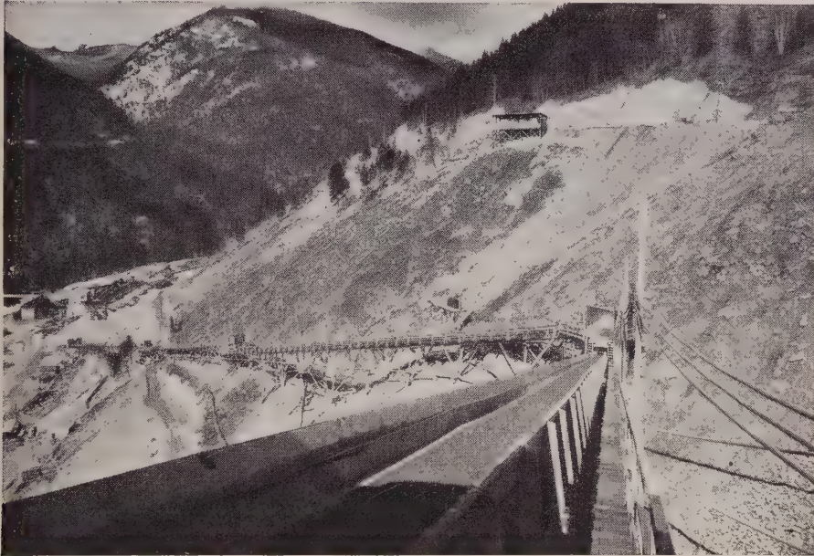
Aggregate for batching plant at Hungry Horse Dam is carried 1600 feet up the canyon wall by conveyor, driven by reliable G-E 100-hp motors in wooden sheds at intervals of 250 to 300 feet.
