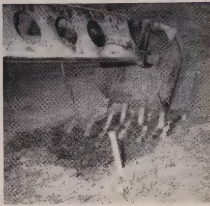
BUCKET with teeth pointing downward cuts neat square holes requiring a minimum of hand finishing. Operator can control precisely the point of entry of the bucket teeth.
