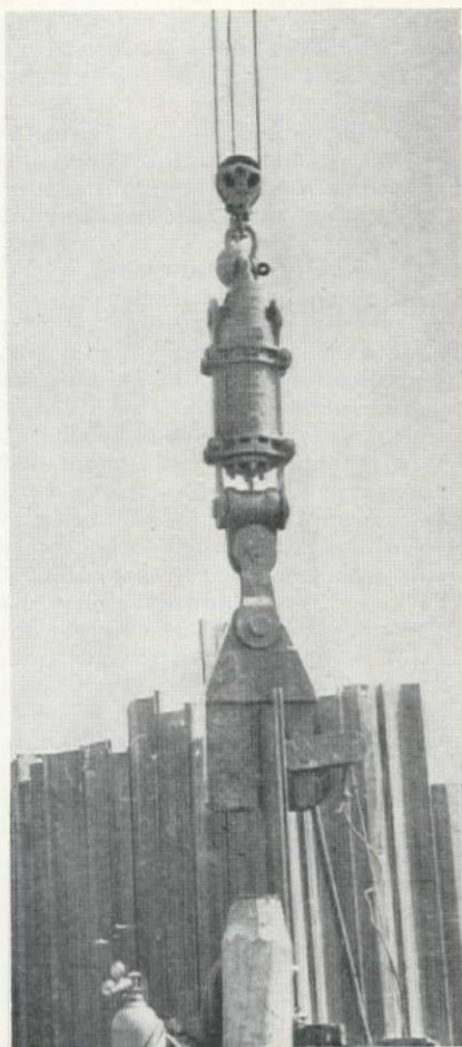
PILE EXTRACTOR with gripper was especially designed by the contractor for the job.
