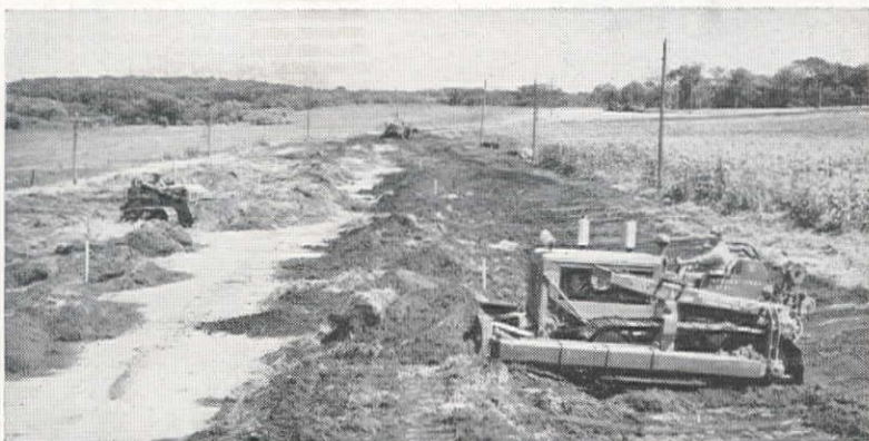
INTERNATIONAL CRAWLERS MAKE SNOWTRAPS —deep snow ditches to keep the highway from drifting over in winter. A TD-9 and two TD-18's are on this job. One TD-18 has 4,500 hours in three years, the other has 9,600 hours in four years!
