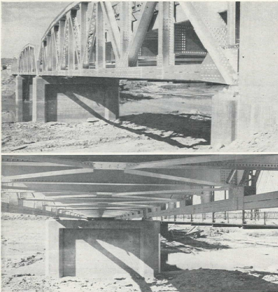
RE-ERECTED BRIDGE viewed from near south abutment. Footings for reinforced concrete piers and north abutment are founded on solid shale while south abutment is supported on timber piling.
