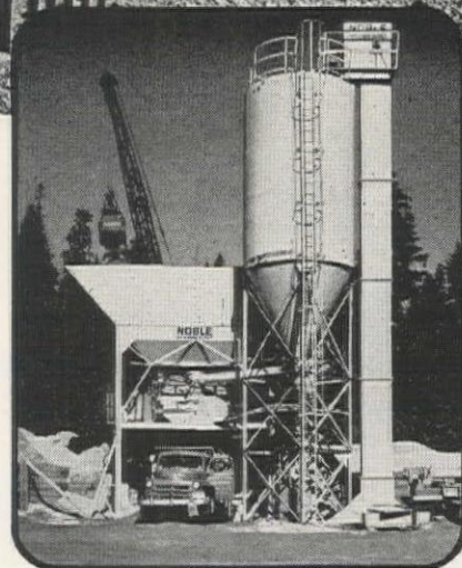
NOBLE CA104 semi-automatic batching plant, with 500-bbl. bulk cement silo, batching for Snoqualmie shed.
