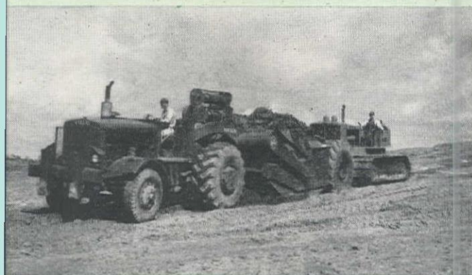
Euclid Scraper ... 15.5 cu. yds. struck ... 275 h.p.
