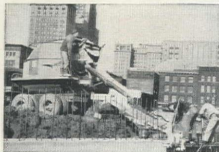
One of Arundel-Brooks' 6\frac{1}{8} cu yd agitators pouring a retaining wall at General Sam Smith Park, being built to relieve traffic congestion at Light and Pratt Streets, Baltimore.
