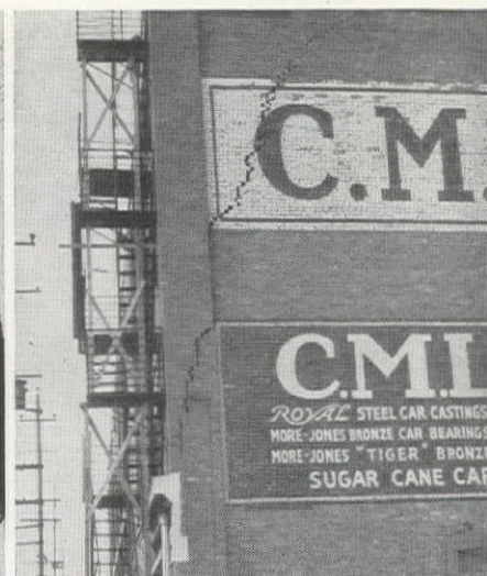
LEFT—Unsupported by any adjoining building, the corner of this structure moved out from under the roof the distance indicated by the crack.
