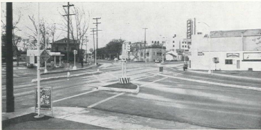
A TOUGH intersection problem solved with installation of traffic islands, traffic signals and the "walk-wait" pedestrian signals so essential for safety on the wide lanes. The location is on the Divisadero Street widening project.
