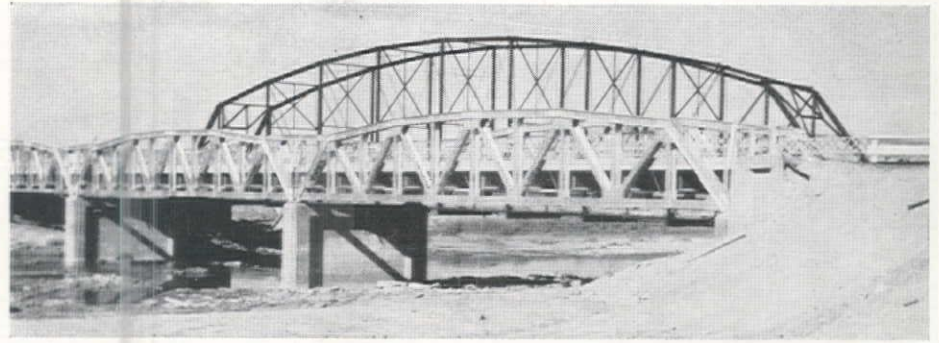
THE BRIDGE re-erected at new site on new substructure. Old bridge in background was later torn down.
