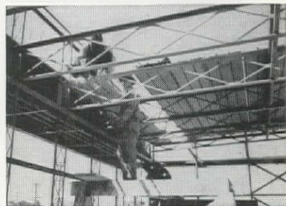
30% Less Steel required for this garden shop, built with welded design for Sears Roebuck & Company, Compton, California. Construction cost cut from $30,000 to $20,000.
