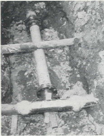
LEFT—Water and sewer lines fractured with pollution inevitable unless break is uncovered.
