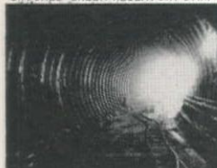
SHIELD DRIVEN SECTION CHICAGO SUBWAY
