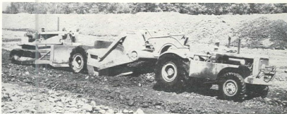
K. C. DACK , owner of his own construction outfit at Milton, Ore., has one of his Caterpillar tractor-scraper combinations hauling rock for a dike on the Walla Walla River.
