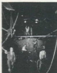
HAND MINED SECTION CHICAGO SUBWAY
