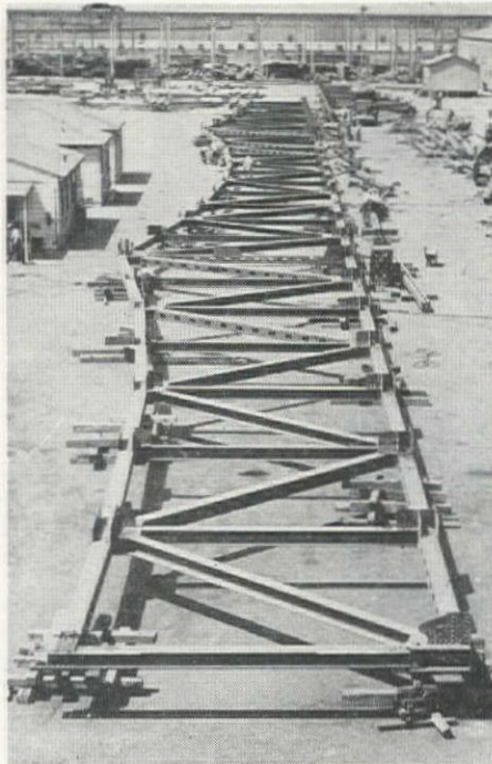
CHECKING A BRIDGE TRUSS
