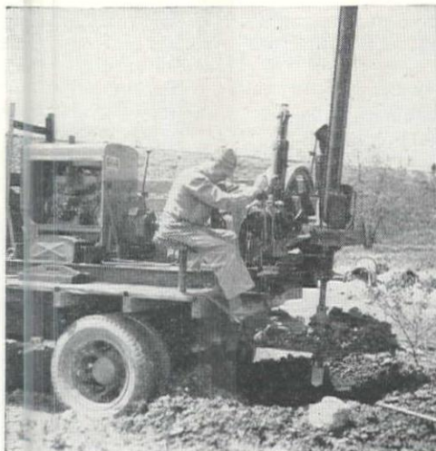
HBR Earth Drill drilling large diameter hole.
