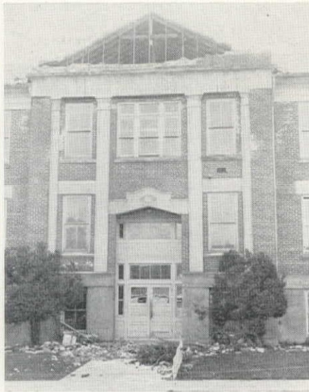
LEFT—Unanchored roof and ceiling beams over the stage of Puyallup high school auditorium slid off supporting masonry walls and crashed to floor, causing $100,000 damage.
