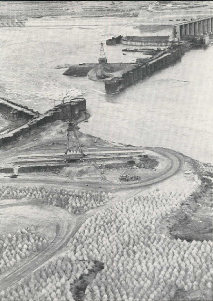
BIRD'S-EYE VIEW from Oregon shore as closure operations begin. "Tent village" is tetrahedron storage area. Note head-tower in foreground for 1,400-ft. cableway across the gap to tail-tower on low-water island. Both towers were movable, with about 300-ft. travel, for accurate spotting of dumped "tets".
