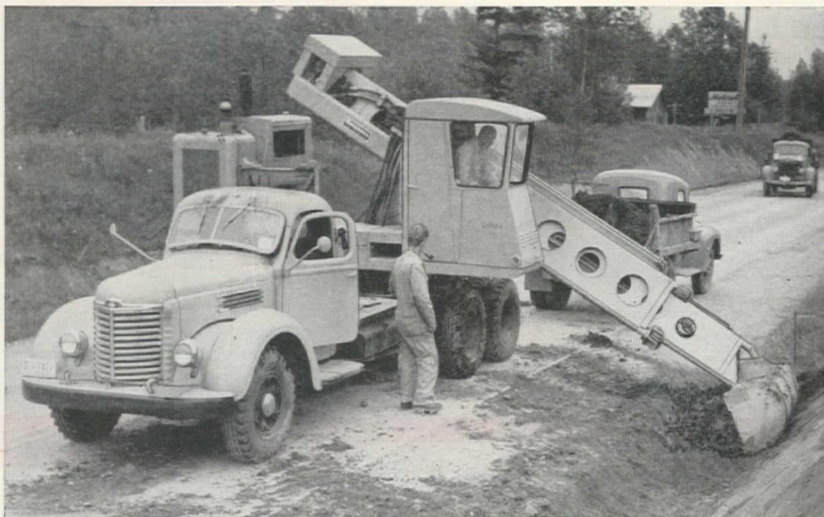
Gradall ditching and cleaning slopes near Bellingham, Washington
