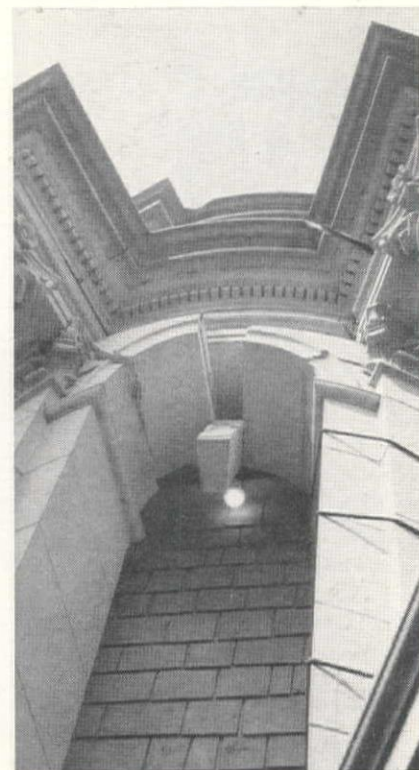
IN THE CAPITOL DOME at Olympia, erected in 1925, unanchored keystone dropped and column caps broke away. It takes strong mortar, steel and concrete, besides stone, to make such structures earthquake-resistant.
