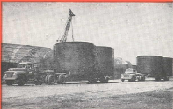
Steel Cylinder and reinforcing cage for concrete pipe sections on the way to project 28 miles away.
