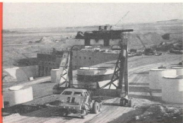
Huge pipe carrier converted, under direction of Chief Engineer Kenneth James, from a tank retriever at a cost of $65,000 to handle the tremendous size and weight of largest precast pipe sections.
