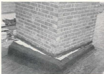
MANY UNREINFORCED masonry chimneys were fractured and rotated far more than this one, which gave way at the flashing point above the roof. A competent designer could have avoided this weakness.
