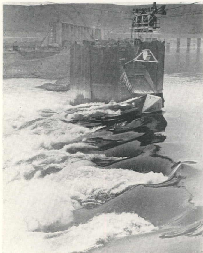
BIRD'S-EYE VIEW from Oregon shore as closure operations begin. "Tent village" is tetrahedron storage area. Note head-tower in foreground for 1,400-ft. cableway across the gap to tail-tower on low-water island. Both towers were movable, with about 300-ft. travel, for accurate spotting of dumped "tets".
