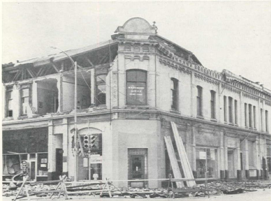
TOP —Poorly anchored brick veneer was knocked off Seattle structure. The obvious lesson here is that building facings must be designed to resist a reasonable amount of horizontal force.
