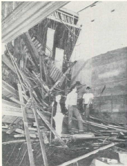
LEFT—Unanchored roof and ceiling beams over the stage of Puyallup high school auditorium slid off supporting masonry walls and crashed to floor, causing $100,000 damage.
