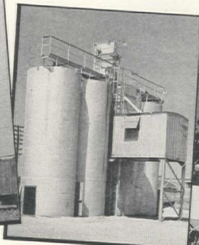
Snoqualmie Pass — Semi-automatic 100-ton plant with 2000-cu. ft. cement silo, batching highway concrete.
