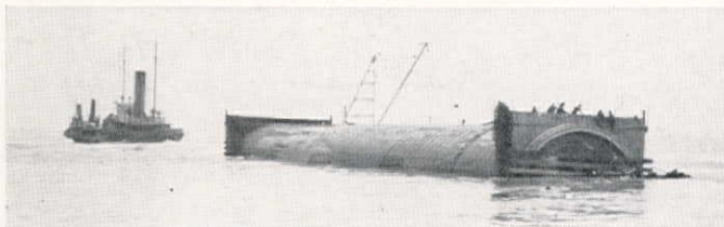
First subaqueous tunnel in the West built of pre-cast concrete sections, towed to position and sunk—later named Posey Tube.
