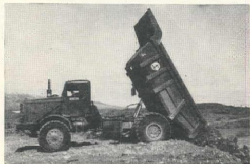
Above, a Rear-Dump "Euc" places 22 tons of earth and rock fill during construction of Chief Joseph Dam at Bridgeport, Washington. Other Euclids of this type have capacities of 10 to 34 ton payload, 125 to 400 h.p.
