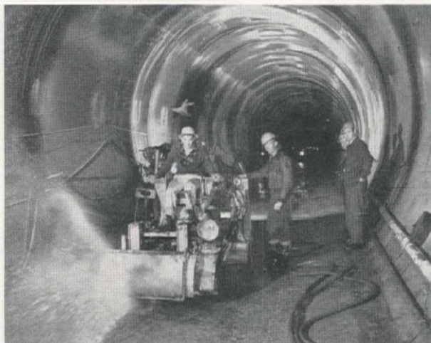
ROUGH and pitted invert in a power-plant tunnel causing serious reduction in flow was an unusual problem solved by building an electrically-powered machine for wet-grinding the concrete smooth.
