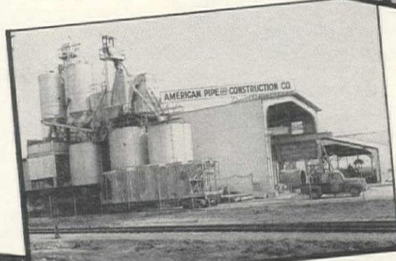
Pipe — 150-ton, 4-compartment plant with two 2000-cu. ft. silos, first of 5 for Amer. Pipe & Construction.
