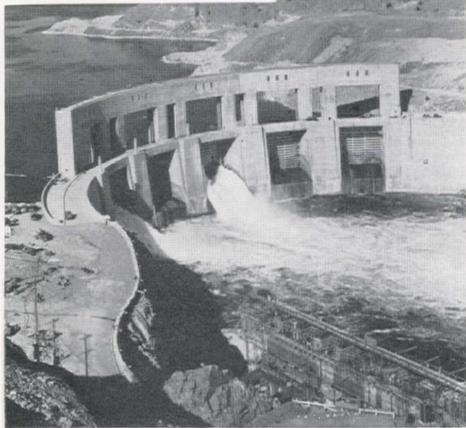
Parker Dam nears completion after setting record-depth foundation 250 ft. below Colorado River.
