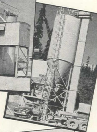
Snoqualmie Pass — Semi-automatic 100-ton plant with 2000-cu. ft. cement silo, batching highway concrete.
