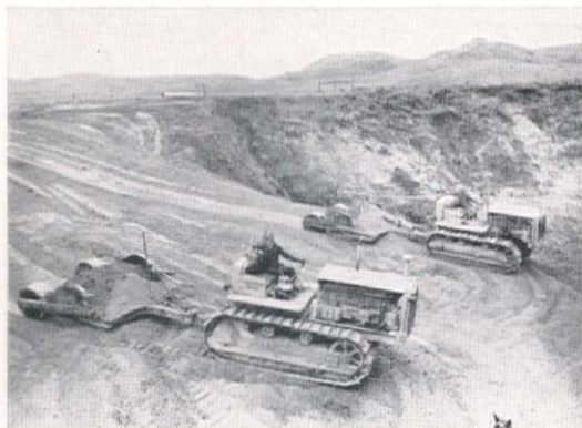
Tractors begin to pull carrying scrapers, which subsequently grew in size and were equipped with rubber-tired wheels.
