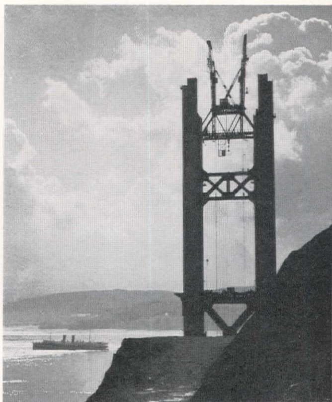
Steel goes skyward for the record-breaking 4,200-ft. Golden Gate Bridge span, with cable spinning active during 1936.
