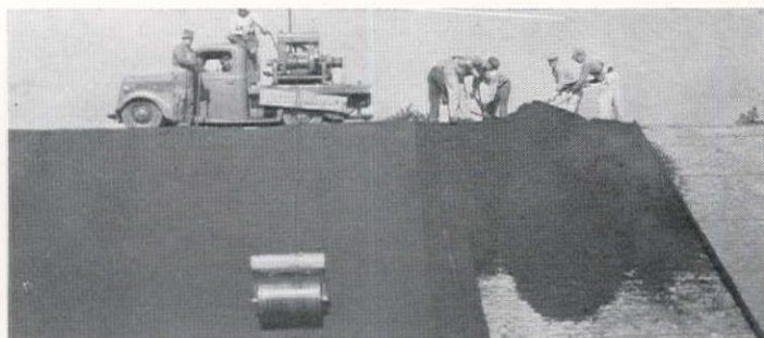
Asphalt lining for flood channels advances from experimental stage to full-scale construction at Los Angeles.
