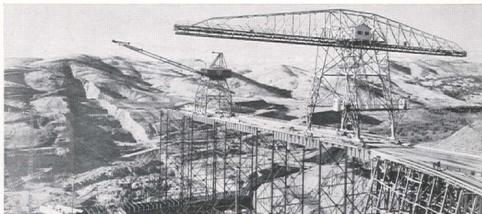
Bids opened for Friant Dam (shown in excavation stage) where construction plant presented excellent example of trestle and gantry-crane concrete handling system.
