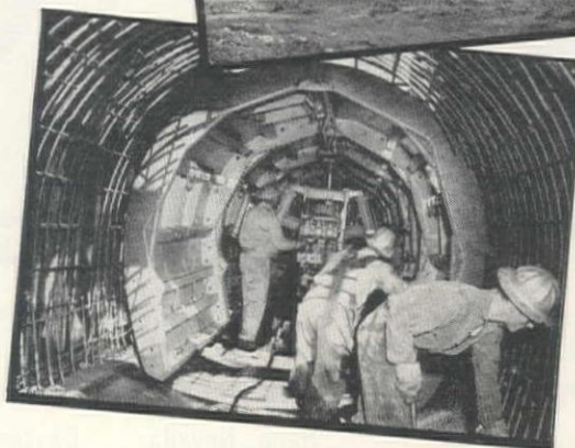
Oakland Outfall Sewer—NOBLE jumbo and 105" telescoping tunnel form, horsehoe type, Stolte, Inc.
