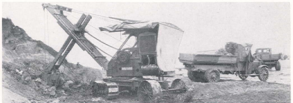
Horsepower on-the-hoof for hauling and excavation work being replaced by dump trucks and gasoline engine powered shovels.
