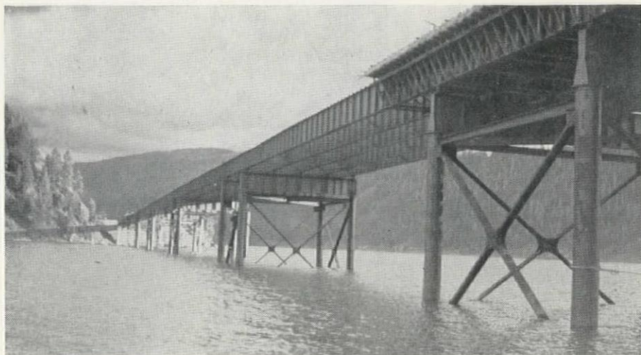
THIS LOCATION was studied for a suspension span, a pontoon bridge and a rockfill causeway, any one of which would have cost almost $2,000,000 as compared to the bid price of $871,155 for the unique design finally developed.
