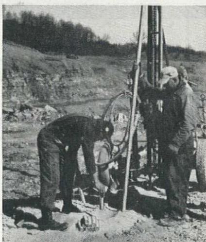
Du Pont "Red Cross Extra" 50% and "Gelex" No. 2 are loaded into wagon drill holes. And Du Pont "MS" Delay Electric Blasting Caps are used in the primers.
