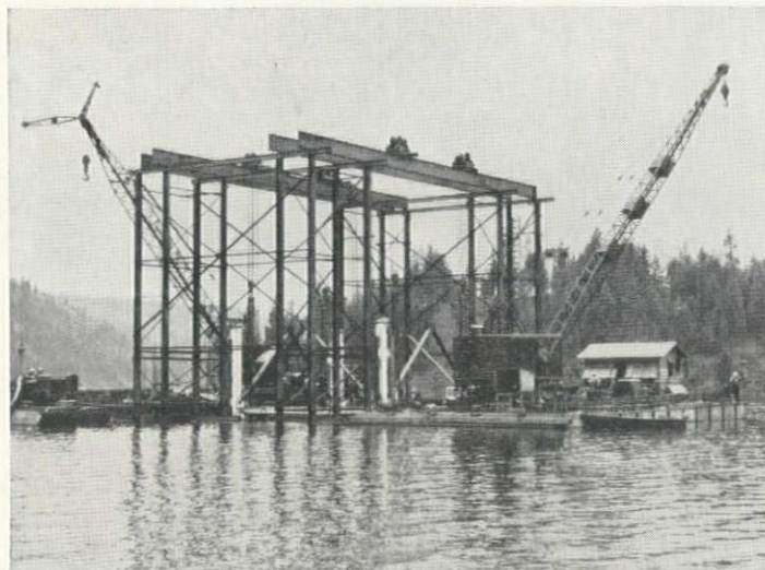
TOWER 6 being erected from pile falsework, showing the winches used to support and lower the 30-ft. square sections as they were assembled.
