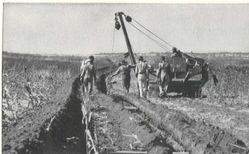
This line was protected in 1927 with Barrett Pipeline Enamel. When taken up for relocation 16 years later, the steel was found to be free from corrosion.
