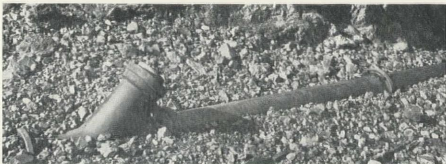
CLOSE-UP of 6-in. "Y"-branch cleanout and mechanical joint sealed with rubber gasket, on the Belvedere Island beach outfall sewer.
