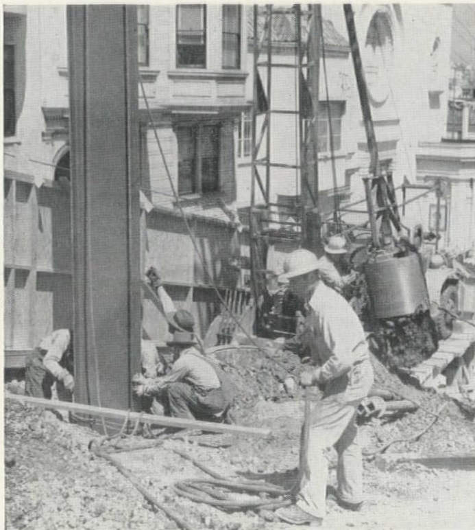
SETTING soldier beams at the east approach. Rig in background is drilling holes for the beams a number of feet below final sub-grade.
