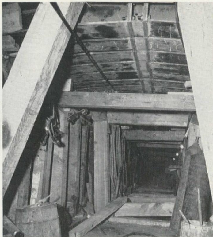
TOP HEADING at east approach with arch ribs in position. Excessive settlement necessitated pouring concrete footings from drifts.
