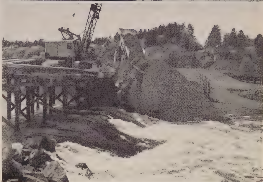
TOP—Widening east half of the dam. Note how bed capacity of Euclid trucks was increased 3 cu. yd. by bolting timbers to sides.
