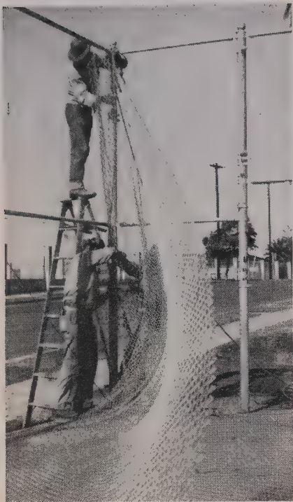
ERECTION of 12-ft. high wire fence. Fabric is #11 gauge, 1\frac{3}{4} mesh, stretched taut and hung with stretcher bands. Maximum post spacing is 10 ft. Provision is made for expansion in the top fence rail.
