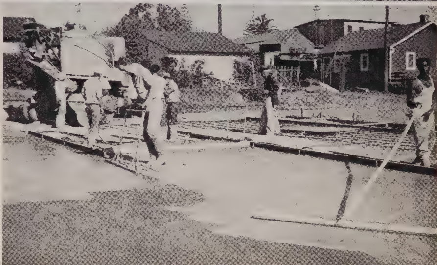
TOP—Concrete delivered by transit-mix truck is delivered into a gasoline buggy which rides over plywood panels to dumping location. BOTTOM—Tamping and floating the last batch of concrete delivered from buggy before applying lampblack to surface.
