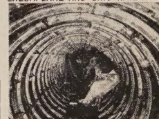
SEWER TUNNEL CUYAHOGA HEIGHTS, OHIO
