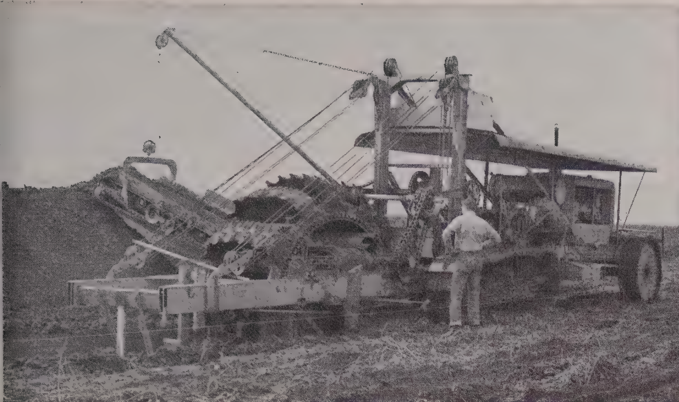
WHEEL-TYPE TRENCHERS dug the 64-in. wide trench to depths of 8½ ft., greater depths requiring trench hoe work. Midget bulldozers, built to order for the job, were equipped with 44-in. wide blades and drags to work the trench bottom to a smooth surface at grade.
