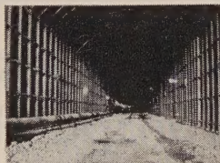
HIGHWAY TUNNEL PENNSYLVANIA TURNPIKE
