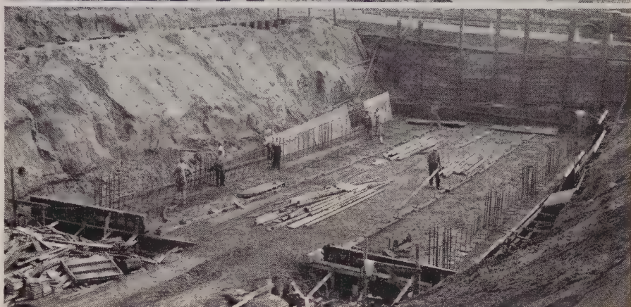
A SPECIAL dewatering system controlled excessive groundwater during construction of the 24th Street undercrossing. Foundation conditions before dewatering are shown at top. Bottom view is after excavation was sealed with membrane waterproofing and base slab.
