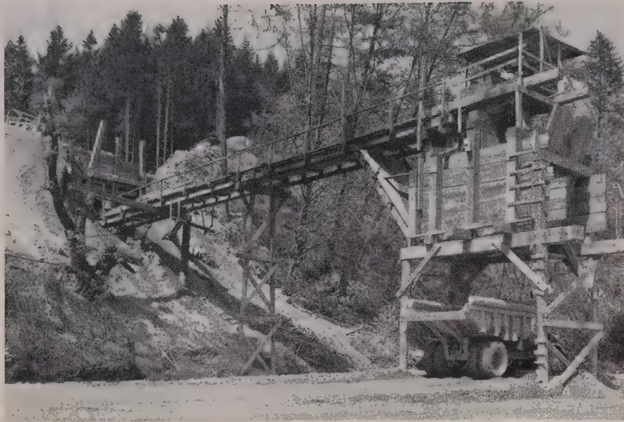
DURING DIRT MOVING operation, a conveyor belt was built across railroad tracks at the borrow pit. The 30-in. wide belt dumped into a twin 15-cu. yd. compartment bunker. A bulldozer power take-off was used to trip and raise the bottom-dump doors of the bunker.
