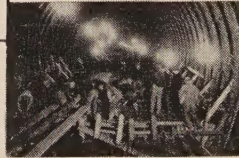
ROADWAY CONSTRUCTION MIDTOWN HUDSON TUNNEL
