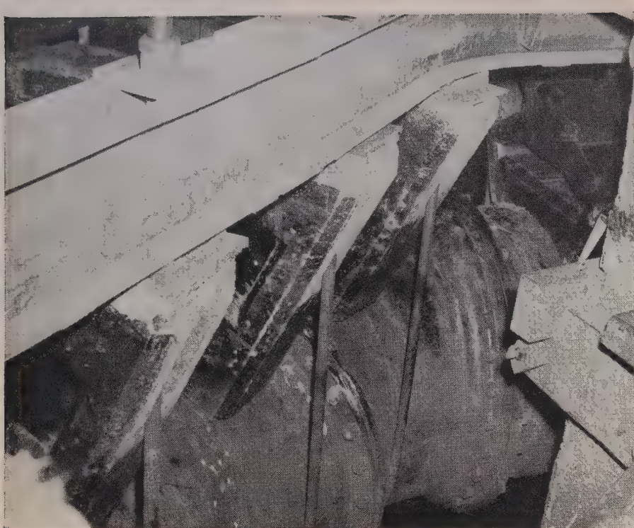
LONGITUDINAL CHANNELS were welded together with 4-in. clearance so that Monel rods could penetrate up to be bolted. Spacer blocks shown are of lightweight concrete.
