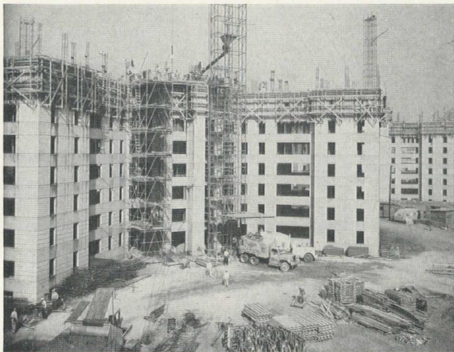
DURING concrete placing operations two transit-mix trucks unloaded concrete into a receiving hopper at the base of the double-section 190-ft. pipe hoisting tower. A two-way portable telephone system was used to control the delivery of the concrete to the upper floor. By using three complete floors of falsework, as shown, the concrete in the slab could reach its required strength before the shoring was needed on the third floor above to maintain the concrete placement schedule. Column steel is shown welded in place ready for the exterior forms to be raised the next working day after the concrete was placed.
