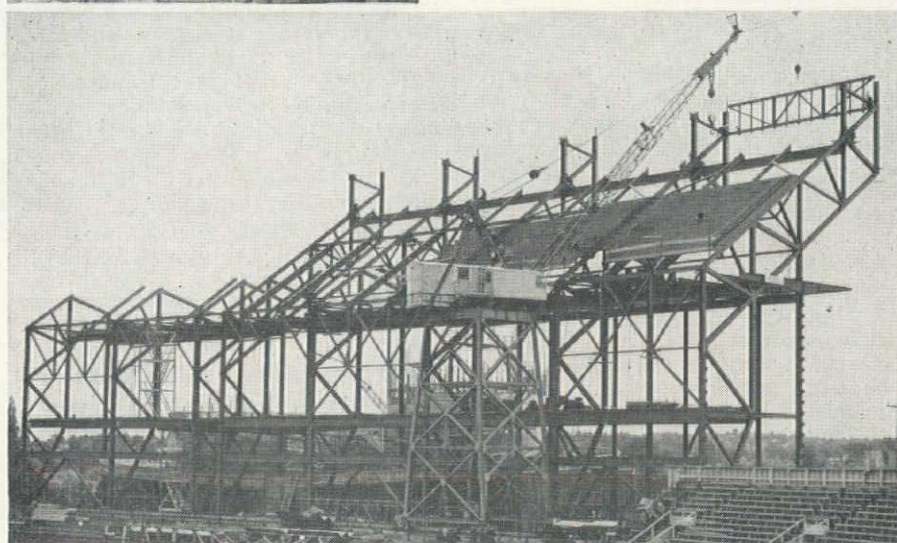
STEEL setting was carried out by crane traveling on curved track to follow line of stadium.
