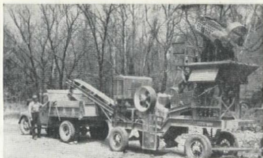
TS-TRAVELER —Screens finished pit run, crushes oversize. Blends and loads. Available in 916, 1016, 1020 or 1024 sizes with bronze or roller bearing jaw crushers.
