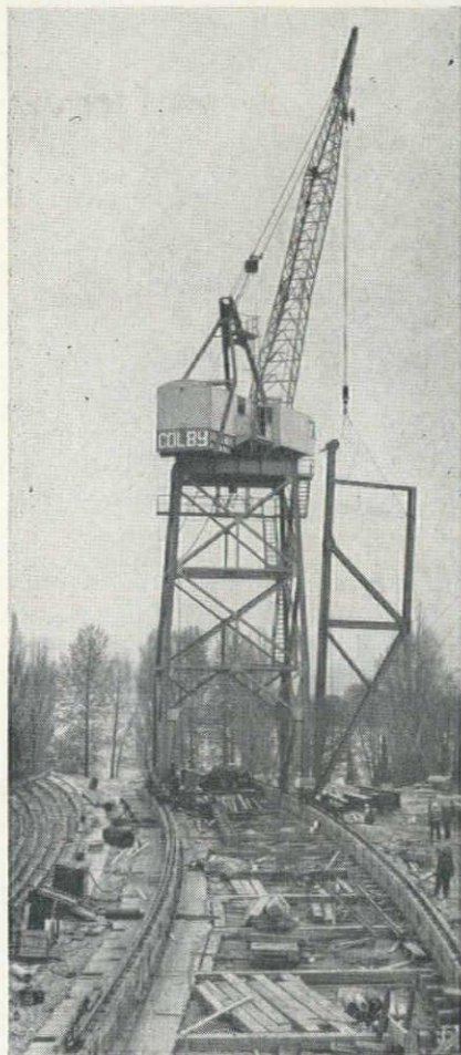
STEEL setting was carried out by crane traveling on curved track to follow line of stadium.
