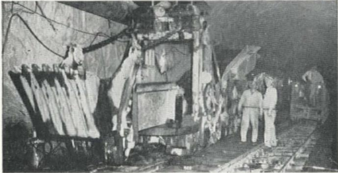
Huge scooper in tunnel of Bechtel-Morrison-Knudsen project at Big Creek Dam for Southern California Edison Company.
