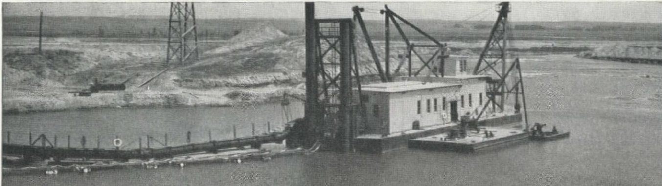
View above shows Bucyrus-Erie hydraulic dredge installation at work. In foreground on floats are electric cables which supply 6600-volt, 3-phase power to the 4000-hp pump motor, 500-hp cutter motor, and various other motors and control. Below is front-view close-up showing cutter in raised position.
