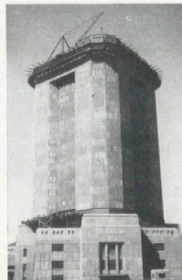
5. View showing the enclosure around the Fort Peck surge tanks nearing completion.
