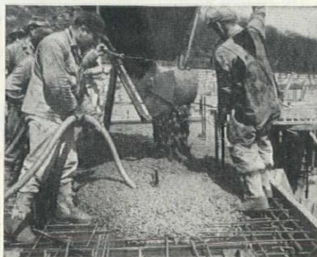
CP Hicycle Vibrator places concrete as fast as it is delivered.
