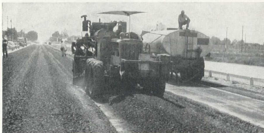
A GARDNER road-mixer worked the windrow, mixing the aggregates and applying the asphalt softener. Between 6 and 8 passes were made with the road-mixer.
