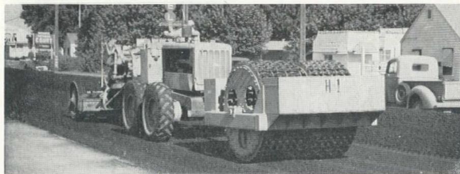
FURTHER passes with the Grid Roller over the newly-mixed material compacted the material in several courses to build the top surface up to its original thickness.
