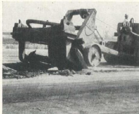
FIRST STEP in the test was ripping up the old pavement, accomplished here by a LeTourneau K-30 ripper pulled by a Caterpillar D-8 tractor.
