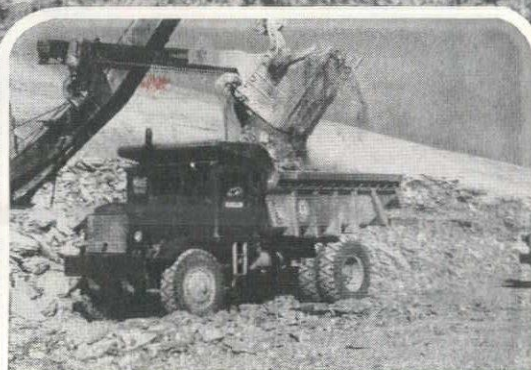
One of the "Eucs" owned by Latrobe Construction Company is loaded with rock and shale by a 2½ yd. shovel.
