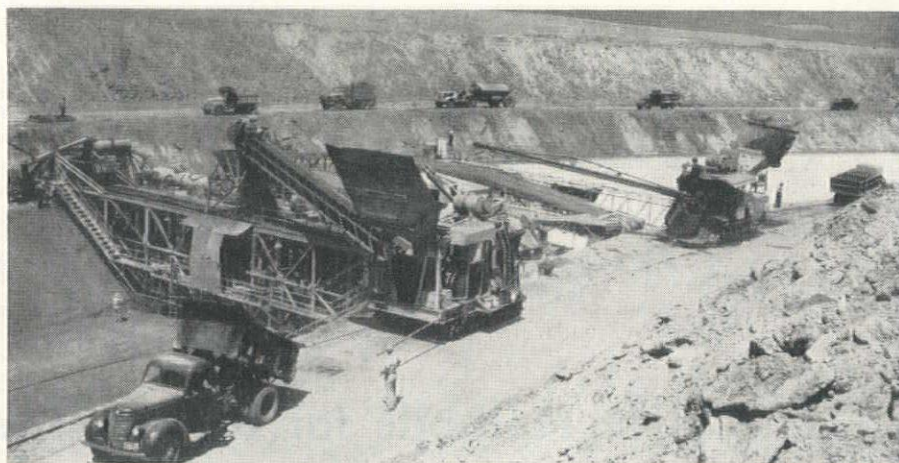
KEEPING FAST-MOVING slip-forms supplied with concrete is the major problem of both contractors. Above, trucks feed two Koehring Twinbatch mixers which deliver concrete to the Western Contracting slip-form. The firm is averaging about 1,600 cu. yd. of concrete lining per 8-hr. day. Morrison-Knudsen & Hasler is placing about 1,750 cu. yd. per 8-hr. day. The entire Delta-Mendota Canal is being lined at the rate of ½ mi. per day.
