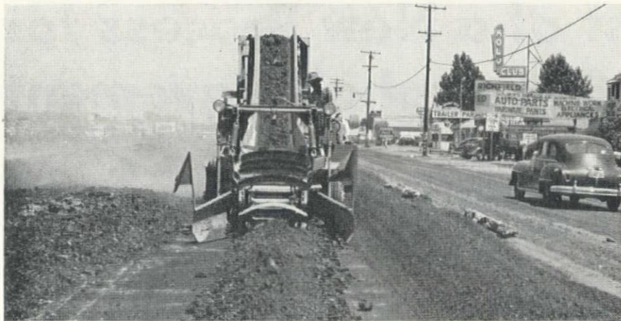
FOLLOWING the Grid Roller, an Athey loader and impact breaker made one pass to reduce lumps to the size of original aggregate and deposit the material in a windrow.
