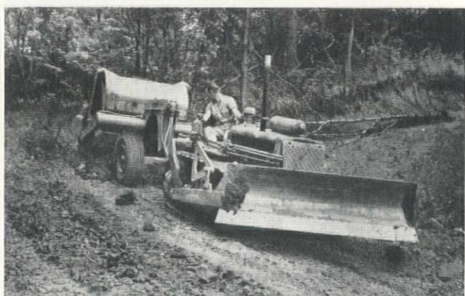
Scraper building a timber access road uses "U. S." braided Hydraulic Control hose. The weather-resistant, oil-resistant neoprene cover is bonded tightly to carcass. High hydrostatic strength is built into the hose through the use of high tensile braided steel wires.
