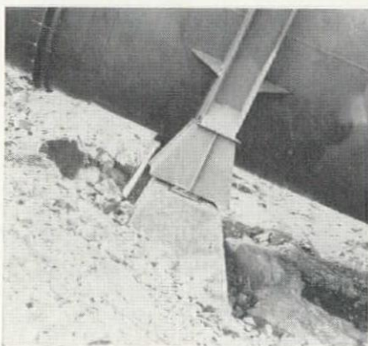
PENSTOCK is supported over its entire length by ring girders set on rockers which transmit load to concrete footings.
