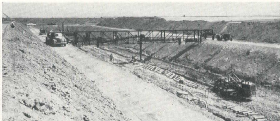
RUBBER-TIRED RIG was especially built for Morrison-Knudsen & Hasler to place gravel in drainage trenches. Dump trucks feed hopper at left and gravel is delivered by conveyor.
