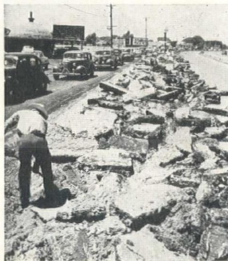
THE RIPPER left large chunks which were bulldozed to the side onto undisturbed pavement to be pulverized against the hard surface.
