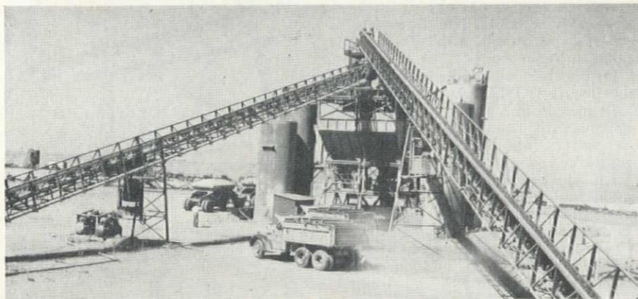
BOTH CONTRACTORS on current operations have high-capacity aggregate and batch plants. Above, the Morrison-Knudsen & Hasler plant. Sand and rock conveyors in foreground lead to batch plant, where all materials are obtained at one stop of the trucks. Stockpiles are in back of photographer. Below, air view of Western Contracting Corp. plant. Batch trucks make three stops—for rock, cement and sand, in that order.
