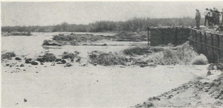
LOOKING UP the Gila River at one of the diversions. Weir crest is across center of picture; canal intake section is to right. Spillway apron is submerged 4 ft. under pool in foreground.
