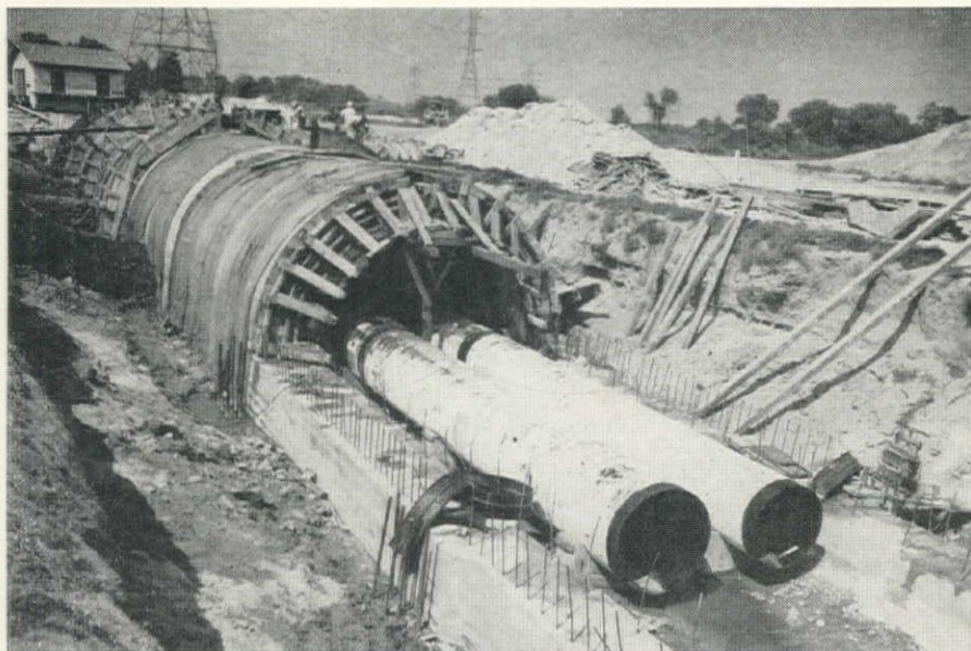
MUNICIPAL water lines, 30- and 36-in. steel pipes, are being relocated through the dam in an 11-ft. modified circular reinforced concrete conduit with walls 2 ft. thick.
