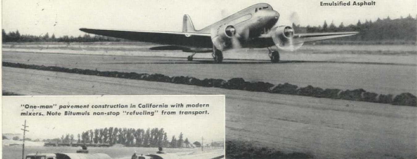
An Aleutian transport lands during runway construction. Bitumuls Sand-Mix although only partially cured — supports heavy loads.
