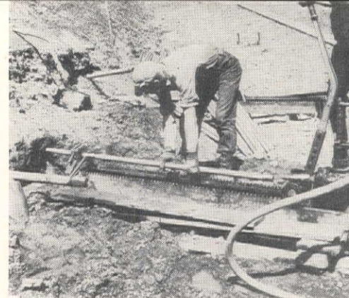
INSTALLATION of drains is accomplished by jacking perforated pipe into holes drilled into the unstable slope. "Hydrauger" equipment in use is especially designed for this work.
