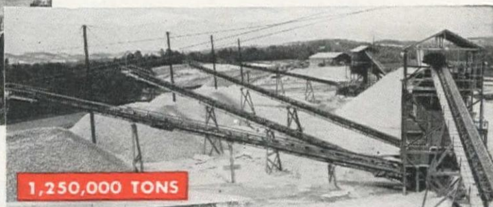
Buggs Island Dam, Va. This TelSmith crushing plant also produced the aggregate for Center Hill Dam.
