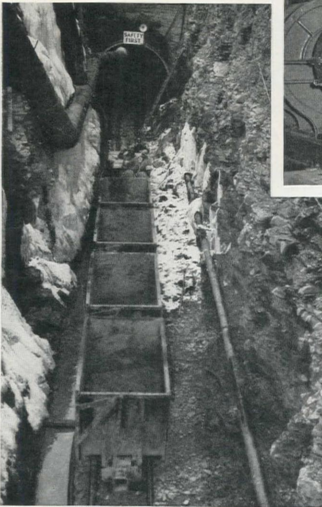
▲ Muck is efficiently hauled by 18 G-E battery and battery-trolley locomotives.
